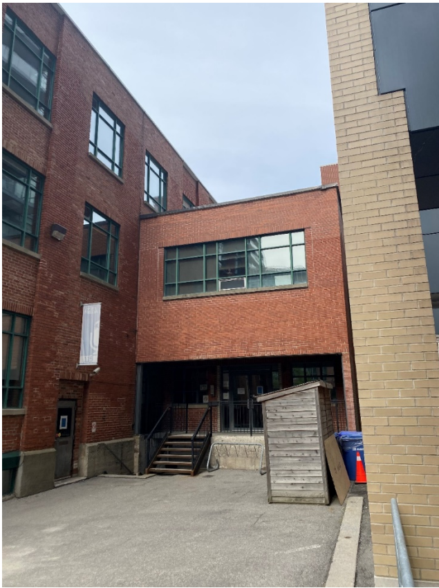
Figure 11: Current photo looking east and showing the 1950 one-storey addition to the Frankel Building complex. (Heritage Planning, 2021)
