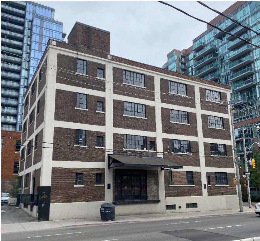
Figure 18: Current photo looking south and showing the north elevation of 125 George Street with its original loading bay and steel awning. (Heritage Planning, 2021)
