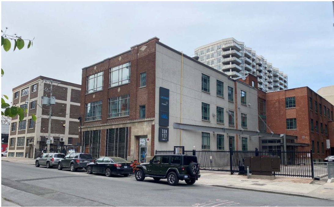
Figure 15: Current contextual photo looking northeast and showing both subject properties as well as the stucco overcladding on the south elevation at 109-117 George Street. (Heritage Planning, 2021)
