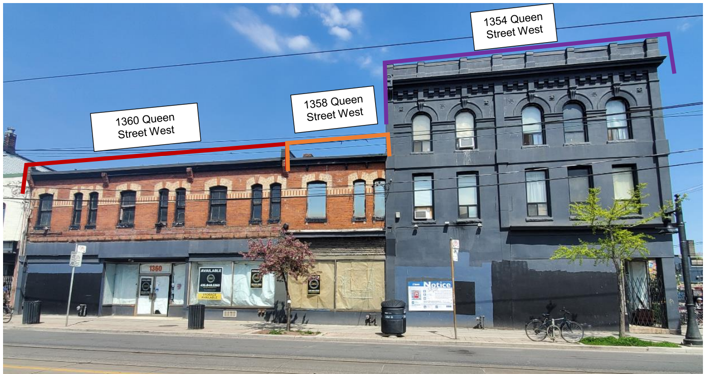
Principal (south) elevations of 1354, 1358, and 1360 Queen Street West (Heritage Planning, 2021)
