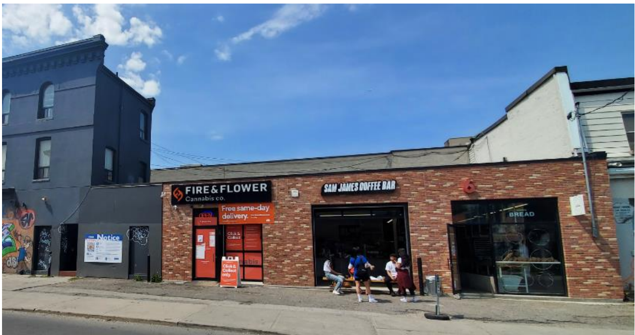
Figure 14. Detail of the one-storey rear addition at 1354 Queen Street West (Heritage Planning, 2021)
