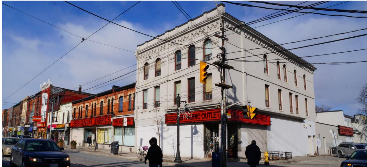
2014 photograph looking northwest at 1354, 1358, and 1360 Queen Street West (Jack Gibney)
