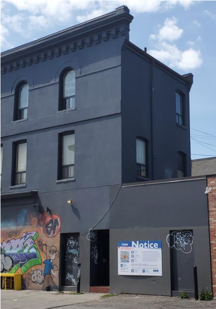
Figure 12. Rear (north) elevation of 1354 Queen Street West (Heritage Planning, 2021)
