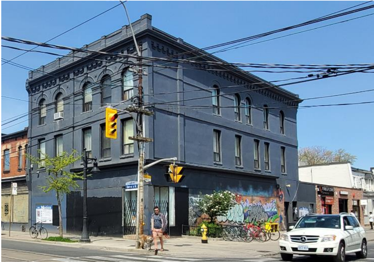
Figure 9. View of the southeast corner of 1354 Queen Street West (Heritage Planning, 2021)
