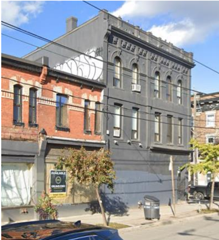
Figure 13. Detail of the chimney in the side (west) elevation of 1354 Queen Street West (Google Streetview, 2020)
