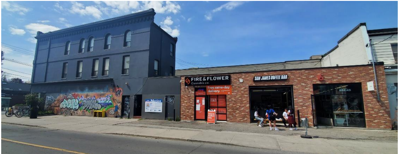
Detail of the side (east) elevation of 1354 Queen Street West with the rear one-storey addition (right) (Heritage Planning, 2021)
