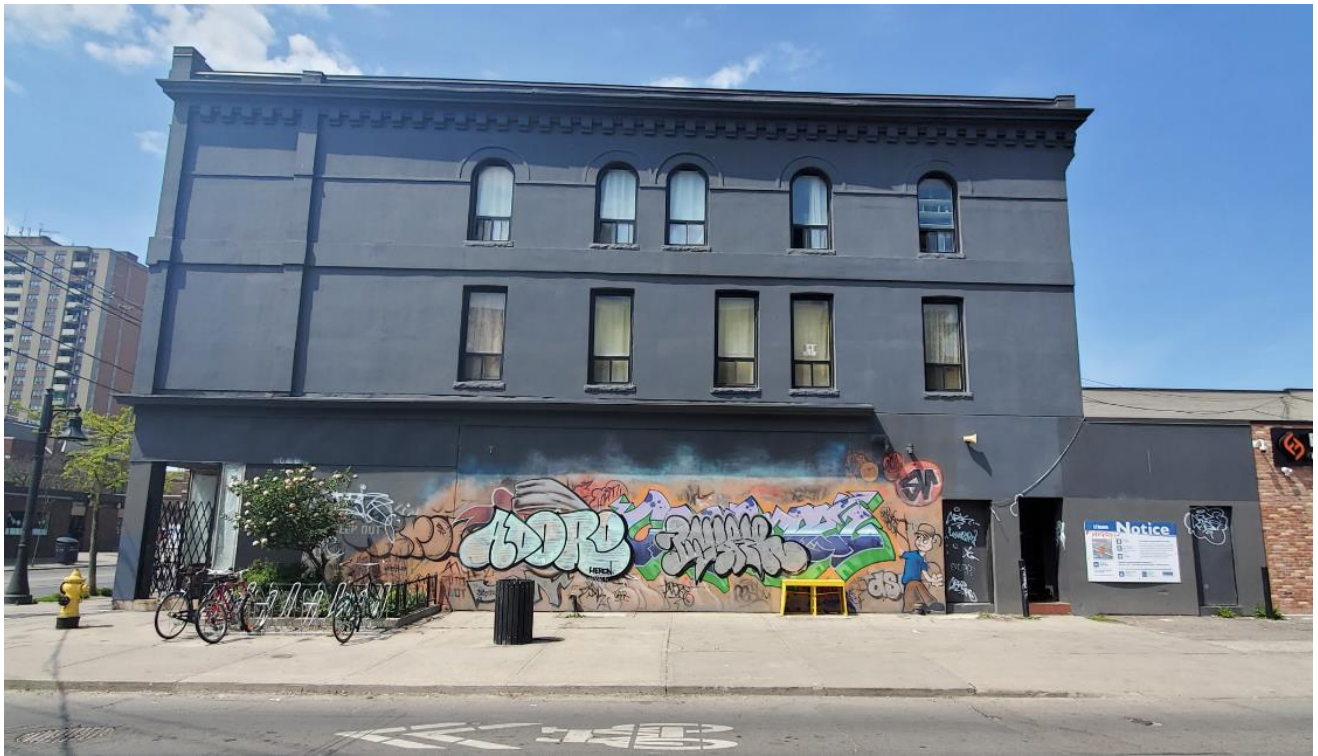
Detail of the side (east) elevation of 1354 Queen Street West (Heritage Planning, 2021)
