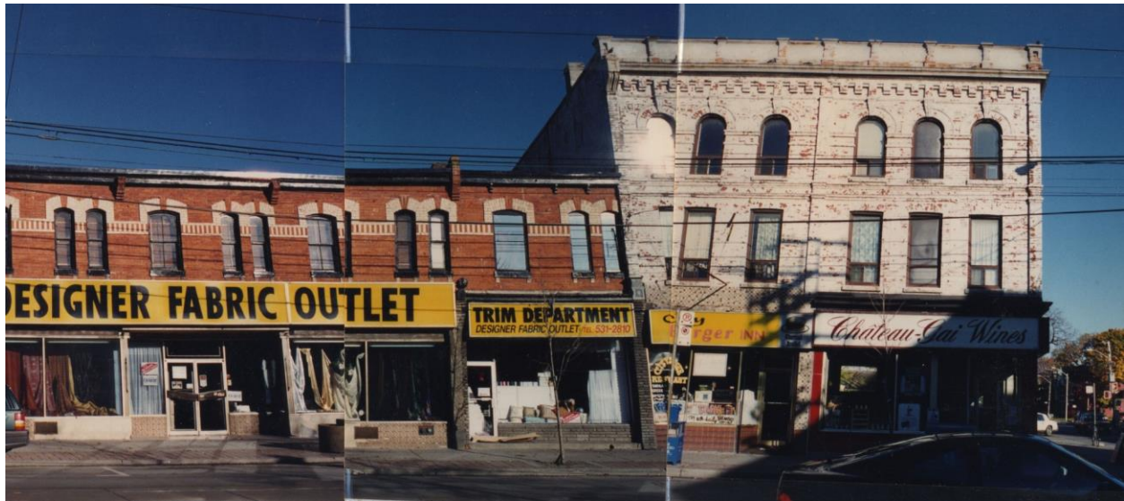
1996 photograph of the principal (south) elevations of 1354, 1358, and 1360 Queen Street West (Jack Gibney)
