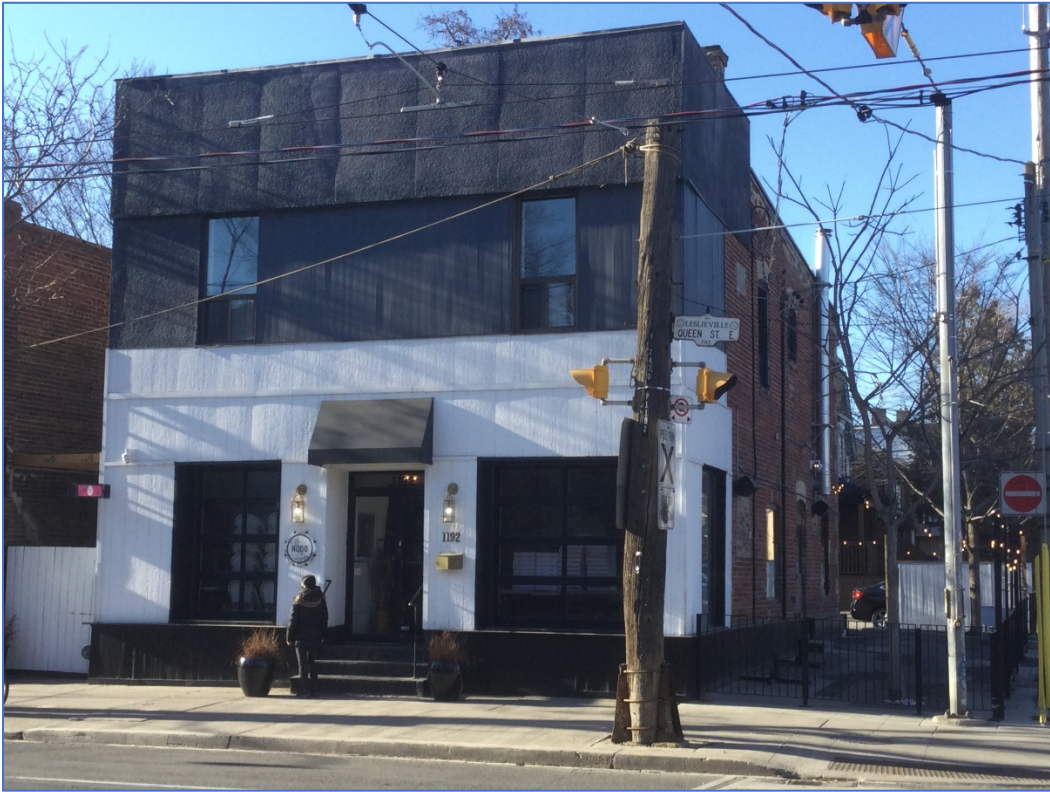
1192 Queen Street East
