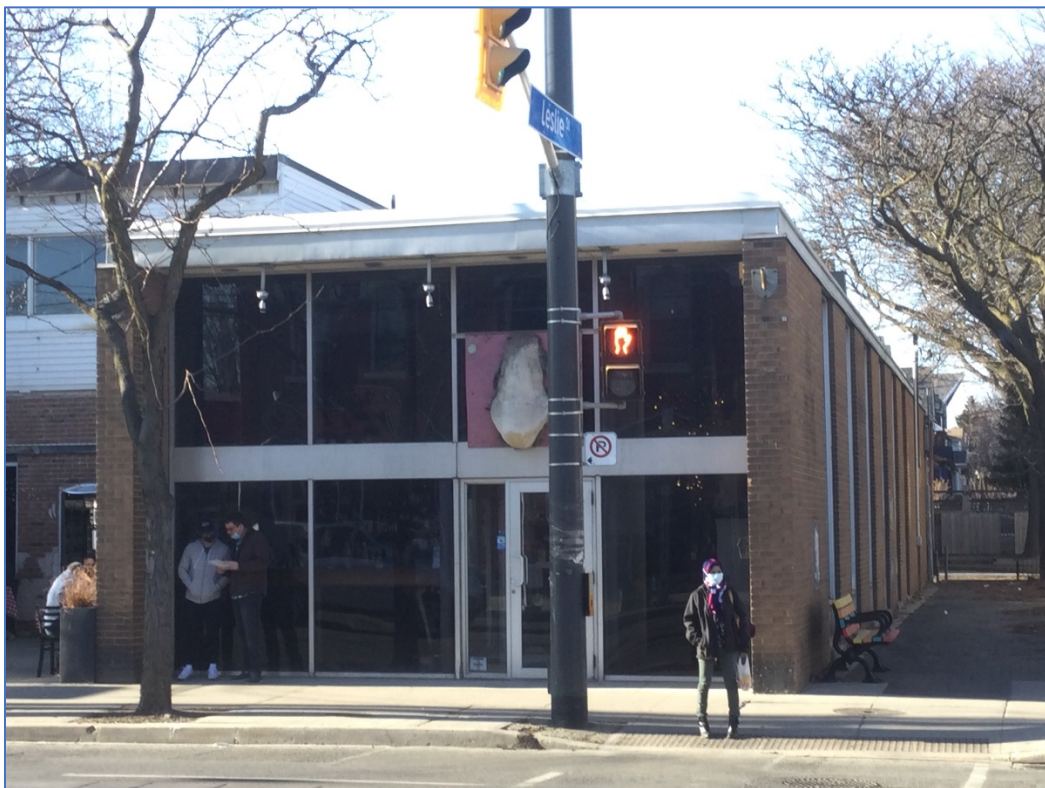
1220 Queen Street East
