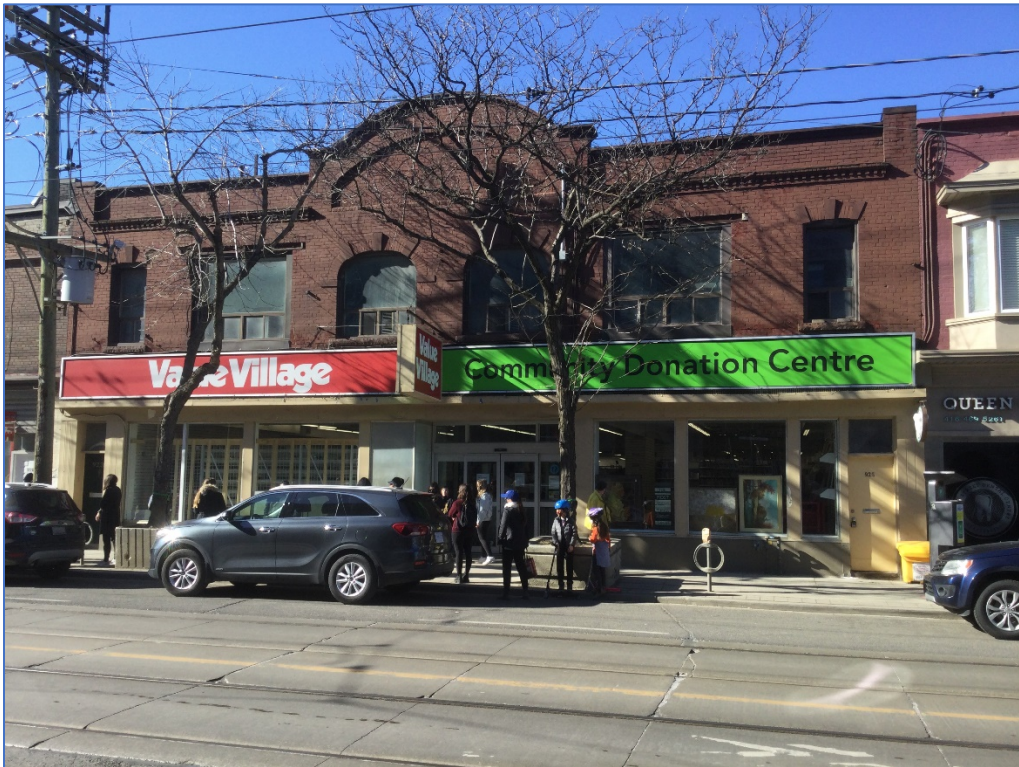
924-926 Queen Street East
