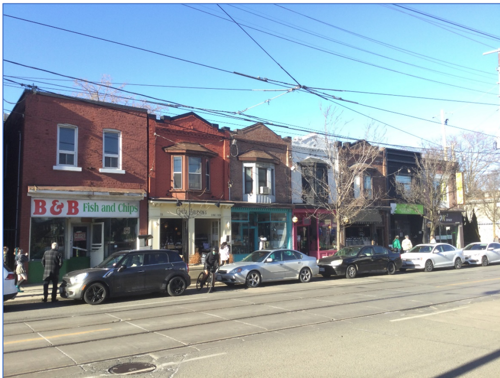
1118-1124 Queen Street East
