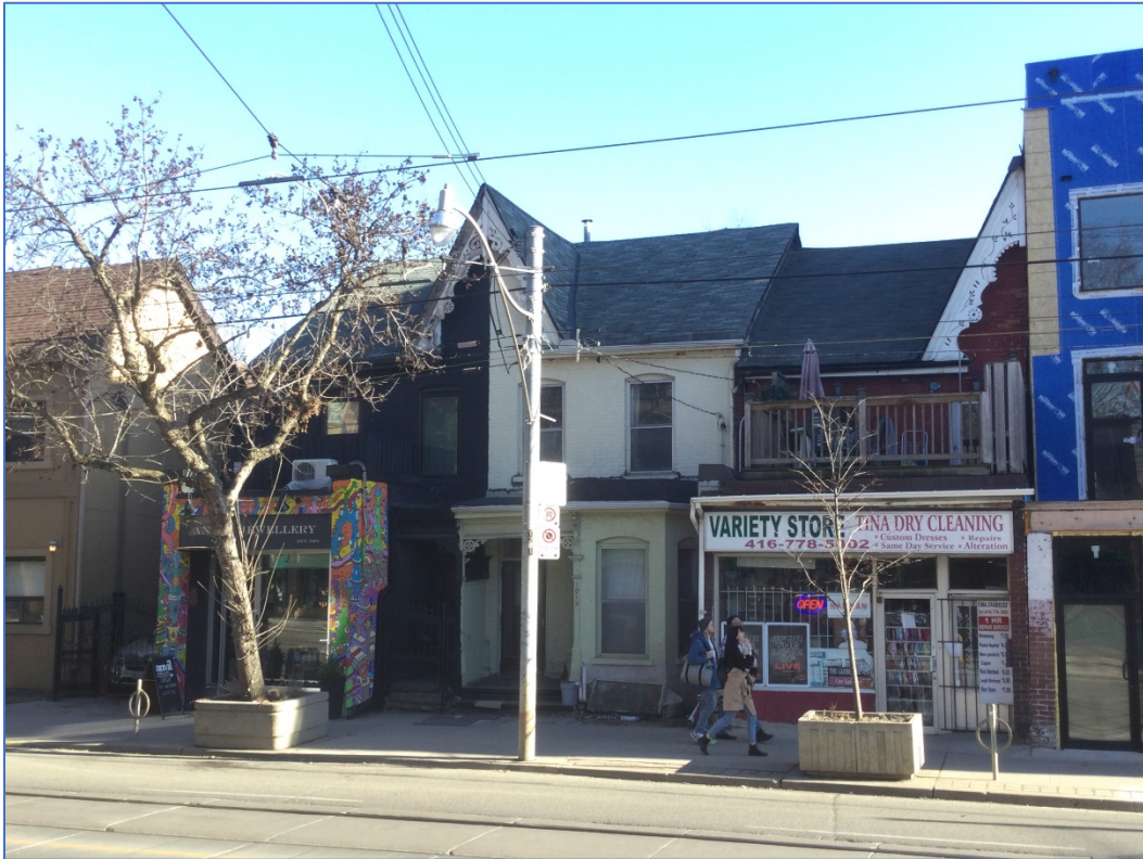
1011-1015 Queen Street East
