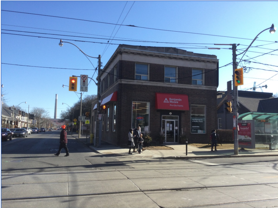
943 Queen Street East
