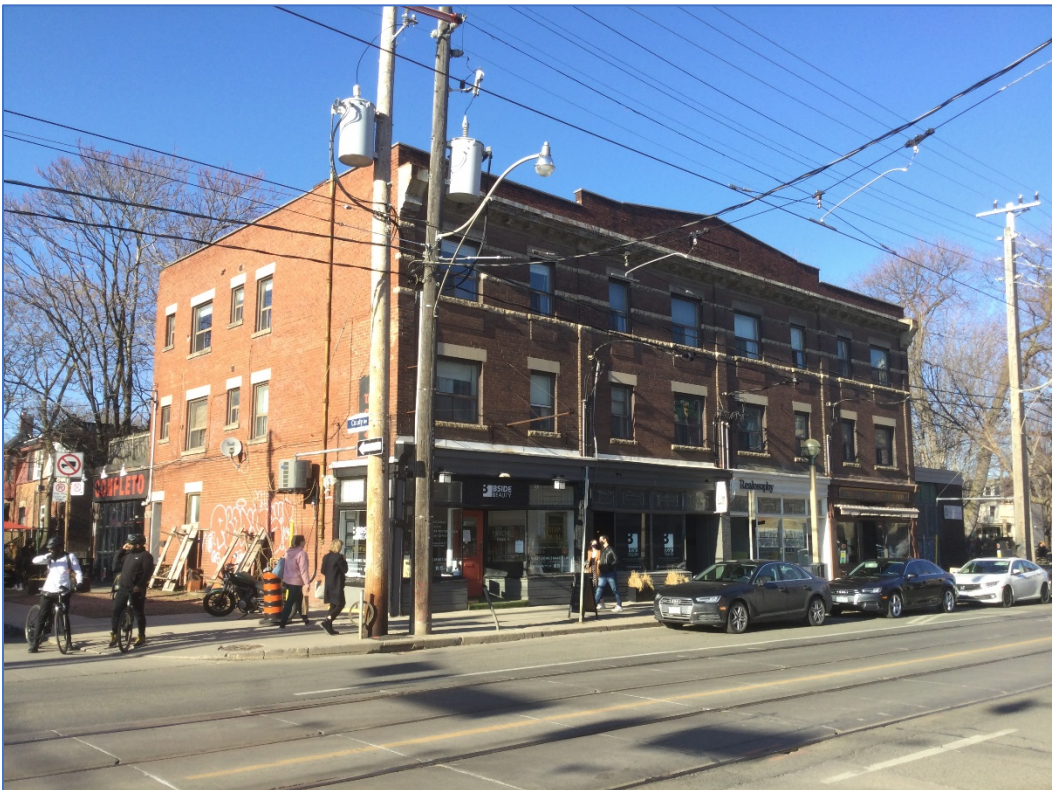
1148-1154 Queen Street East
