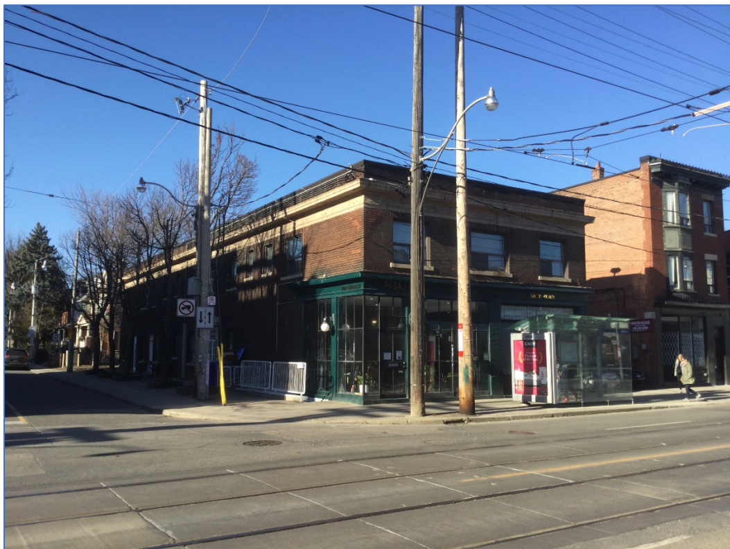
1100 Queen Street East
