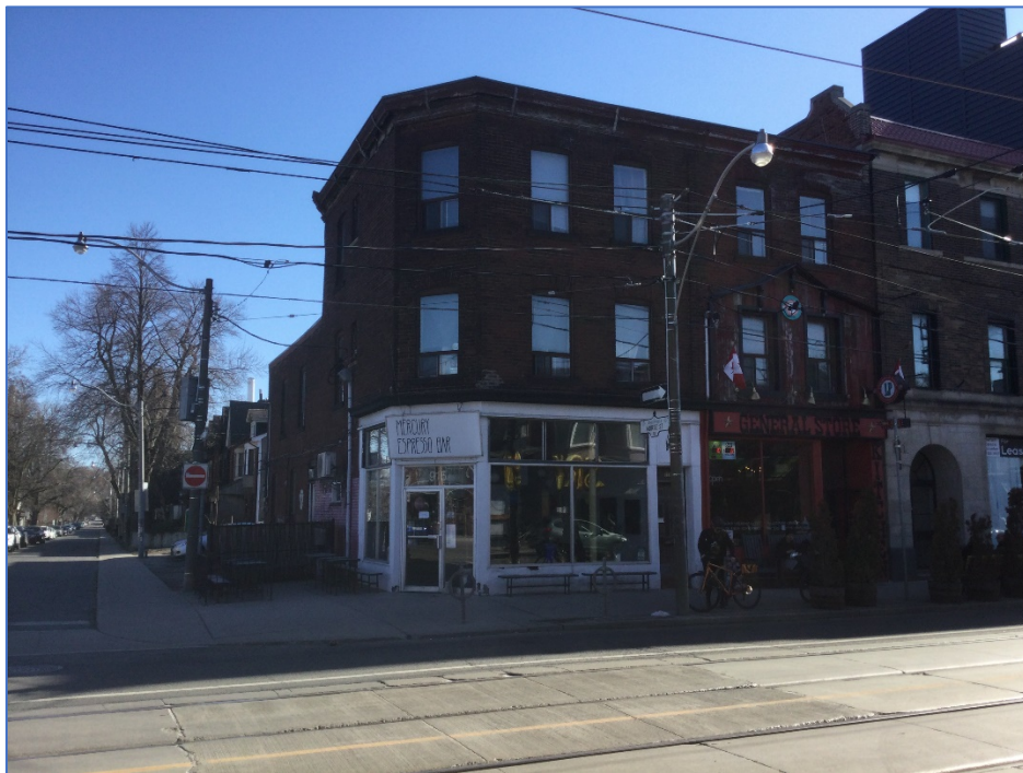
913-915 Queen Street East
