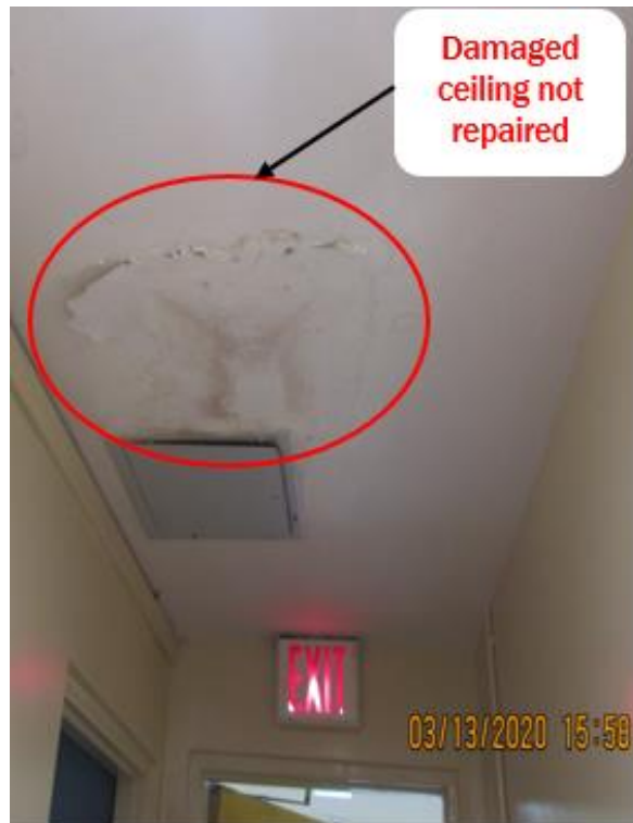
Photograph 6: Damaged hallway ceiling was not repaired
