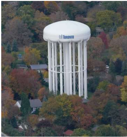
Toronto Water SCADA System Security
