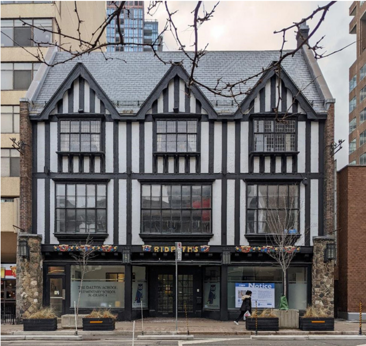
East (principal) elevation of 906 Yonge Street (Heritage Planning, 2021)
