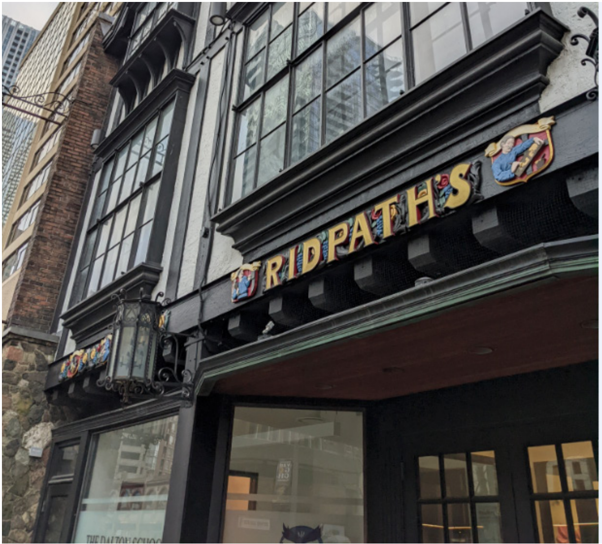
22. Detailed view of ground floor attributes on 906 Yonge Street's east elevation, including the timber post and beam structure, the horizontal beam above the storefront supported by timber brackets, and copper soffit details in each bay. (Heritage Planning, 2021)
