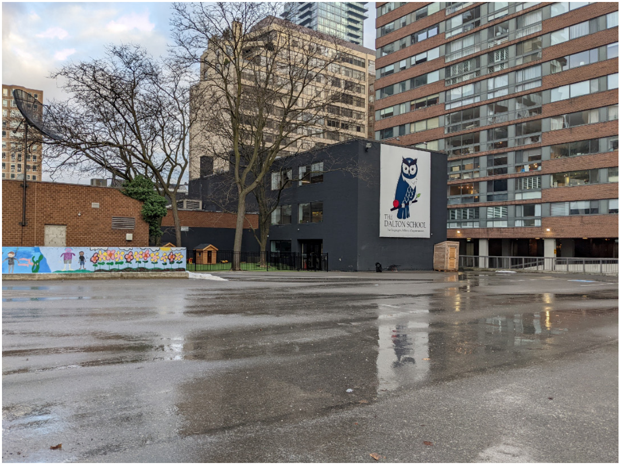
25. View of the north (side) and west (rear) elevations of the rear portion of 906 Yonge Street, visible from McMurrich Street (Heritage Planning, 2021)
