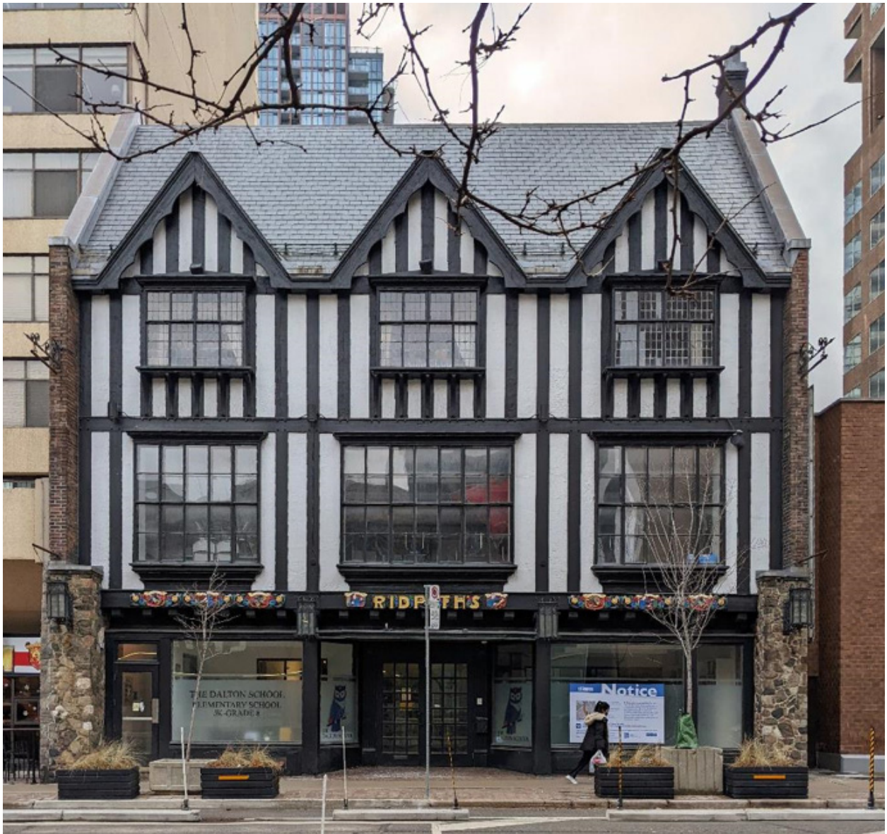
19. View of the east (principal) elevation of 906 Yonge Street (Heritage Planning, 2021)
