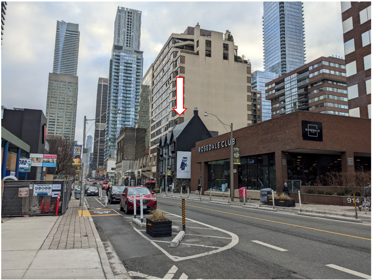
28. Context view of 906 Yonge Street, looking southwest from Yonge Street (Heritage Planning, 2021)
