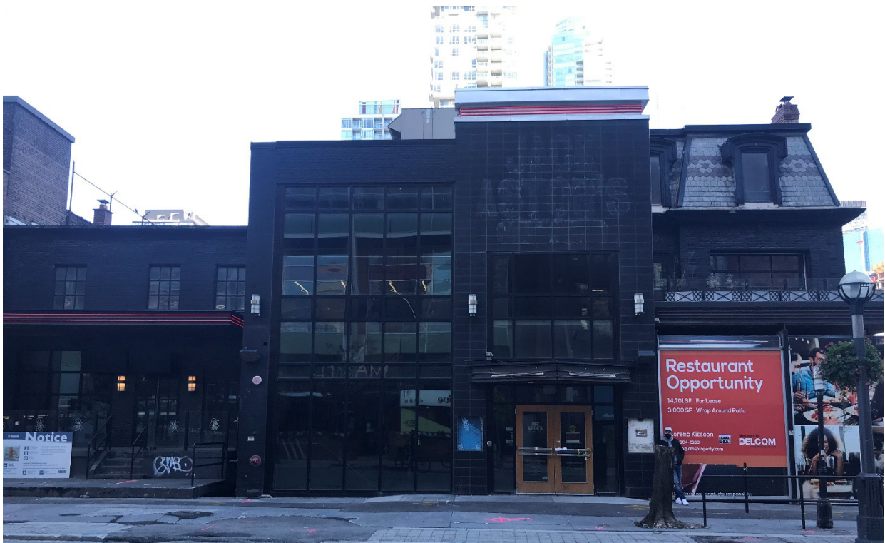
12. Current photograph showing the principal (west) elevations of the consolidated buildings comprising 133 John Street. At far left is the truncated form of the formerly three-storey rowhouse at then 137 John (Heritage Planning, 2021)
