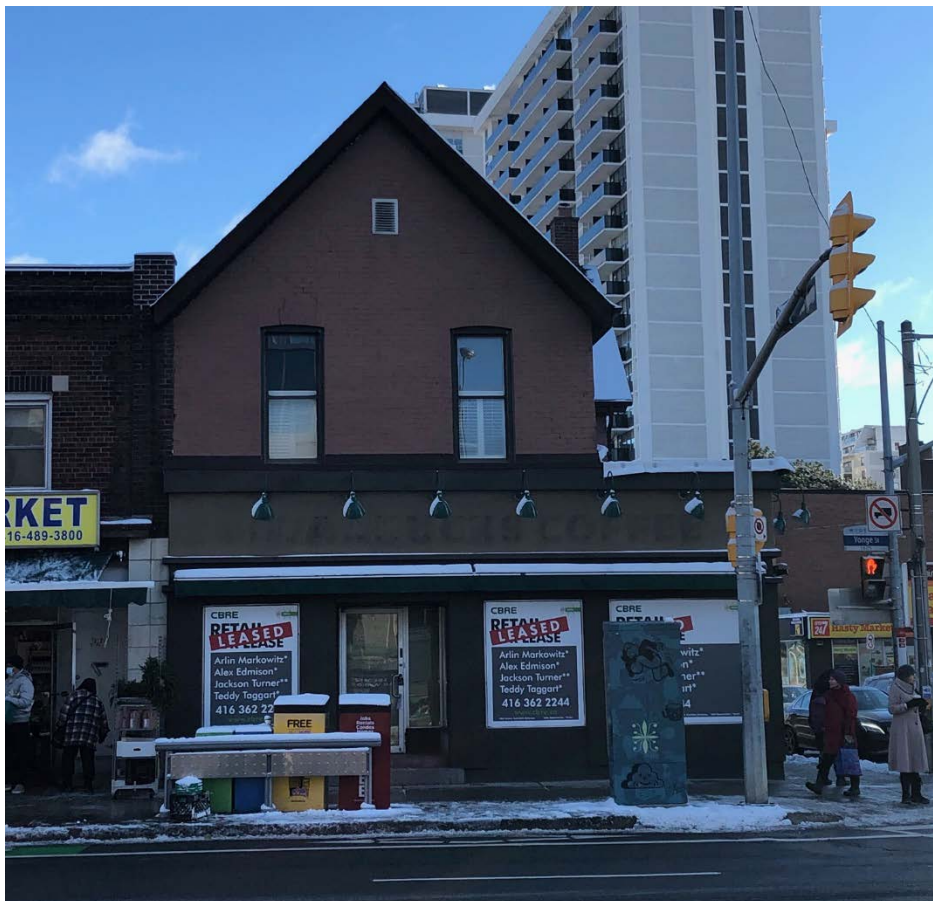
12. Current photograph looking east, showing the west elevation of the building at 1909 Yonge Street. (Heritage Planning, 2021)
