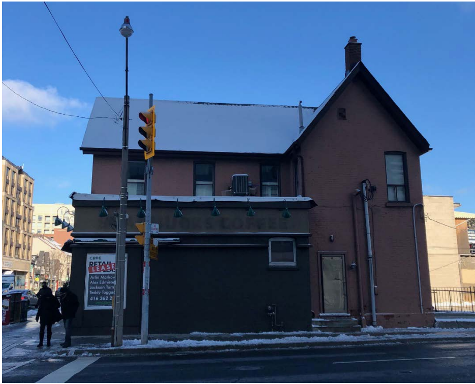
13. Current photograph looking north, showing the south elevation of the building at 1909 Yonge Street. (Heritage Planning, 2021)
