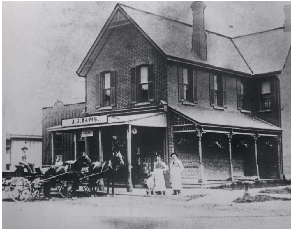
4. c. 1900 photograph of the J. J. Davis General Store and Post Office at the northeast corner of Yonge Street and Davisville Avenue. Note that at this time, the building retained its original L-shaped footprint and wooden verandahs along its west and south elevations. (TPL)
