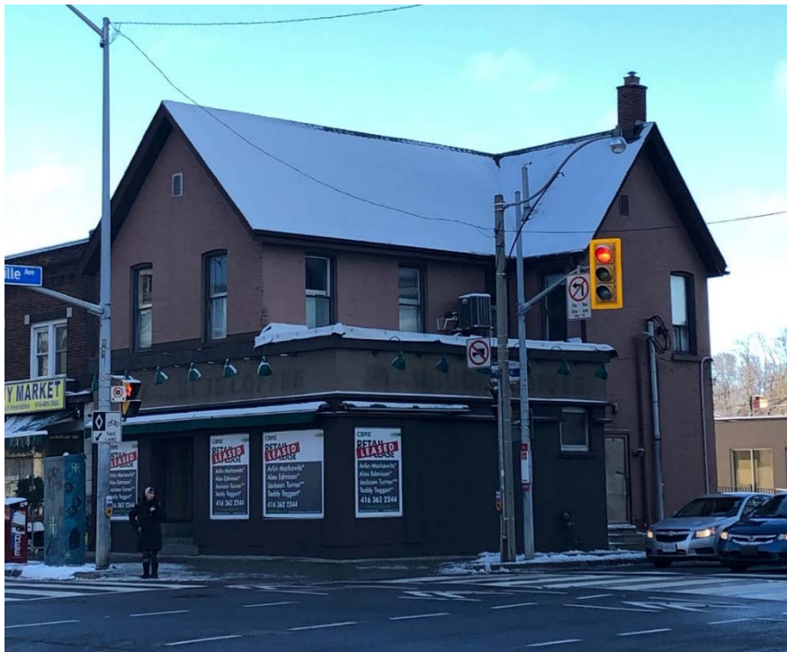
West and south elevations of 1909 Yonge Street at the northeast corner of Yonge Street and Davisville Avenue (Heritage Planning, 2021)
