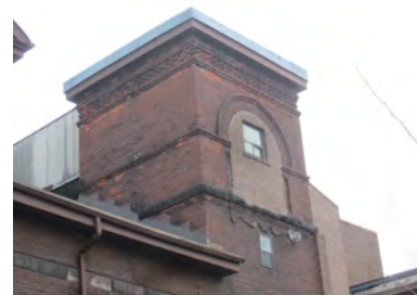
Window alterations on the south facade of the tower (ERA, 2015).
