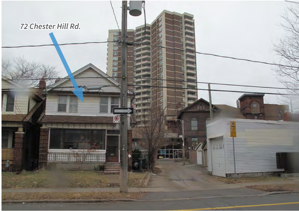
View looking north toward the site from Chester Hill Road; 72 Chester Hill Road in the foreground forming part of the subject site (ERA, 2018).
