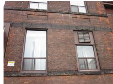
Typical aluminium framed windows on the south elevation (ERA, 2015).
