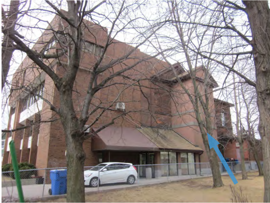
North elevation; 1996 elevator addition annotated with an arrow (ERA, 2018).
