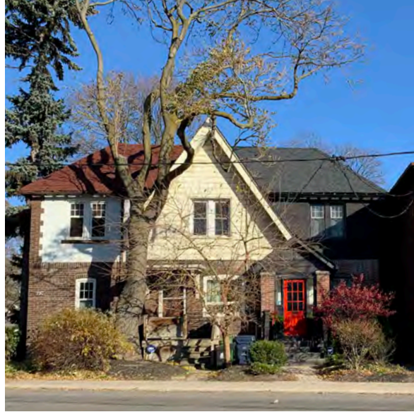
927-931 Broadview Avenue front (west) elevation (DiamondCorp, 2020).
