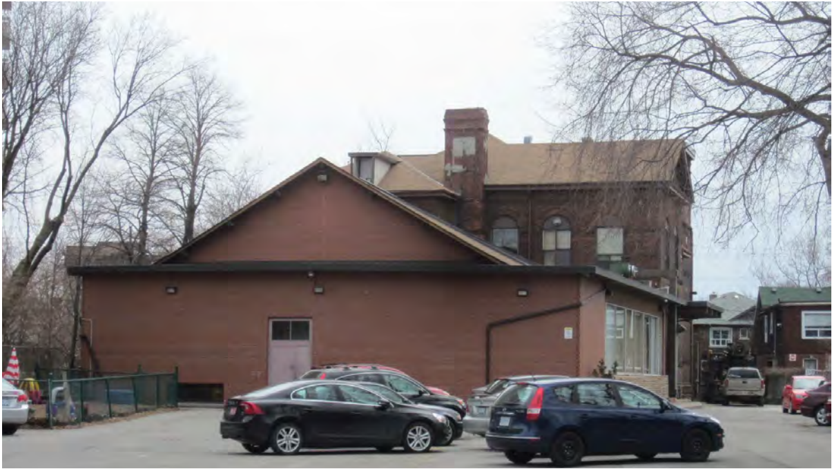
Rear (west) elevation (ERA, 2015).
