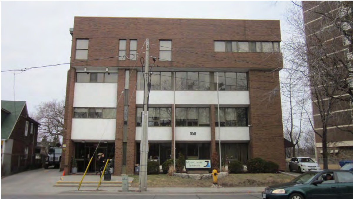
Main (east) elevation (ERA, 2015).
