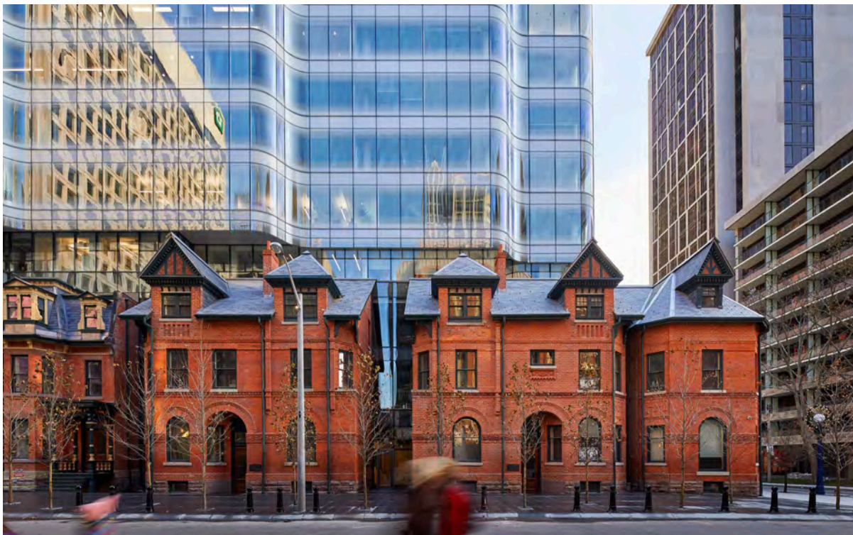
At 7 St. Thomas, the project involved partial building retention with reinstatement and reconstruction (HPA).
