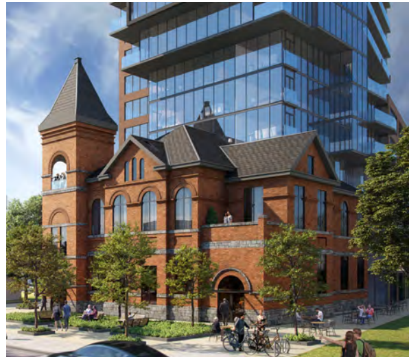
Rendering of restored and rehabilitated 1891 building with new canopies above two restored entrances (G+C, 2021)
