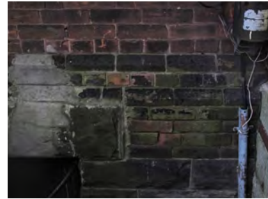
Soiling and biological growth on north facade (ERA, 2018).
