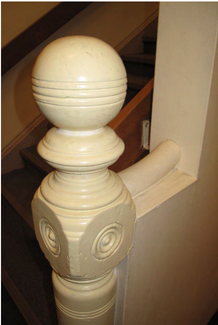
Newel post and handrail from former Chester Public School; (ERA, 2018).
