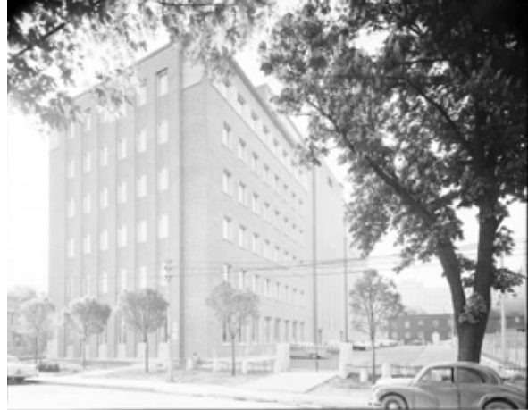
South and east facades of the building c. 1957 (Canadian Architectural Archives, University of Calgary).
