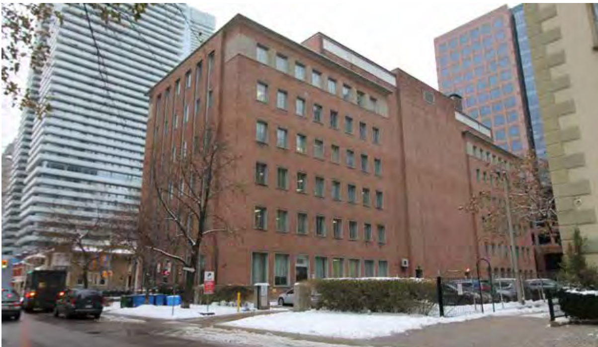
East and south elevation of the Site viewed from Charles Street (ERA, 2019).
