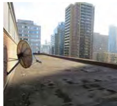
Roof condition (ERA, 2015).
