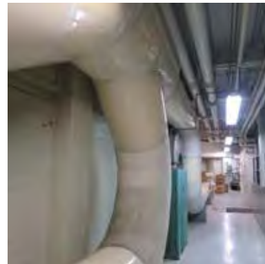
Mechanical penthouse (ERA, 2015).
