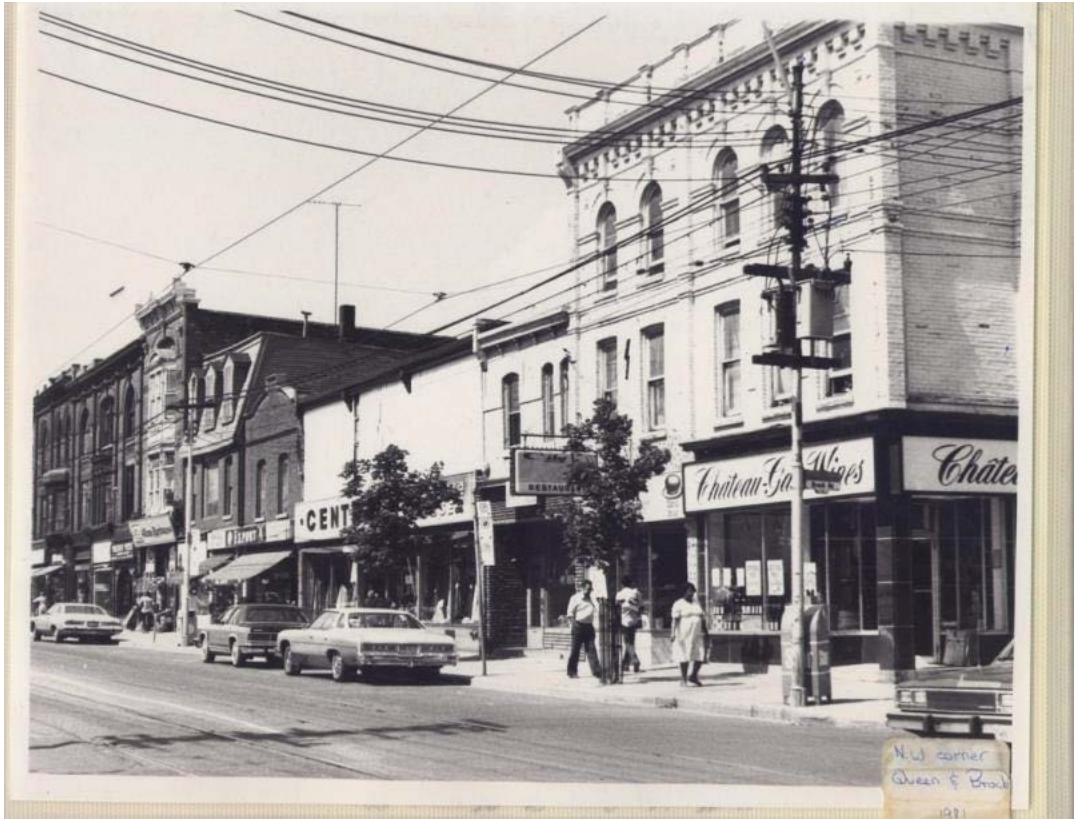
1981 Photo of the site.
