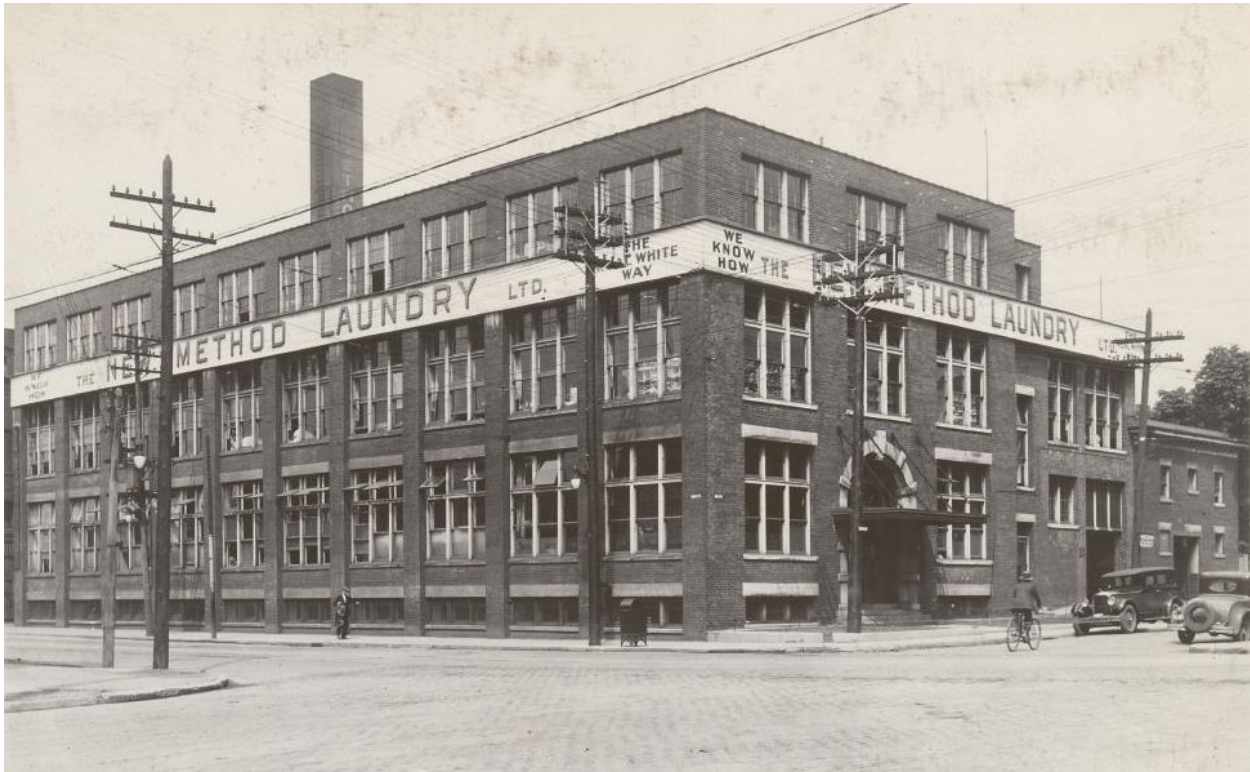
Image 14. Archival photo (1929-30) of the New Method Laundry building with its 1923-built third-storey addition and modified cornice (replaced by signage). City of Toronto Archives, Fonds 1488, Series 1230, Item 3575.
