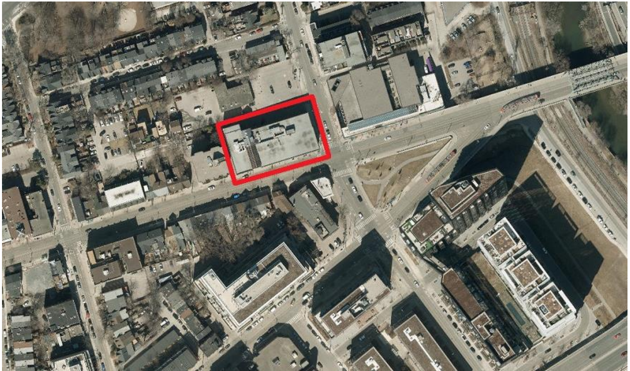
Image 6. Aerial Photo (2021) showing 544 and 550 Queen Street East (indicated in red).
