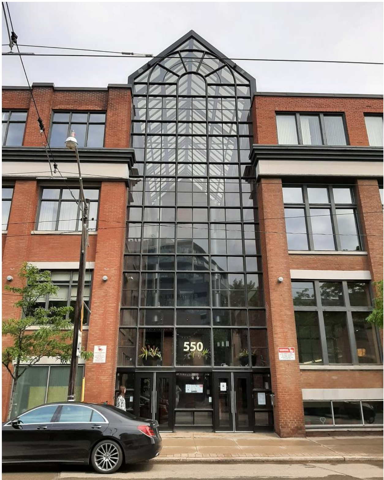
Image 19. Atrium connecting the former National Electric Heating and New Method Laundry buildings which comprise 544 and 550 Queen Street East. Heritage Planning, 2022.
