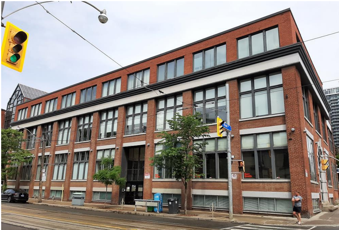
Image 20. Front elevation of the former New Method Laundry building (today part of 544 and 550 Queen Street East). Heritage Planning, 2022.
