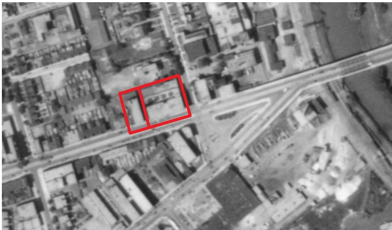
Image 4. Aerial Photo (1939) showing 544-548 Queen Street East and 2 River Street (550-554 Queen Street East) today listed as 550 Queen Street East (indicated in red).
