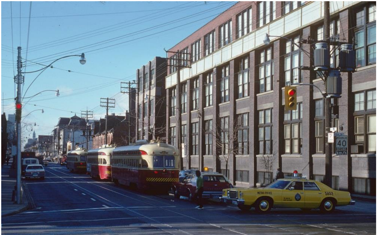
Image 15. Archival Photo (1981) of the New Method Laundry and National Electric Heating prior to their conversion into 544 and 550 Queen Street East. City of Toronto Archives, Fonds 1526, File 75, Item 41.
