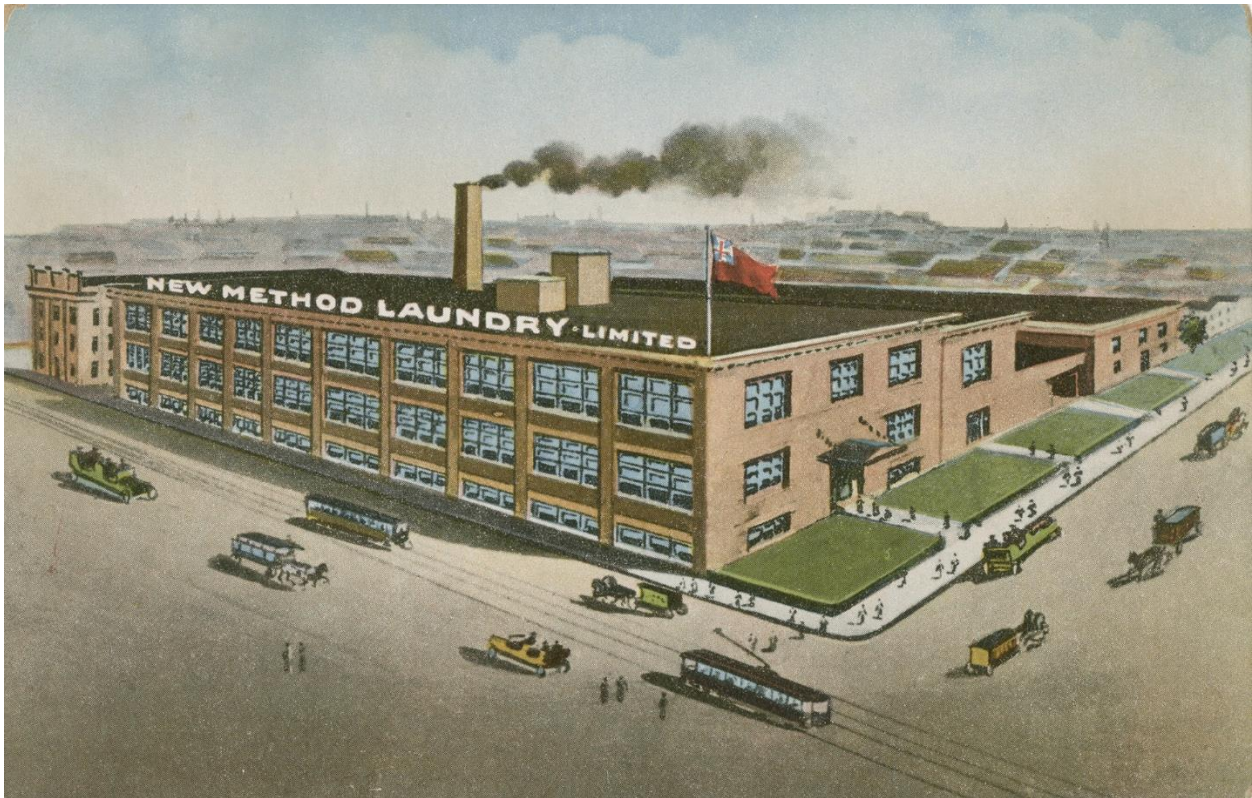
Image 11. Postcard (1910) featuring New Method Laundry Co. Ltd. building at 2 River Street (550 Queen Street East) in its original two-storey configuration with rear addition and stables and the adjacent National Electric Heating Co. Ltd. building (with parapet/false front) at 544-548 Queen Street East. TPL - Baldwin Collection.
