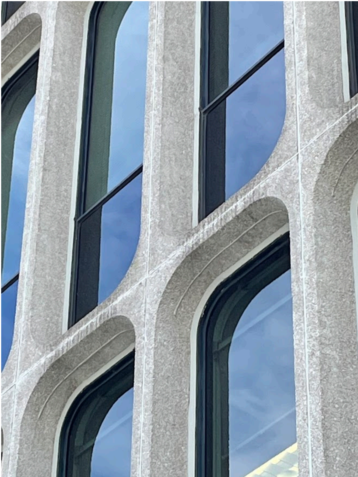
Image 17. Current photograph showing detail of the deep profile of the precast concrete panels (Heritage Planning, 2022)
