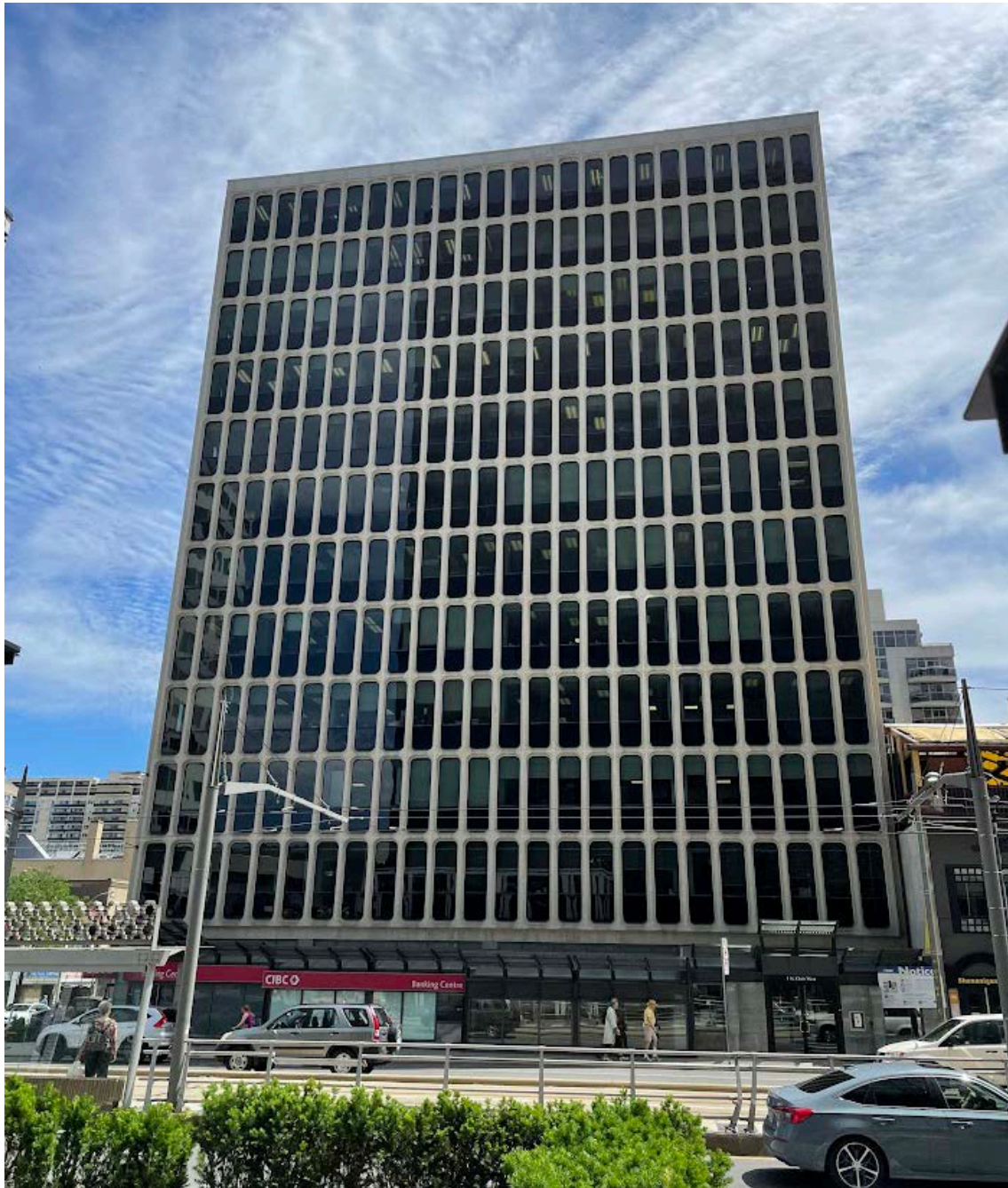
Current photograph showing the north elevation of the property at 1 St. Clair Avenue West (Heritage Planning, 2022)
