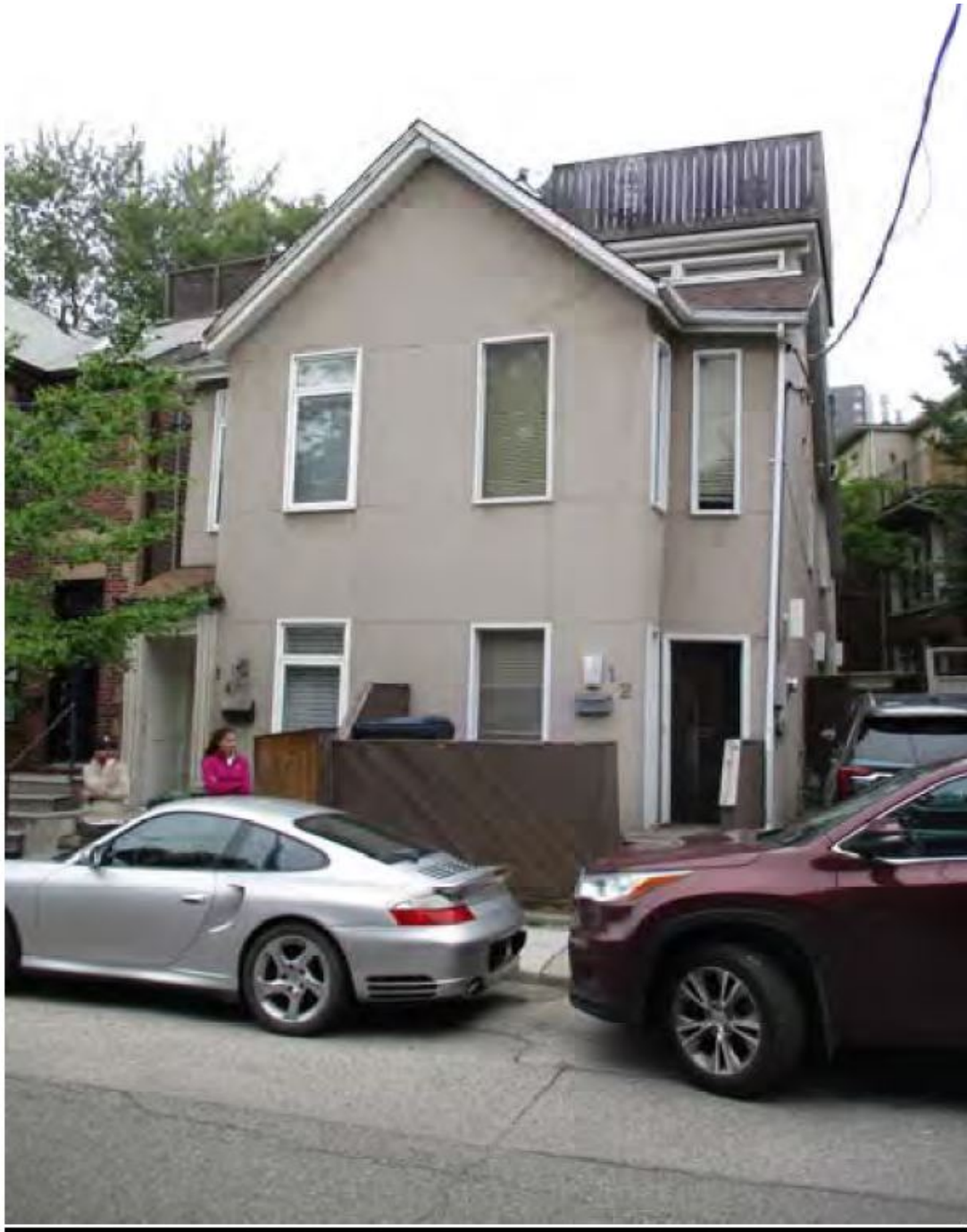
Photograph of the south (principle) façade of the existing building at 12-14 Bishop Street.
