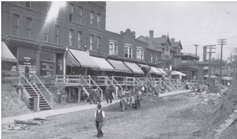
Image 9. 1914-1916 Archival photo showing the excavated basement level and temporary raised stairs and platforms erected to access the original storefronts during the street regrading (CTA)
