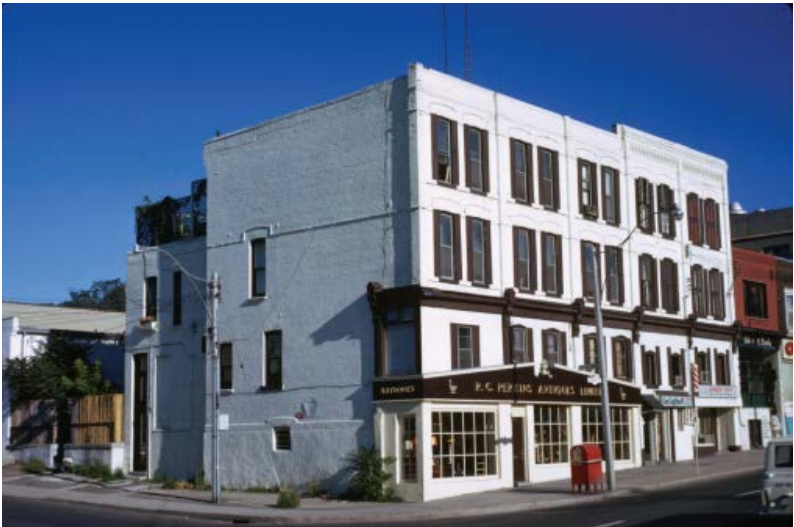
Image 16. 1973 Archival photo showing the commercial block at 1196-1204 Yonge with its brick cladding painted and amalgamation of the three southern storefronts into a single retail space. (CTA)
