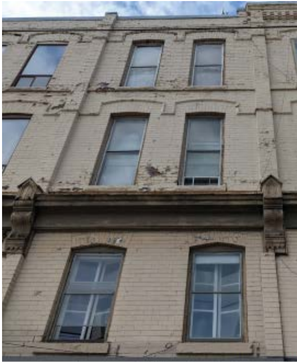
Image 20. 2021 Image showing the brick detailing in the third and fourth storeys, the 1920s punched windows at the second storey level and the wooden cornice with decorative "birdhouse" capitals at each bay, signalling the location of the ceiling of the original storefronts.
