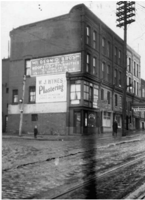
Image 15. 1935 Archival photo indicating that by this time all five bays of the commercial block had shifted the original storefronts to the basement level and replaced the new second storey space with residential units. (CTA)
