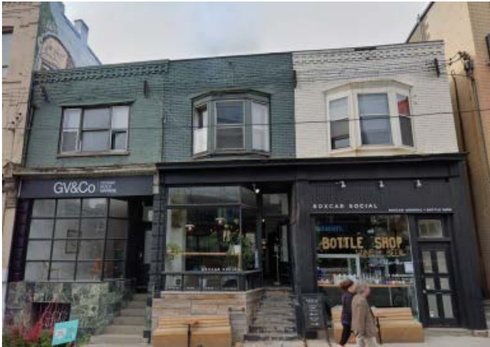
Image 21. 2021 Image showing the east elevations of the commercial main street row at 1206-1210 with their bay windows and decorative brick detailing in the upper storey and post-1914 raised entry stairs (external at 1206-1208 and internal at 1210).
