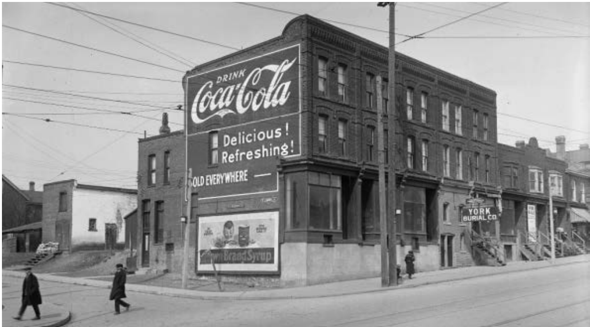
Image 11. 1920 Archival photo showing the shift of storefront down to the new street level at 1202 Yonge for York Burial. (CTA)
