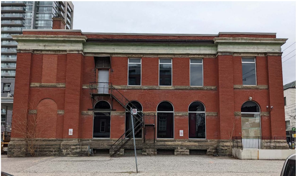
Figure 18. Side (east) elevation of 1117 Queen Street West, showing the fire escape added in 1960. (Heritage Planning, 2022)
