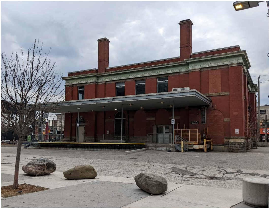
Figure 17. Rear (south) elevation of 1117 Queen Street West. (Heritage Planning, 2022)
