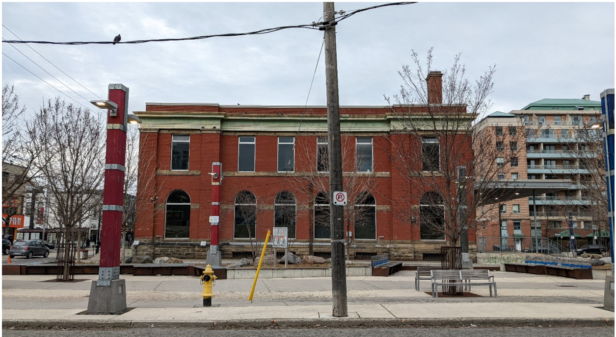
Figure 19. Side (west) elevation of 1117 Queen Street West. (Heritage Planning, 2022)
