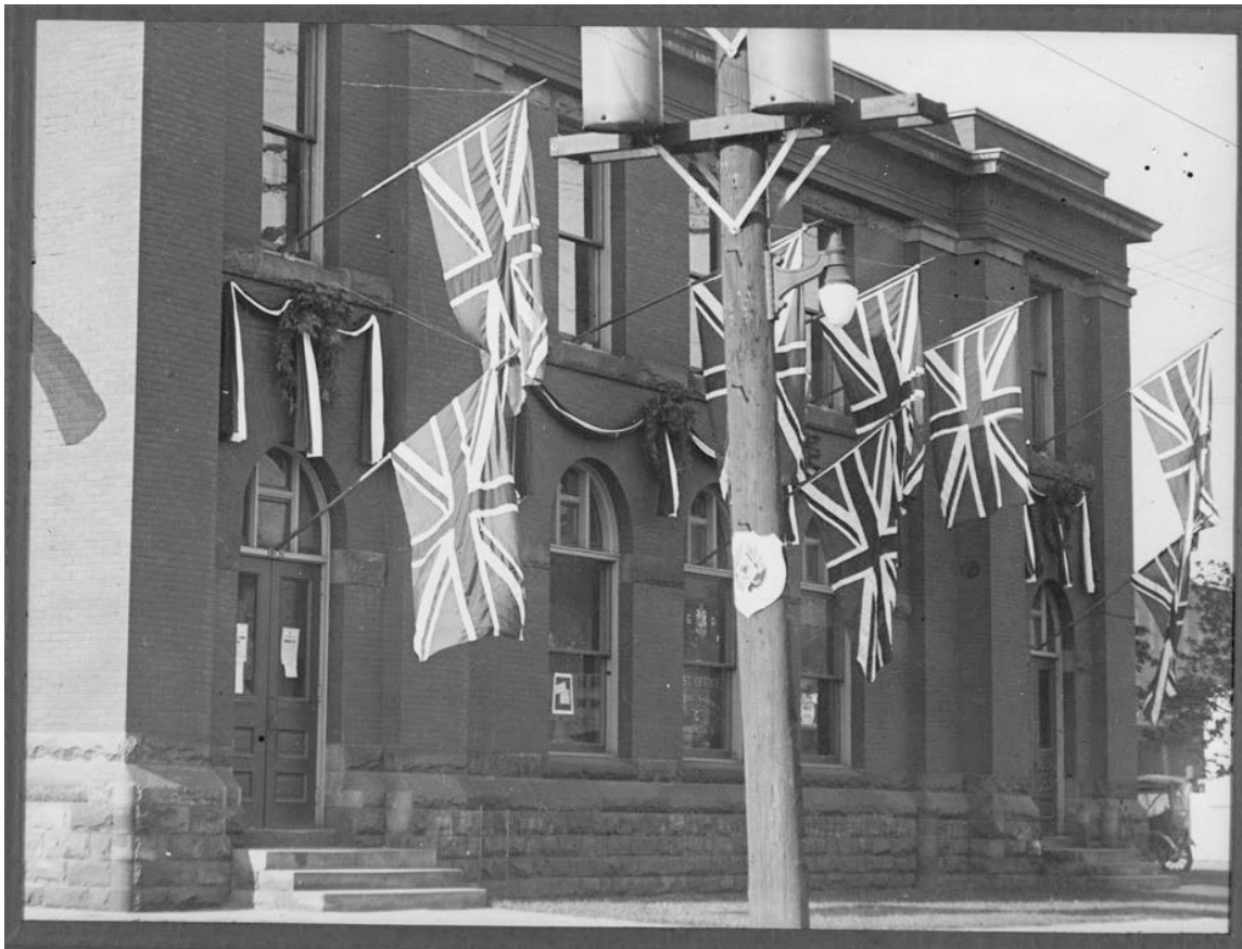
Figure 13. 1927 Photo of north elevation of 1117 Queen Street West. Post offices across Ontario were decorated for the "Diamond Jubilee of Confederation". (Library and Archives Canada)
