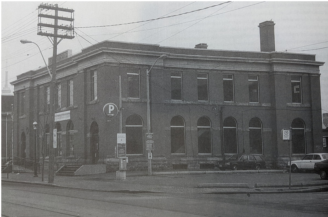
Figure 16. Archival photo of 1117 Queen Street West c.1991 after modifications to the front entrances were made to replace the stairs and install ramp access to the building. (Wright, p.88)
