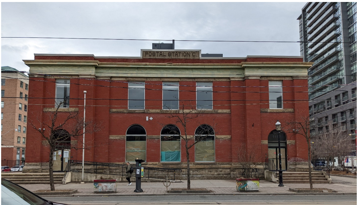
Figure 14. Principal (north) elevation of 1117 Queen Street West. (Heritage Planning, 2022)
