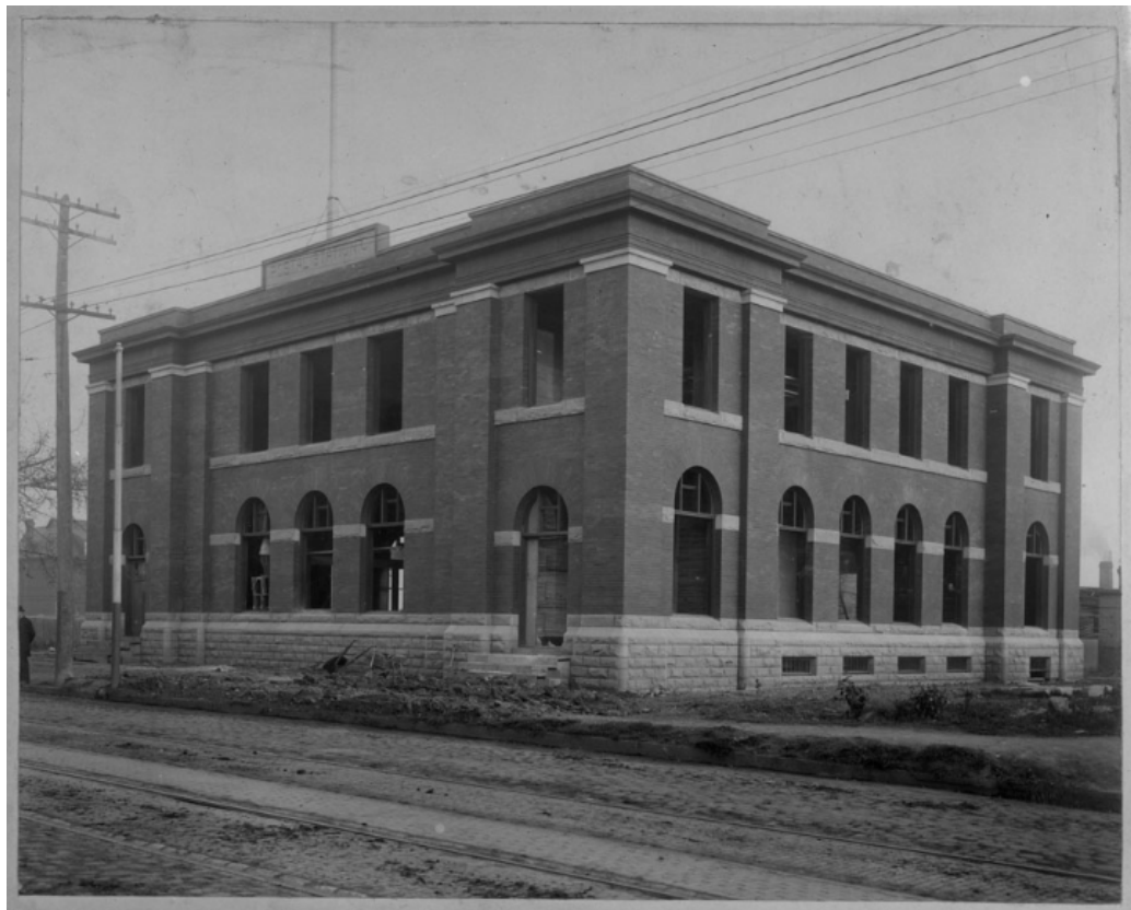
Figure 8. 1177 Queen Street West in 1902 showing the building under construction. (Library and Archives Canada)
