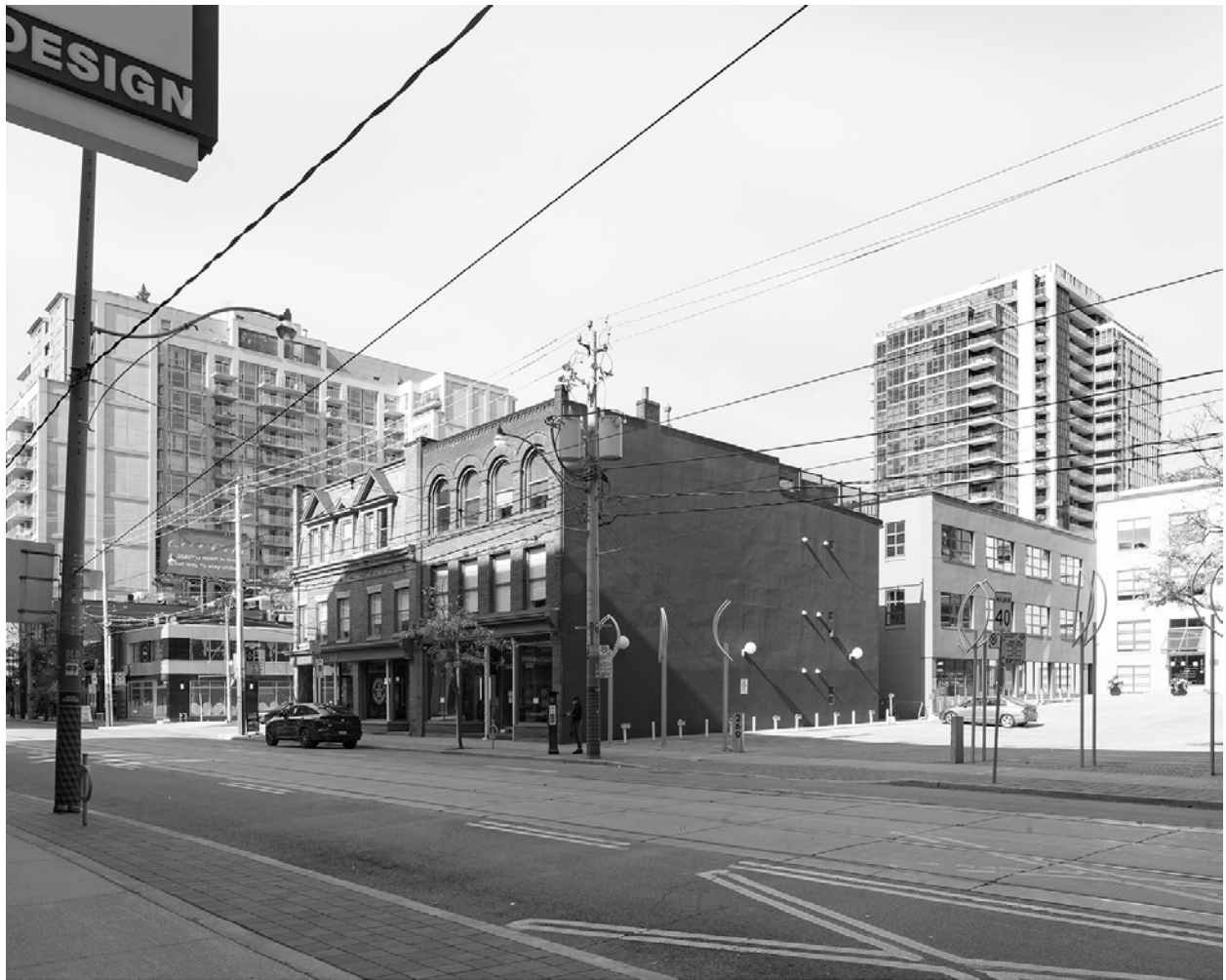
The south elevation of 254 King Street East and the south and east elevation of 256 King Street East. (City of Toronto, 2020)
