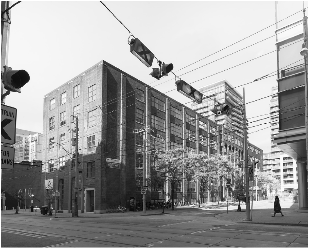
The south and east elevation of 266 King Street East. (City of Toronto, 2022)
