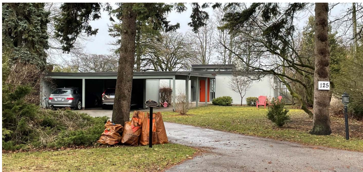
125 Sylvan Avenue: View of the principal (north) elevation, Heritage Planning, 2022
