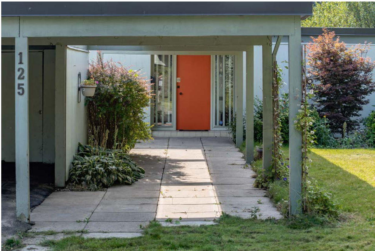
Image 13. 125 Sylvan Avenue, walkway and front door, Sutton Realty Inc., 2021.
