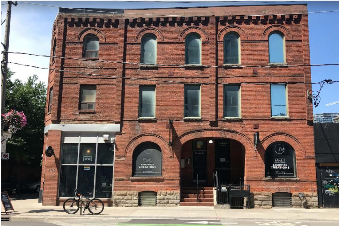
Image 16. Current photo showing the east elevation of 120-122 Sherbourne Street (Heritage Planning, 2022)
