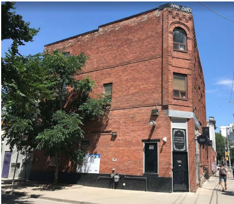
Image 18. Current photo showing the south elevation of the property at 120 Sherbourne Street (including entrance address at 52 Britain Street). (Heritage Planning, 2022)
