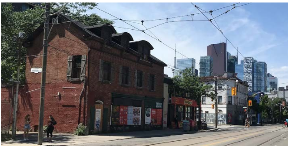
Image 12. Current contextual photo looking west and showing the historic Andrew McFarren Building in the foreground near the southeast corner of Queen and Sherbourne. (Heritage Planning, 2022)
