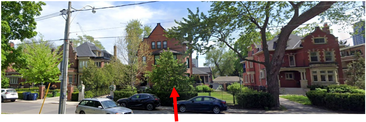
View of 33, 31 and 29 and 33 Maple Avenue from Glen Road with 31 Maple Avenue marked by an arrow (Google)
