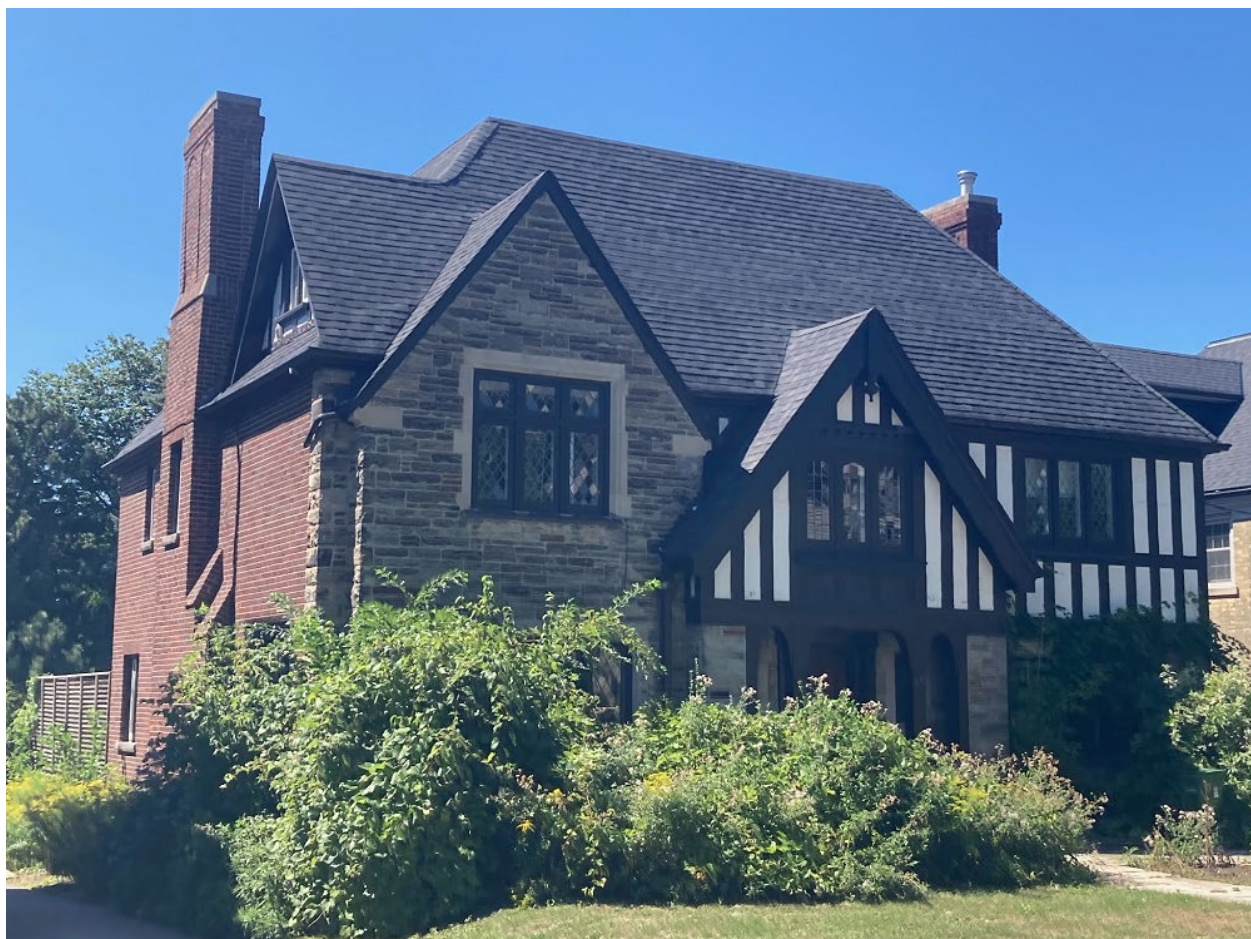
Image 5. 14 Rosemary Lane. Front (north) and side (east) elevations. Heritage Planning, 2022.
