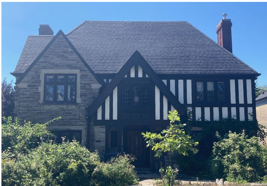
Image 3. 14 Rosemary Lane. Front (north) elevation. Heritage Planning, 2022.
