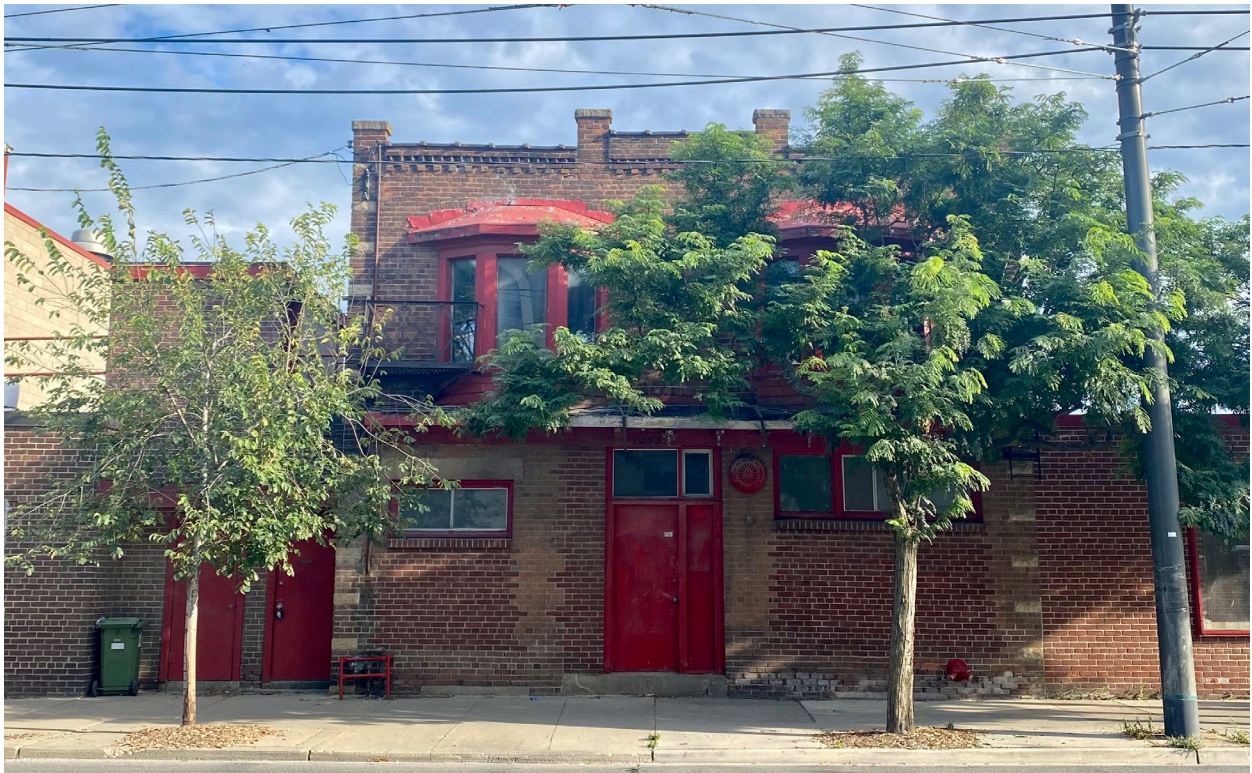
Figure 29: North elevation of the 1920-1921 structure, with the 1950 addition visible at left, 2022. (Heritage Planning)
