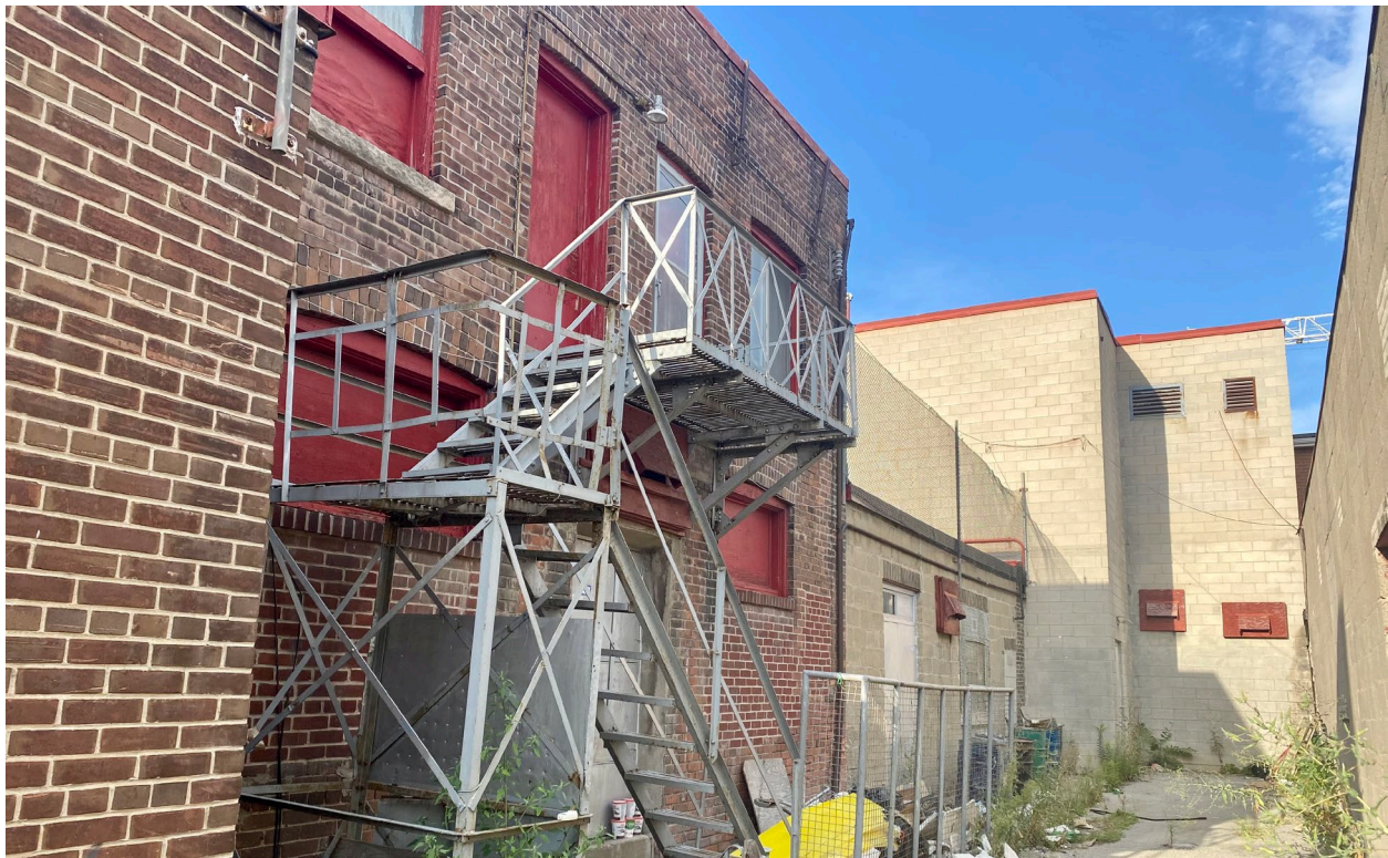
Figure 35: Northeastward view of the rear of the subject property, with the oldest (1920-1921) structure visible at left, 2022. (Heritage Planning)
