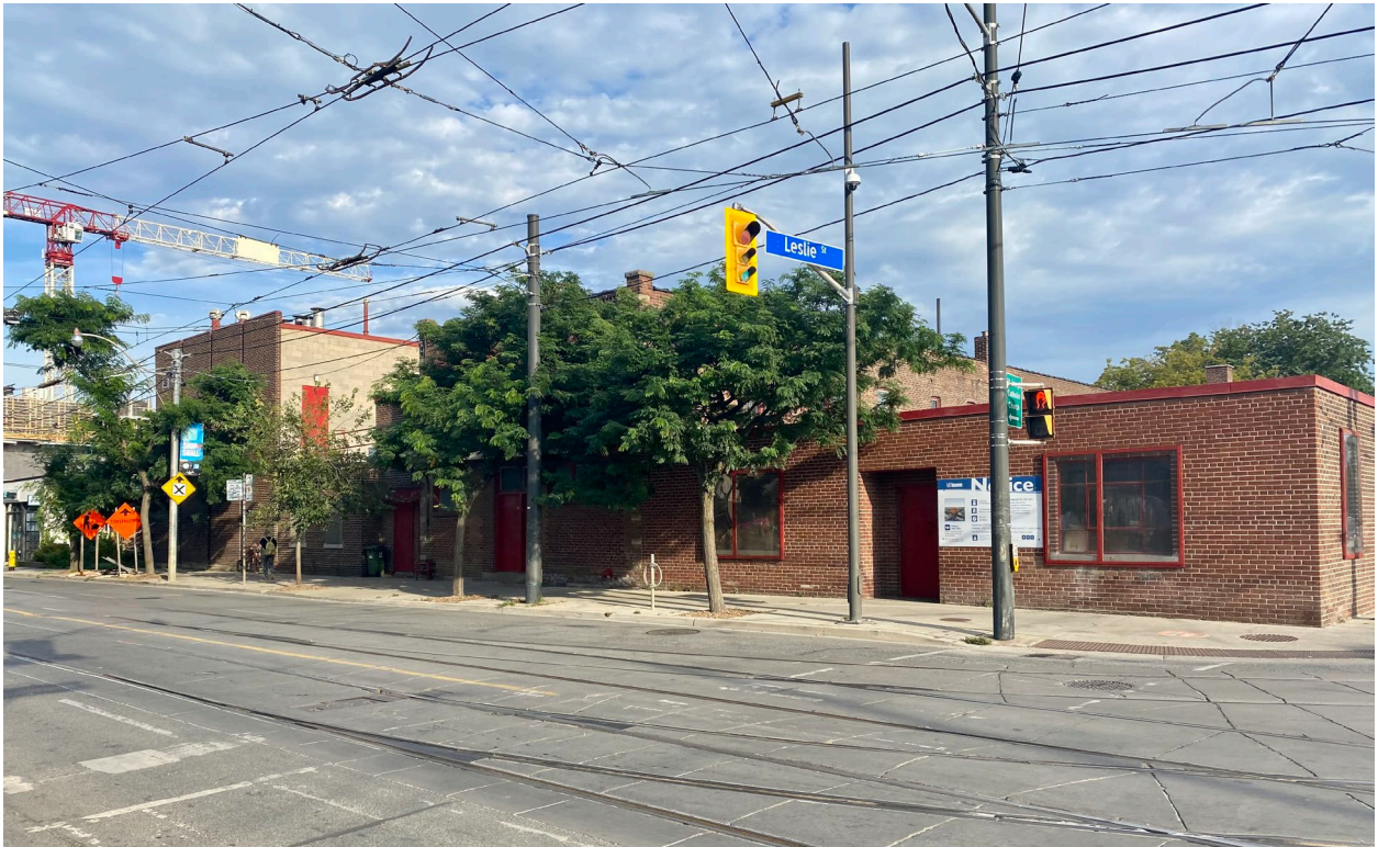
Figure 32: North elevation of 1233-1235 Queen Street East along Leslie Street, showing the c.1955 addition, 2022. (Heritage Planning)
