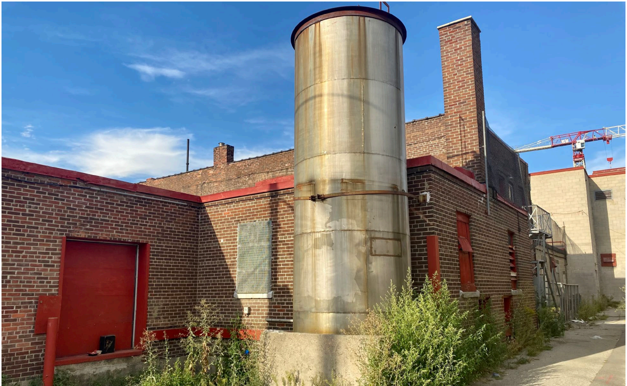
Figure 34: Southwest corner of the subject property, showing the c.1956 addition and 1960 steel tank, with the oldest (1920-1921) structure visible beyond, 2022. (Heritage Planning)
