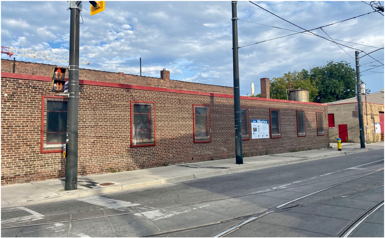
Figure 33: West elevation of 1233-1235 Queen Street East along Leslie Street, showing the c.1955 addition, 2022. (Heritage Planning)
