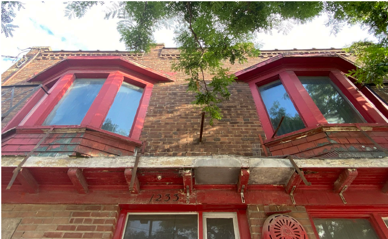
Figure 30: Details of the 1920-1921 structure, 2022. (Heritage Planning)
