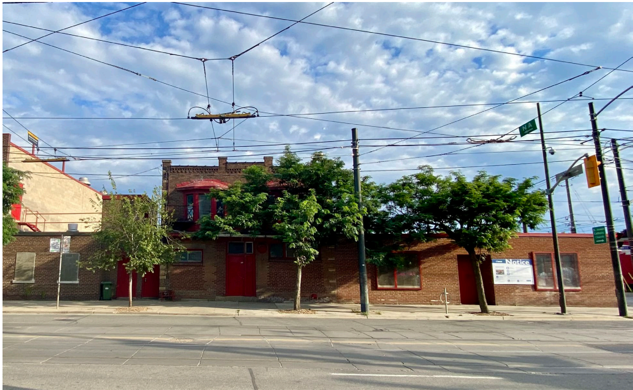
Figure 1: 1233-1235 Queen Street East, 2022. (Heritage Planning)
