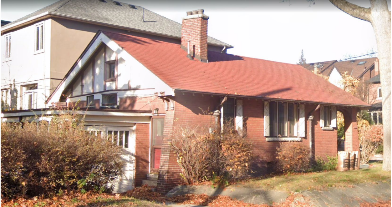
Image 15. Current image looking northwest
