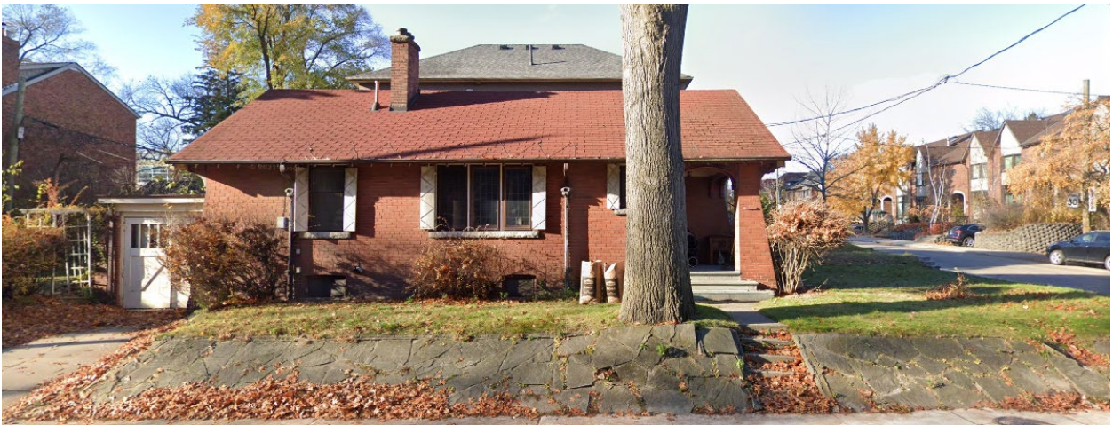
Image 14. Current image showing the east elevation including the attached single-car garage at the rear (south) end of the property.
