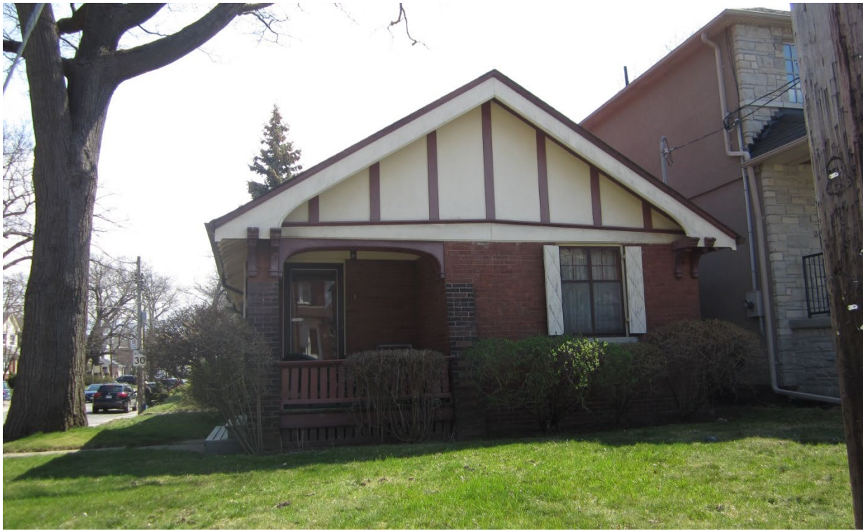
Image 12. Current image of the north elevation
