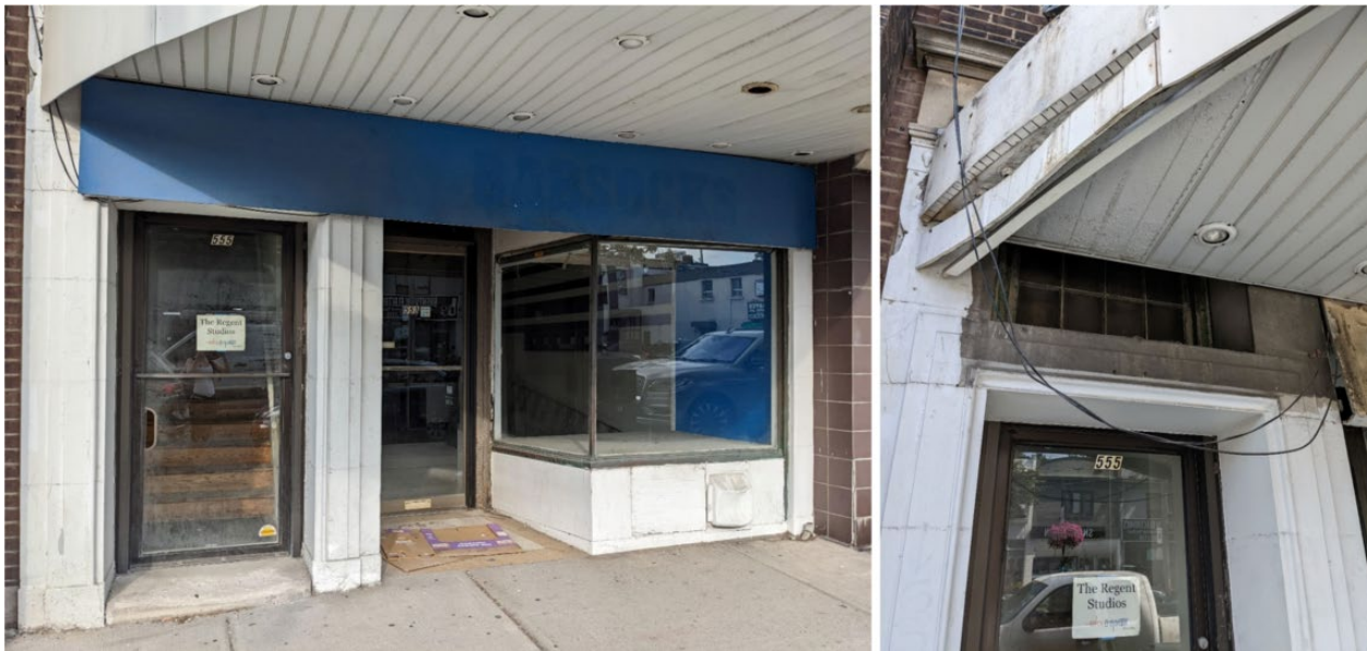
Figures 22, 23. Detail of the north storefront and entrance door surround with hoarding removed (Heritage Planning, 2022)
