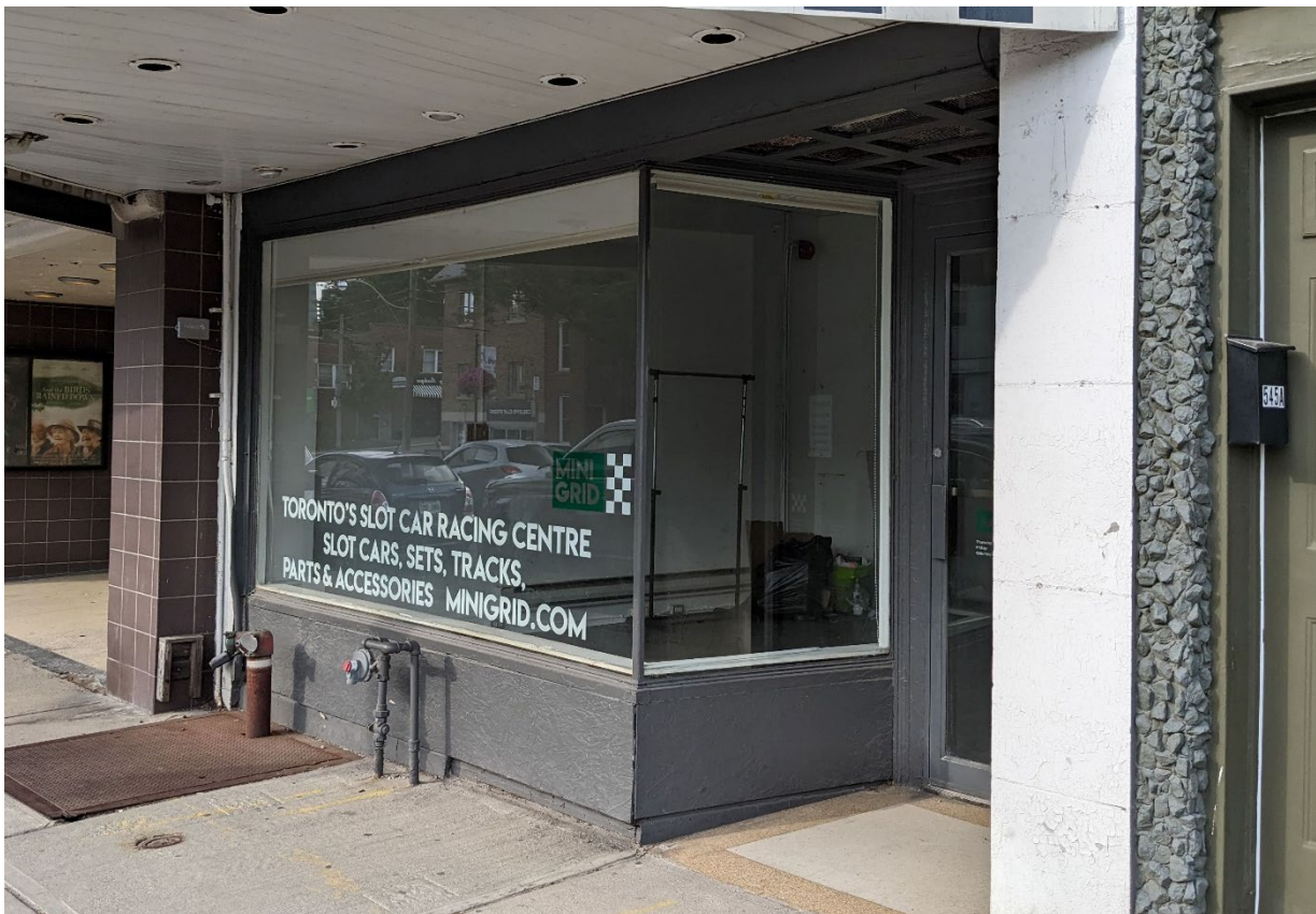
Figure 24. Detail of the south storefront (Heritage Planning, 2022).
