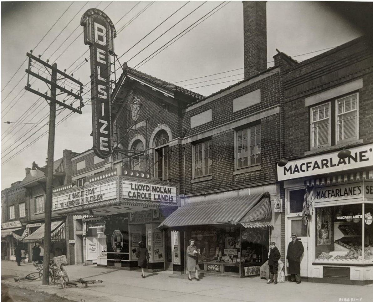
Figure 19. Archival image from 1942 showing the original casement windows, storefronts, and alterations to the front entrance and the third known iteration of the marquee and canopy. The front entrance was later redone in 1950 (Archives of Ontario).
