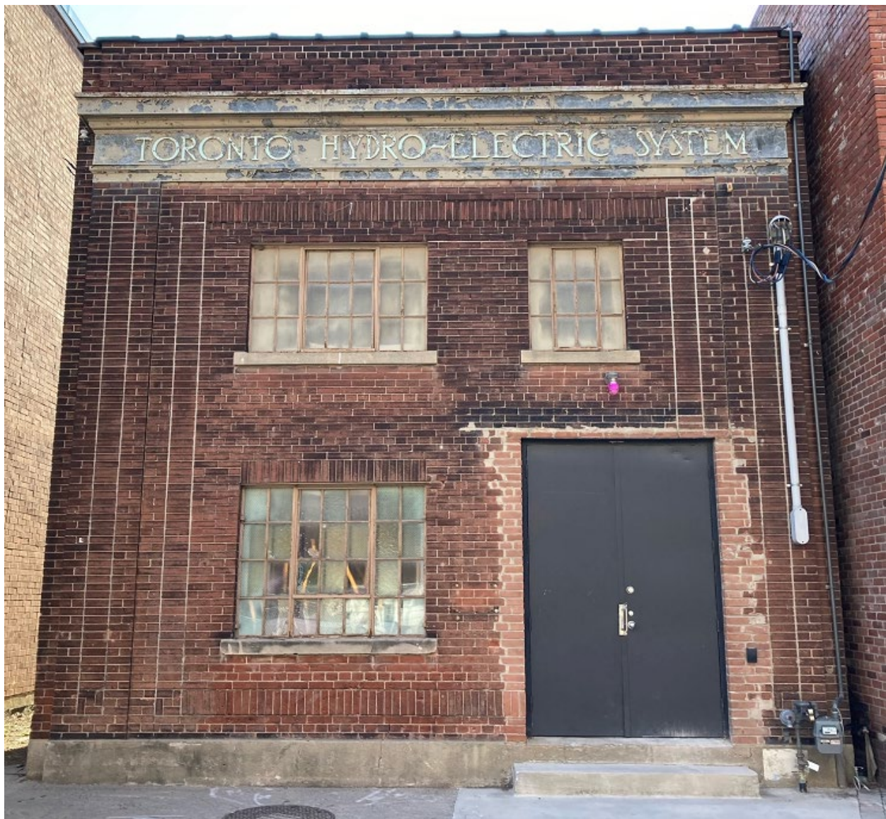
18 Portland Street. Principal (east) elevation. Heritage Planning, 2022.
