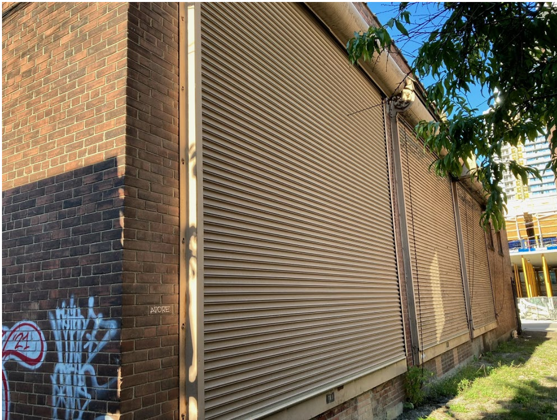
Image 13. 18 Portland Street. Side (south) and rear (east) elevations. Note the three large, metal, garage doors. Heritage Planning, 2022.
