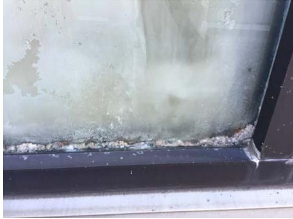
Failure of insulated glass unit at clerestory windows
