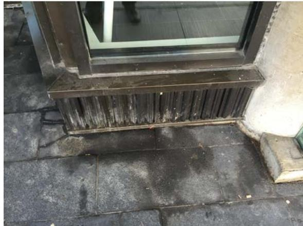
Deterioration of slate paving, and metal surfaces of siding, sill and windows
