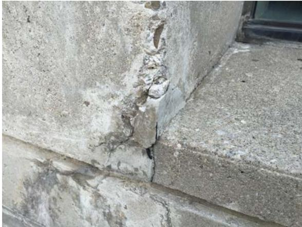
Spalling of concrete surfaces at window sills
