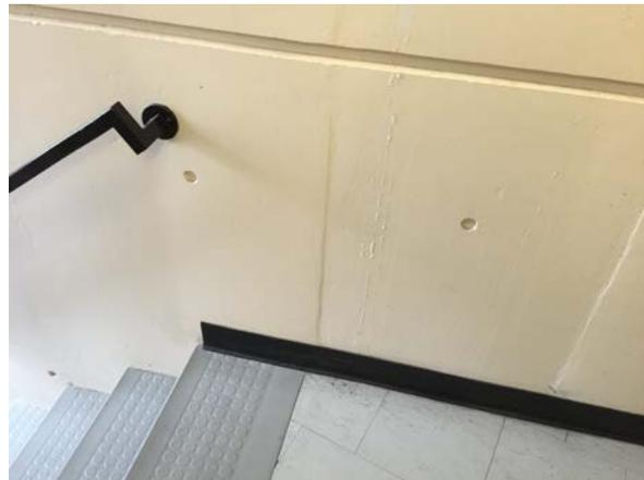
Handrail does not extend over the top landing
