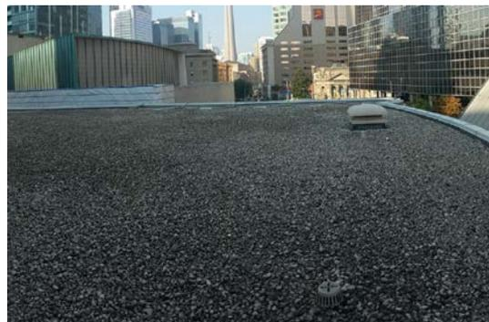
Roof drain and cover in good condition (lower right) with an exhaust fan cap in the background.
