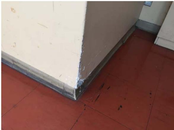
Damage drywall finish at corner
