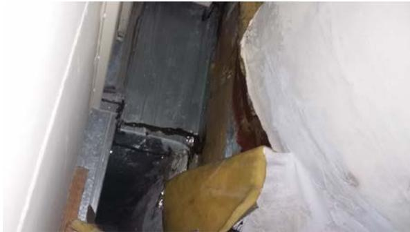
Damaged insulation on AHU S5.
