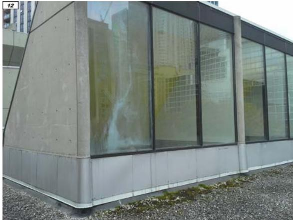
Failure "Fogging" at clerestory insulated glass unit
