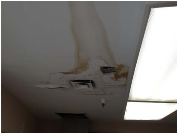
Water damage at drywall ceiling
