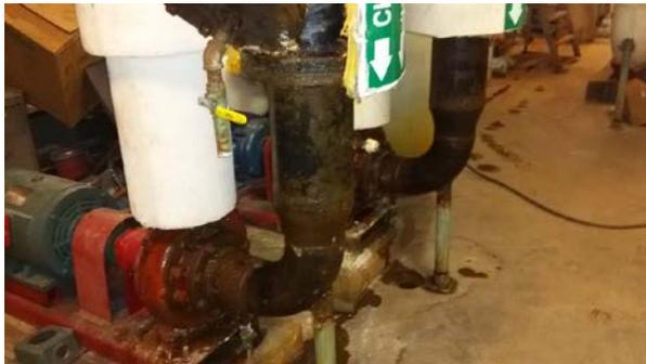
Chilled water return pumps and piping with missing and damaged insulation with visible condensation.
