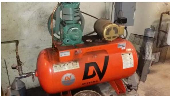
Air compressor with belt guard removed.
