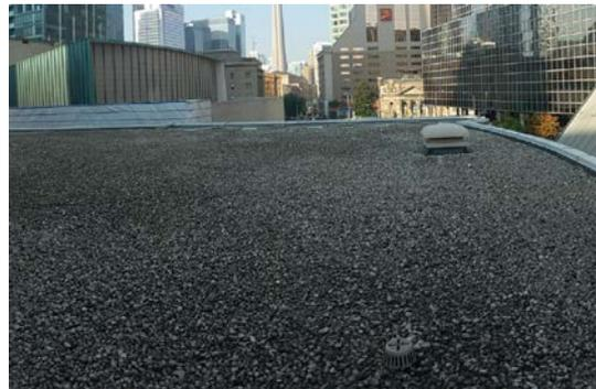
Roof drain and cover in good condition (lower right) with an exhaust fan cap in the background.
