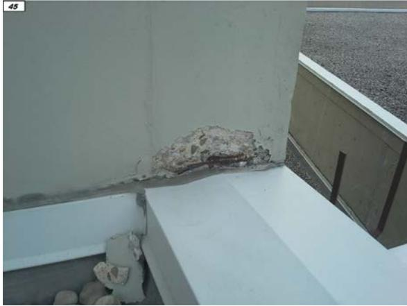
Spalling of concrete surfaces at curbs abutting concrete walls
