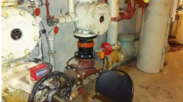
Sprinkler system valves. Valve in centre of image is in good condition. Valve in left of image is in fair condition.
