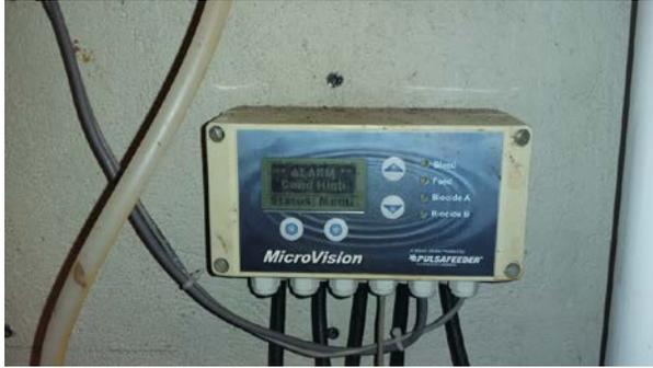
Condenser water chemical treatment control panel showing High Conductivity Alarm.
