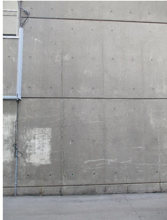
S.14: Cracking of concrete walls on all exterior elevations.
