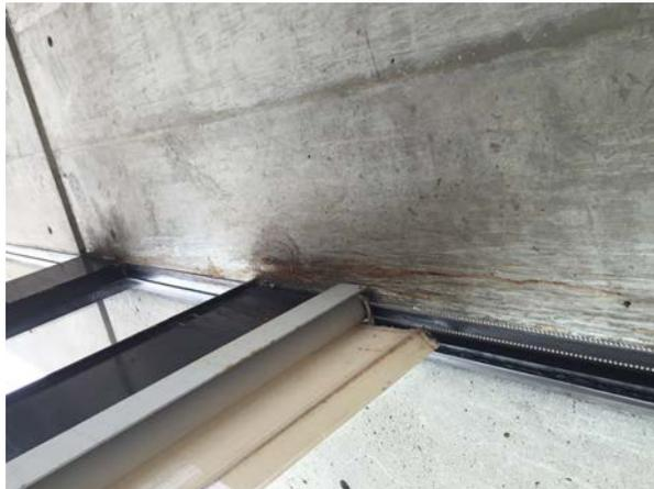
Water stains at interior concrete surface due to moisture condensation
