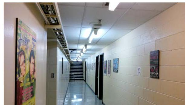
Photo 10: Typical service corridor wrap-around luminaires
