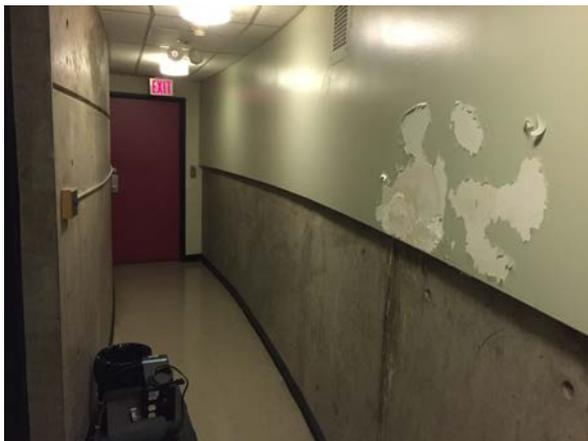
More drywall damage due to water infiltration
