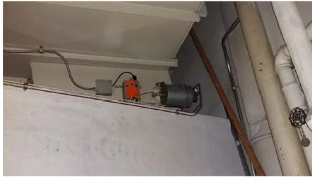
New motorized damper actuator connected to the building automation system with a decommissioned pneumatic actuator in the foreground.
