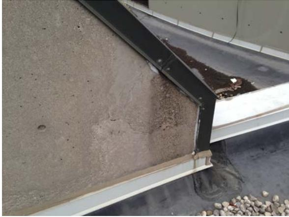
Old and deteriorated sealant/flashing at clerestory
