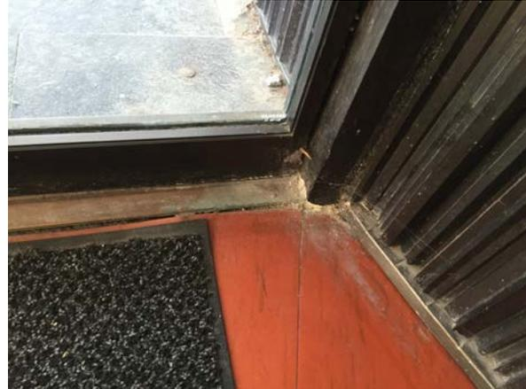
Damage from salts at bottom sill of window and deteriorated flooring
