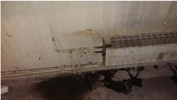
Storage room hydronic radiator in poor condition.
