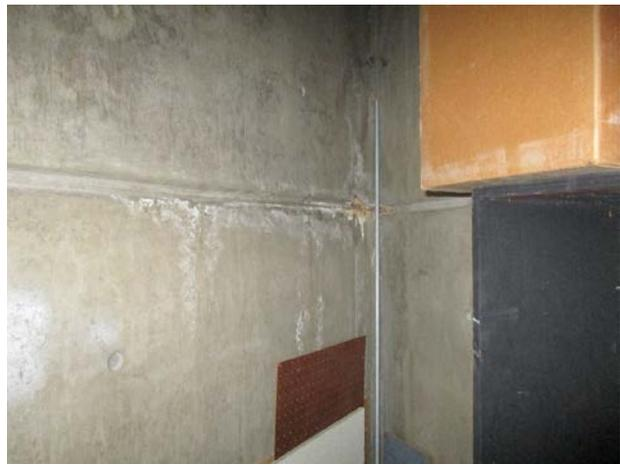
S.6: Roof of the storage room adjacent to the sound control and projection rooms has been leaking.
