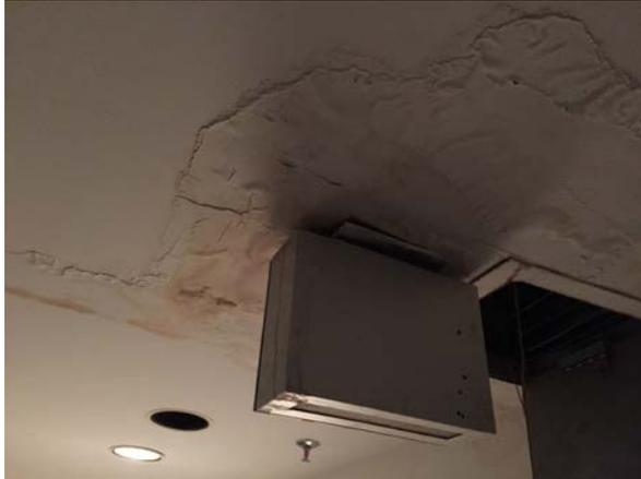
Water damage at drywall ceiling
