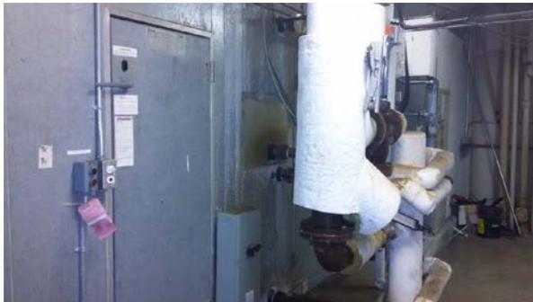
AHU S4 chilled water piping with missing insulation and visible condensation.
