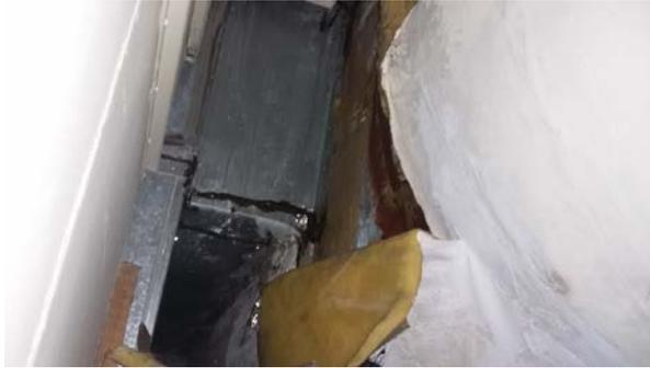
Damaged insulation on AHU S5.
