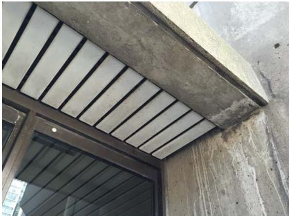
Roof water run-off and damage at east entrance on Front Street
