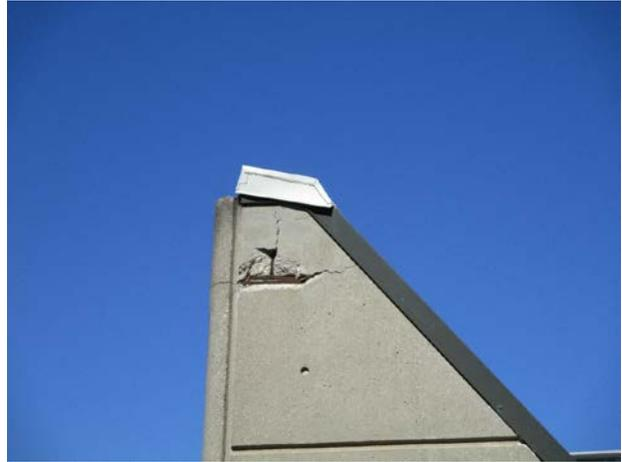
S.13: Spalling of concrete walls on all exterior elevations.
