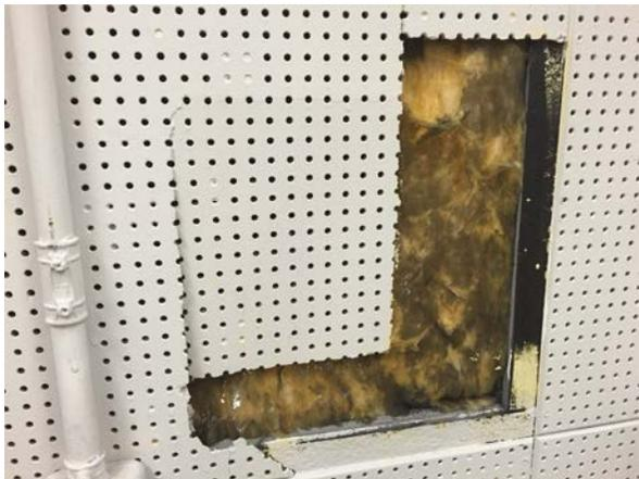
Old and deteriorated wall-mounted acoustical material
