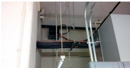
Photo 4: Branch "corflex" feeder conductors
