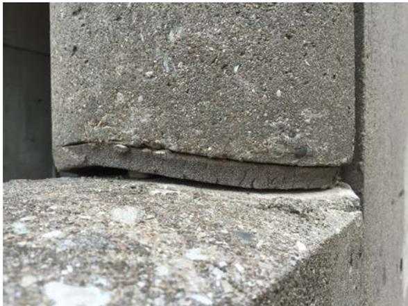
Dry sealant at joint between concrete shear wall and parapet
