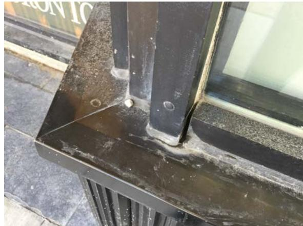
Old sealants and flashing no longer weathertight
