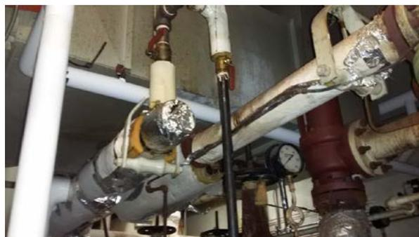
Poor insulation on piping associated with steam heat exchangers C-1 and C-2.
