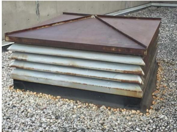
Old and deteriorated mechanical louvre
