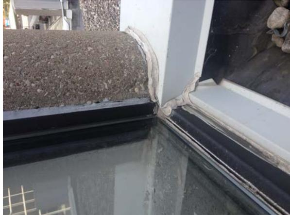
Deteriorated sealant and flashing at clerestory's curb
