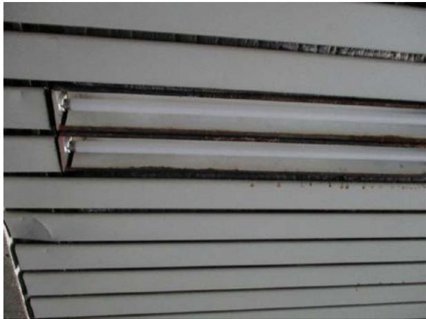
S.4: Corridor at east exit stair showing signs of water ingress (219).
