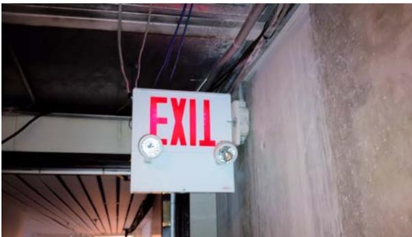
Photo 15: Typical combination exit sign (upside down text)
