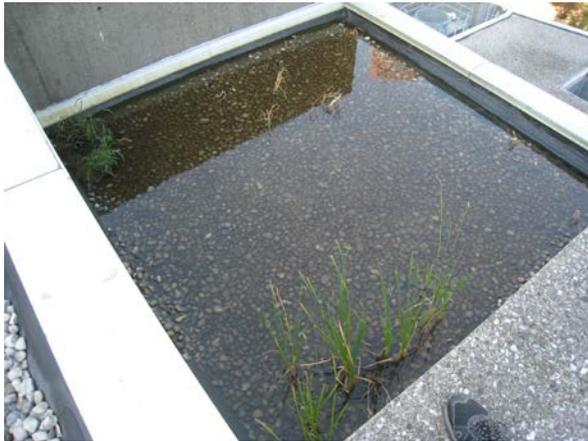
Water ponding over high roof area
