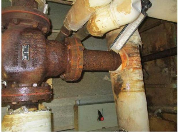
S.3: Condensation dripping from mechanical units and connections is pooling in mechanical rooms.
