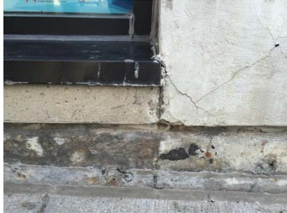
Deteriorated sill flashing and bottom of wall
