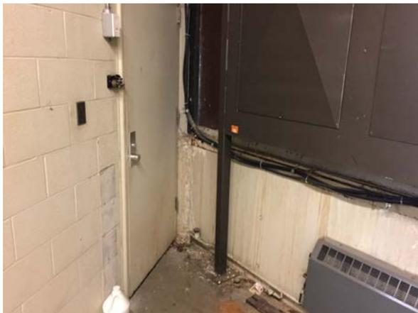
Substantial water infiltration and damage to substrates
