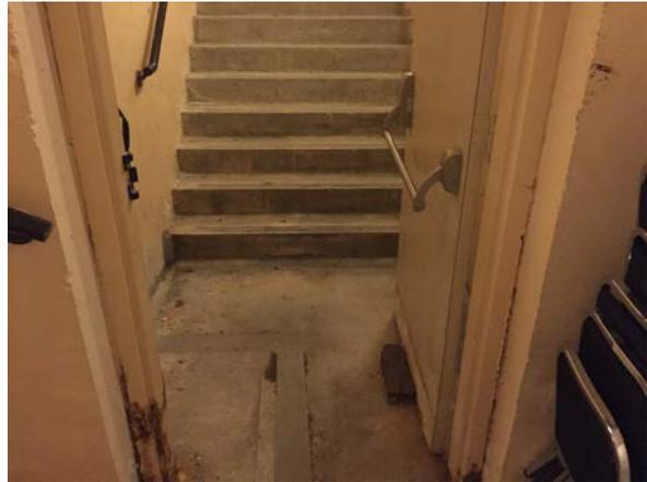
Fire door propped open with weight and deteriorated flooring
