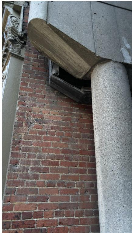
S.15: Infill construction between the SLCA and the neighbouring building to the east has failed.
