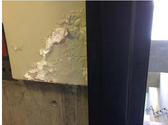
Damage at drywall surface from water infiltrations
