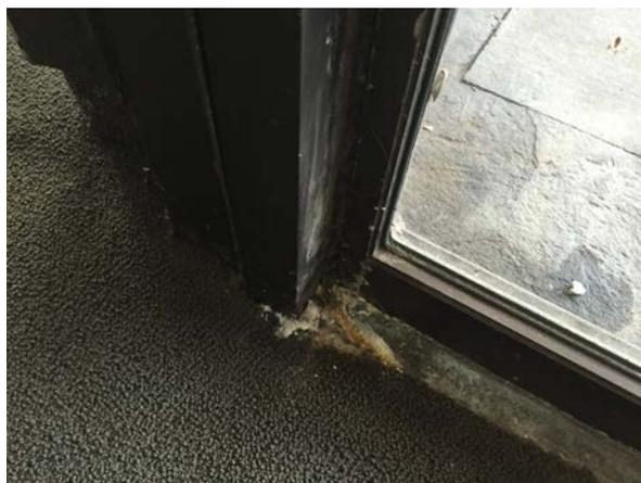
Damage from salts at bottom sill of window
