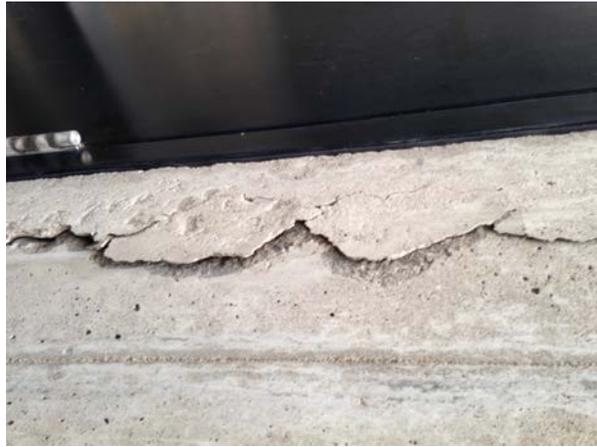
Spalling of concrete surfaces at clerestory walls
