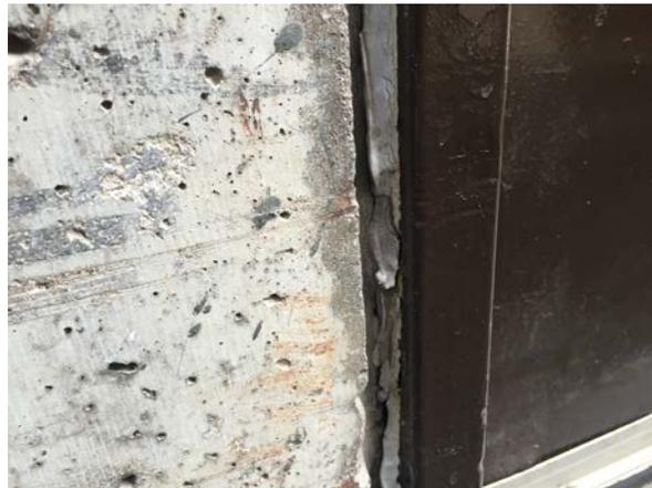
Dry sealant between window frame and concrete wall
