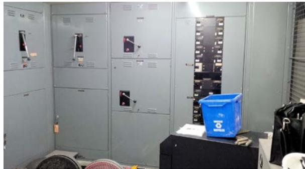
Photo 2: 2500amp;208/120v,3p,4w main switchboard
