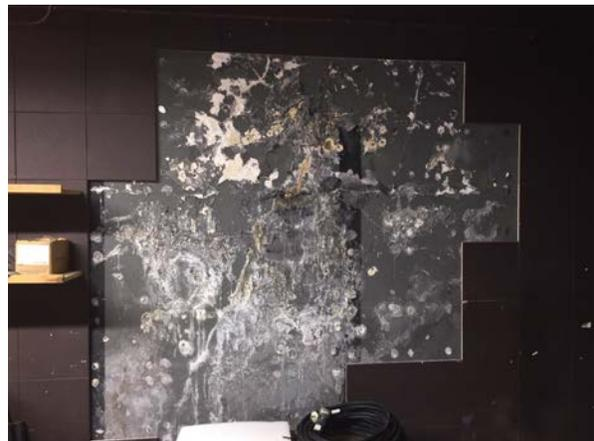
Water damage observed over interior concrete wall surfaces
