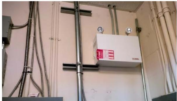
Photo 14: Typical emergency battery lighting unit
