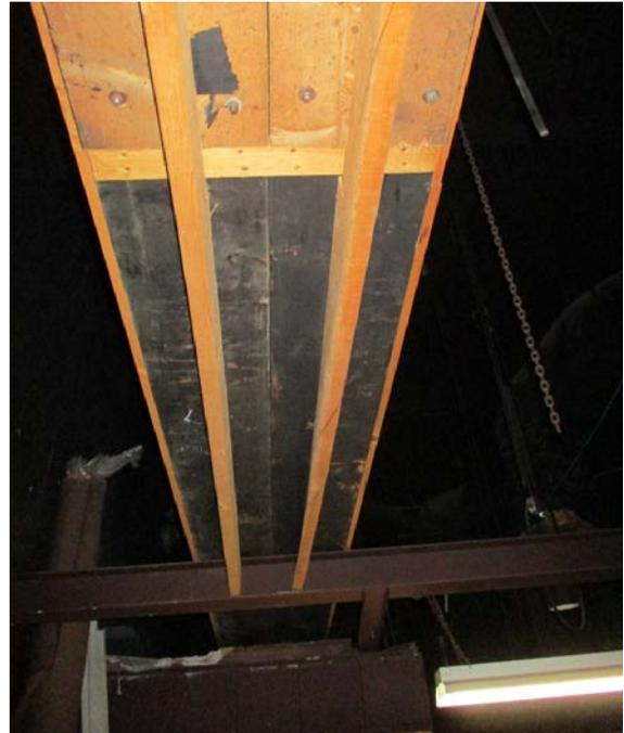
S.7: Unstable wood plank ramps installed in backstage areas behind light slot 203, 204 and associated service areas.
