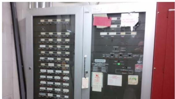
Photo 16: Existing Fire Alarm Control Panel (FACP)
