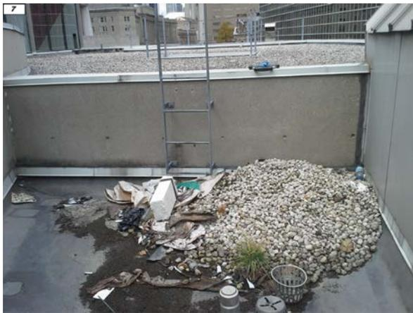
Debris accumulated over roofing membranes
