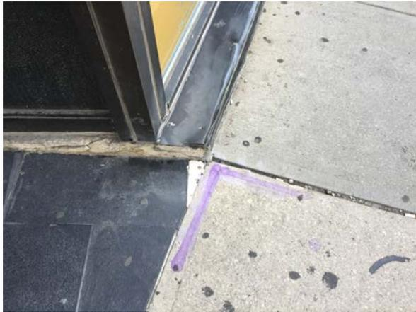
Sag and cracking of exterior paved surfaces at Scott and Front Street
