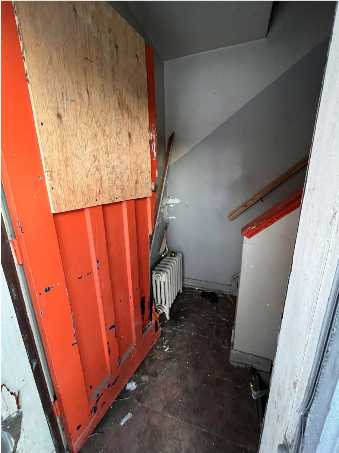
18 CORDOVA AVENUE - SIDE ENTRANCE
