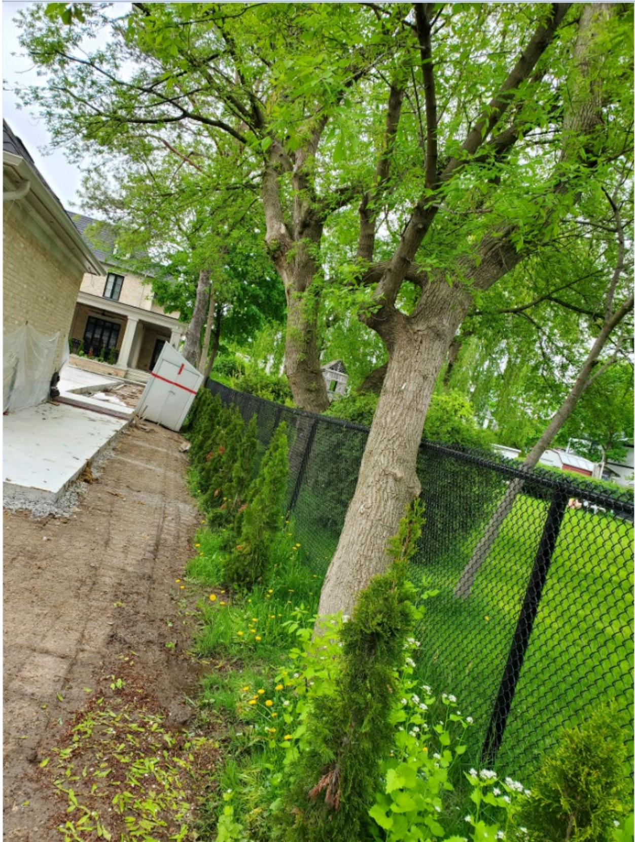
Attachment 3: Photo of south pool enclosure fence with tree from neighbour's property
