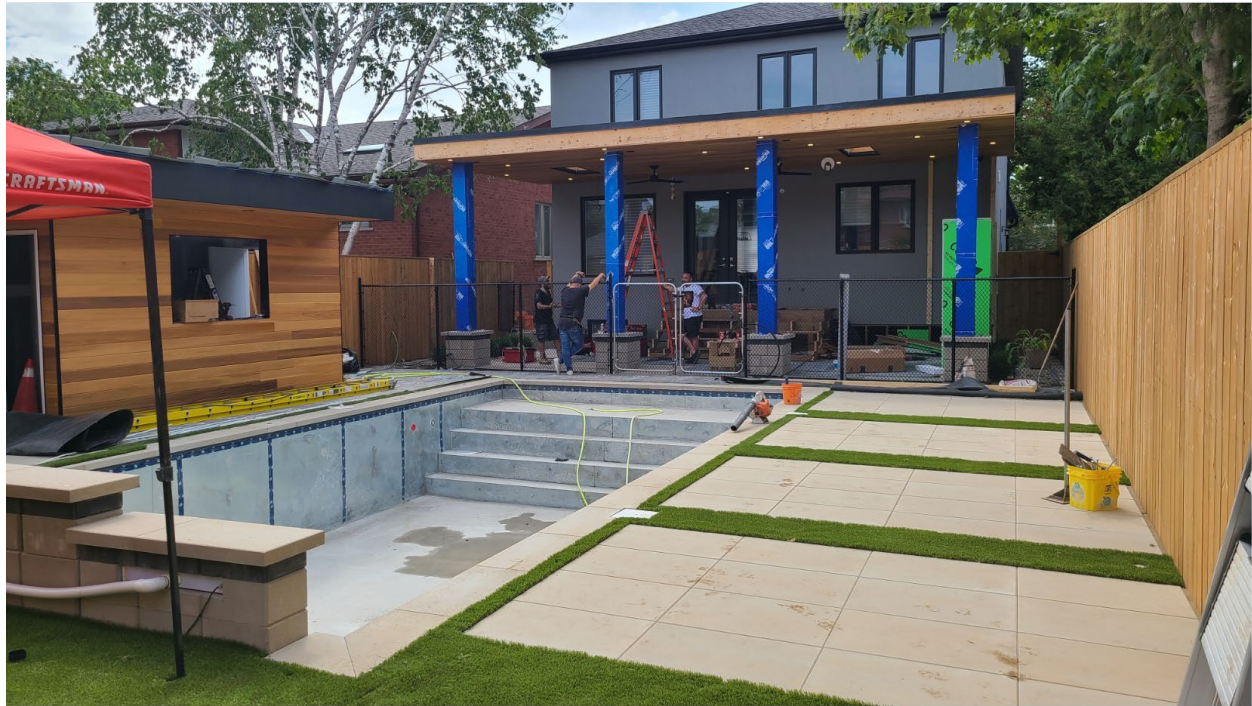
Attachment 5: Photograph of north perimeter fence (photo taken facing West)
