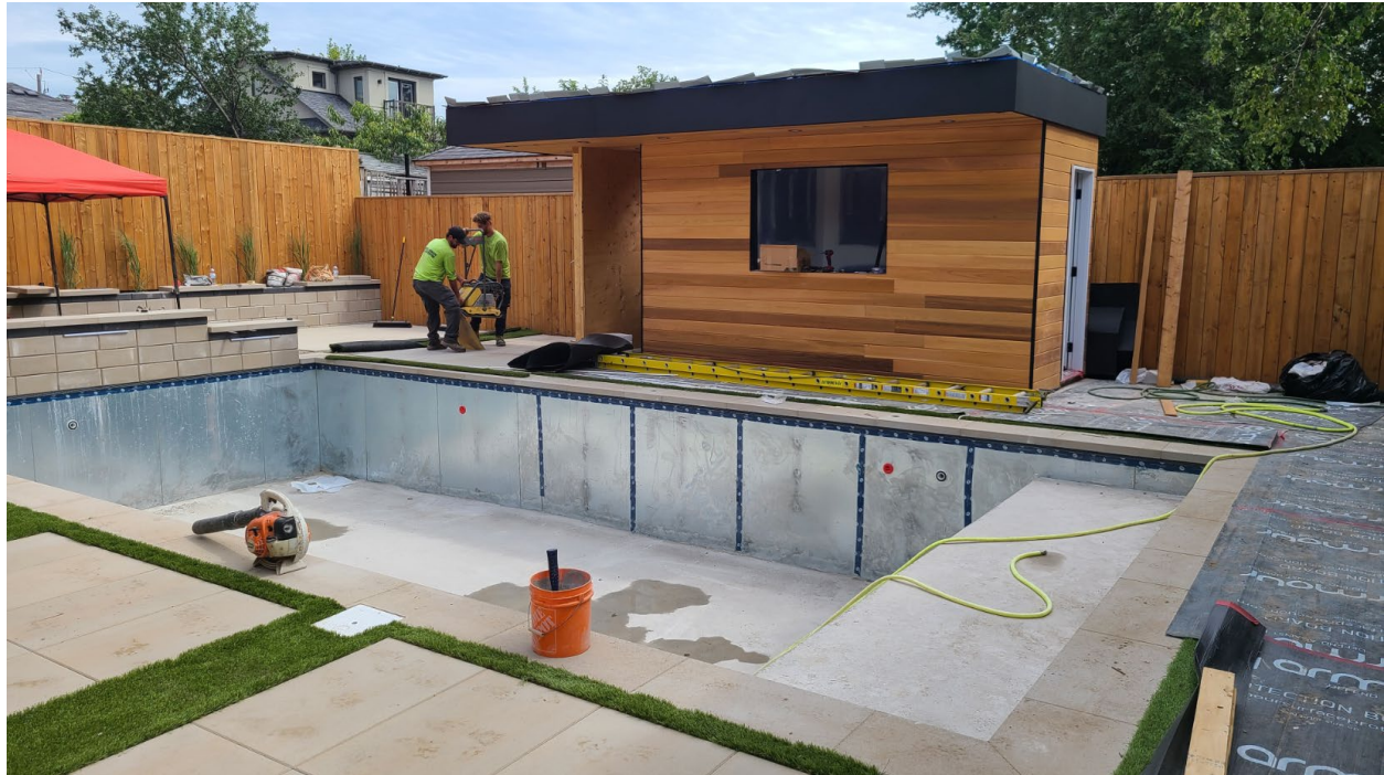
Attachment 3: Photograph of perimeter fence (photo taken facing South East)
