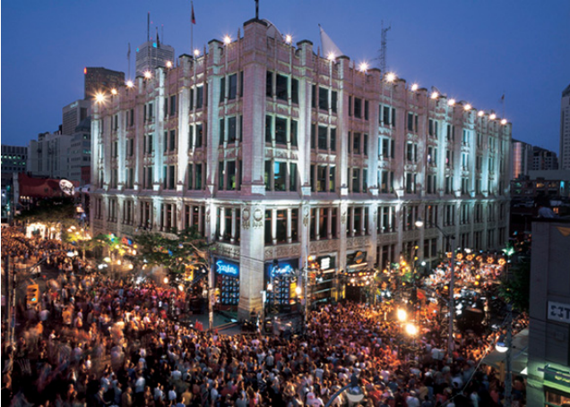
ChumCity Building, Queen Street West, Toronto
