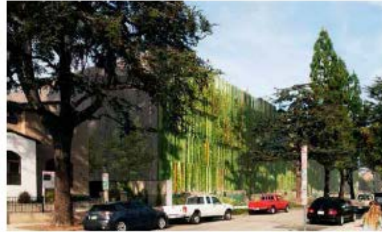
Figure 6.19: Culver Studio Parking Structure Perimeter Wall Treatment, Culver City, USA.
