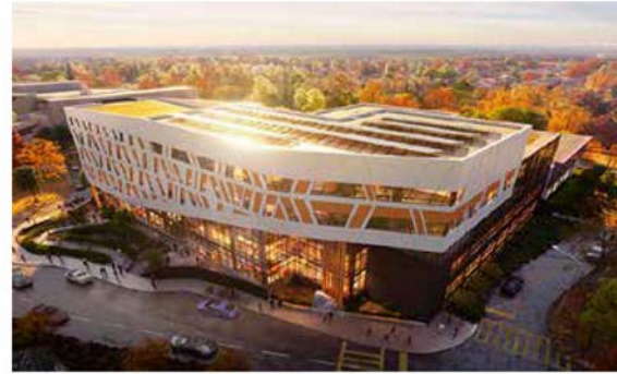
Figure 1.13: A net zero carbon building. Centennial College Mass Timber Building, Toronto.
