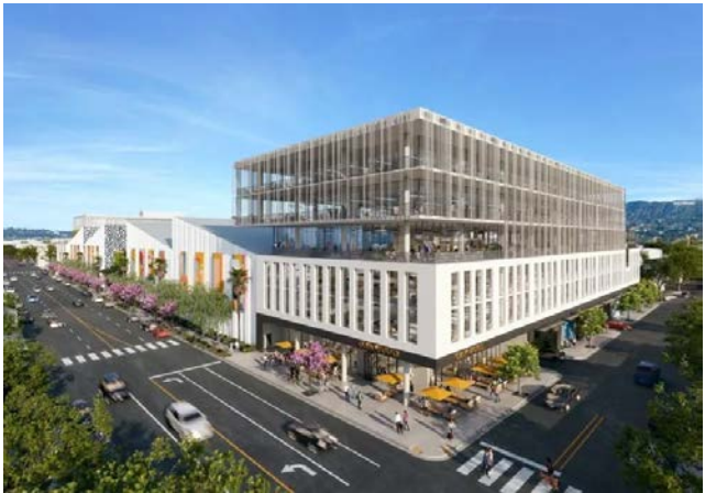
Echelon Studios Offices, Hollywood, USA
