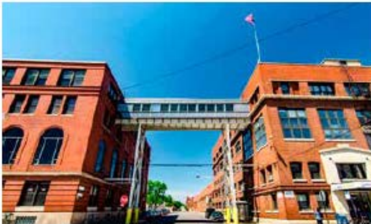
Figure 6.20: Cinespace Elevated skybridge anchored by perimeter buildings, with recessed gateway
