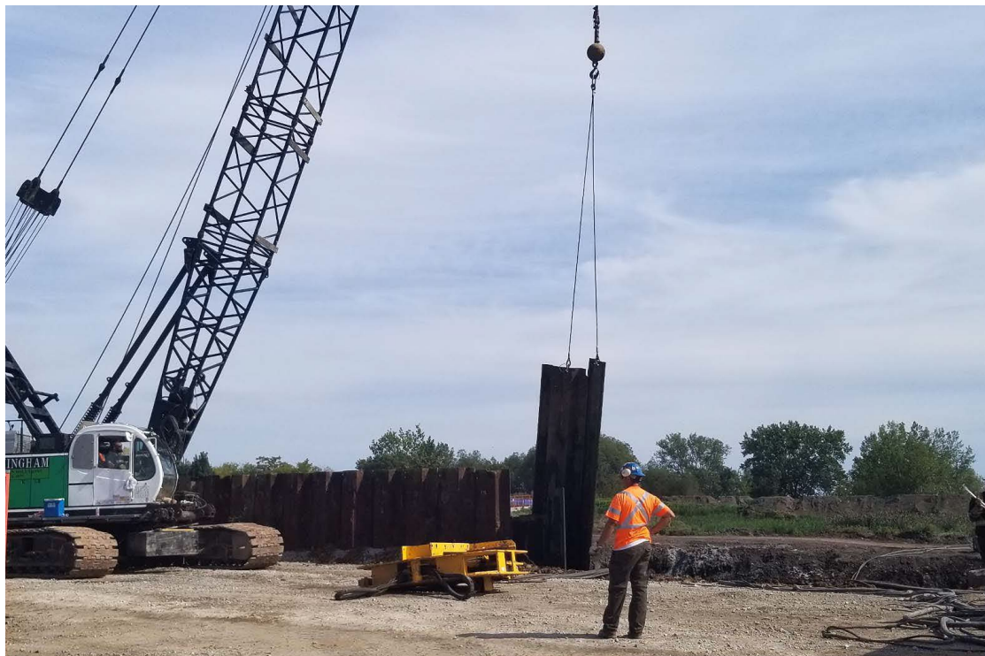
Figure 2 – Removal of buried steel sheet piles
