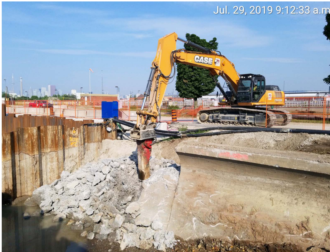
Figure 3 – Demolition and removal of buried seawall
