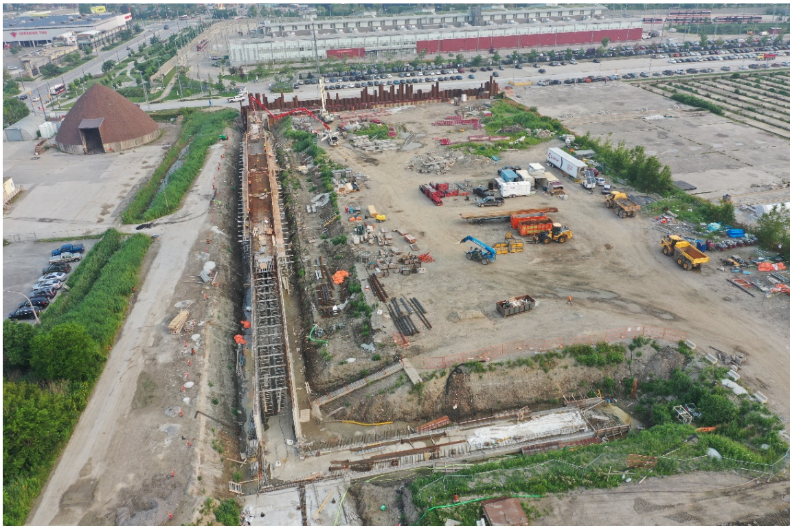
Figure 8 – West Bypass Conduits
