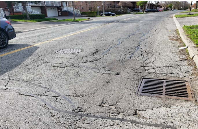
Figure 14: Existing conditions photos of Sentinel Road. The photos show the poor asphalt and sidewalk conditions.
