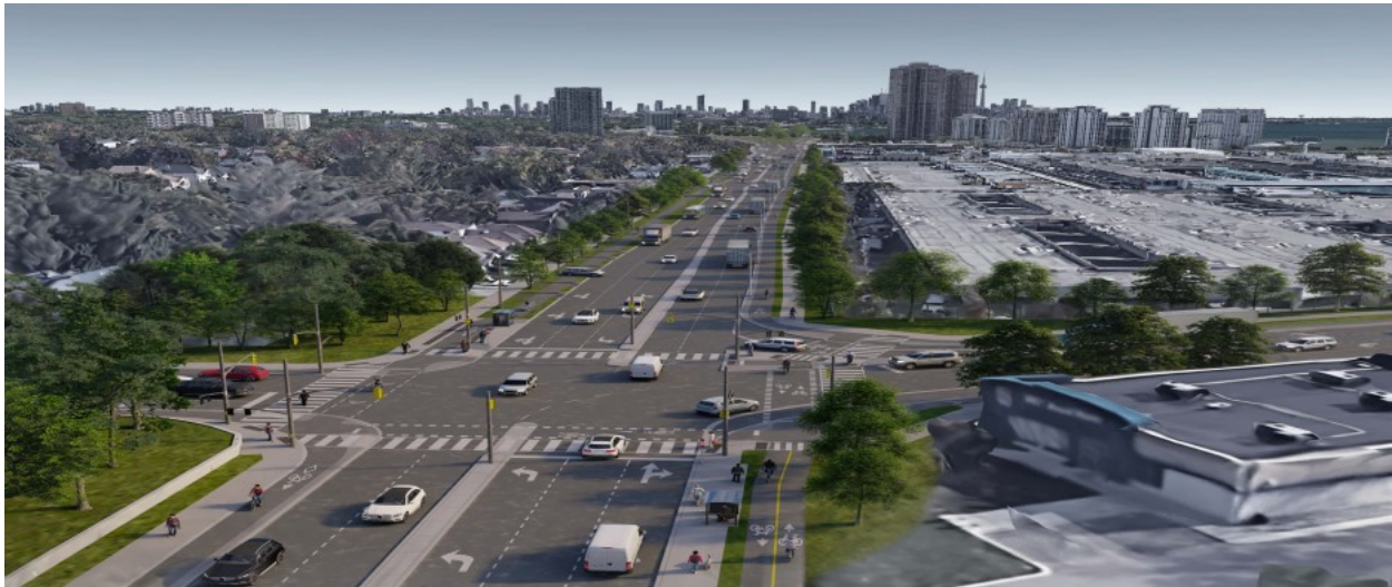
Figure 25: Artist rendering of The Queensway and Park Lawn Road Intersection. A new median, cycle tracks, protected intersection features, truck aprons, improved bus stops, new planted areas and wider sidewalks are proposed on The Queensway.
