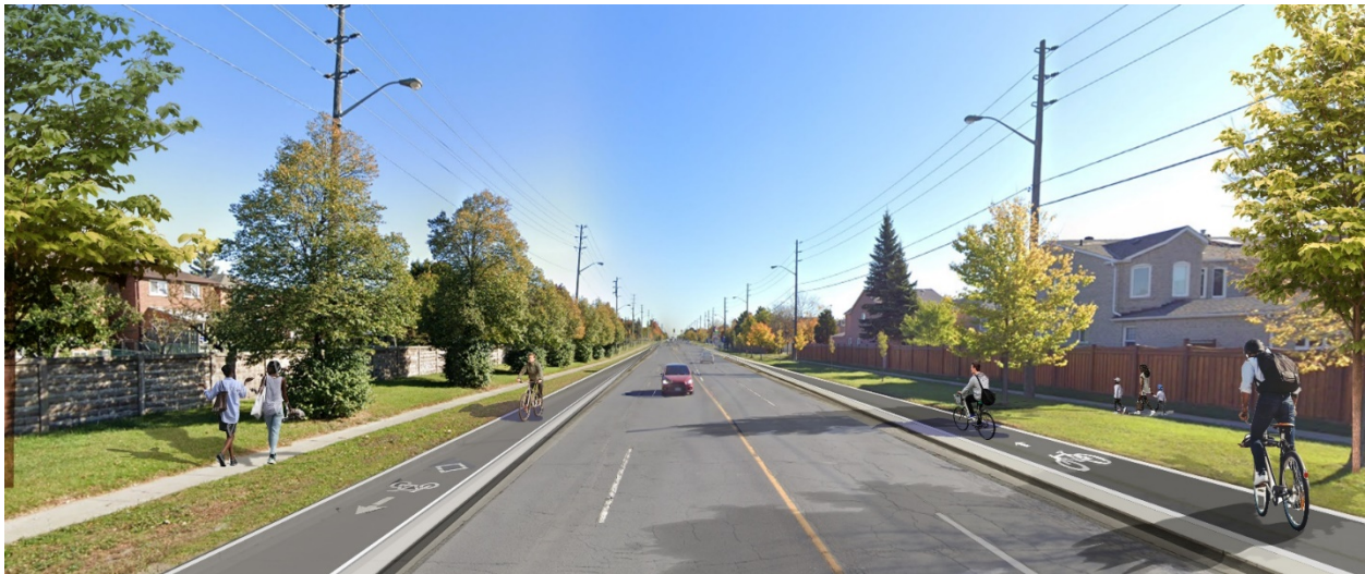
Figure 22: Artist rendering of Steeles Avenue East including two motor vehicle lanes in each direction and new uni-directional raised cycle tracks.
