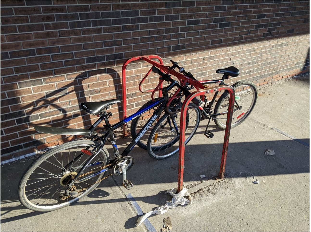
Figure 1: Victoria Van Horne Plaza Bicycle Parking (in front of Value Village). Note the visible rusting on the rack.
