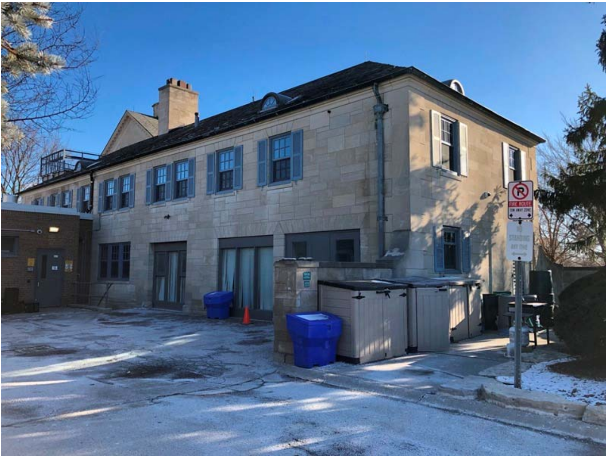
5. North and west elevation of the service-garage building with the gable of the main house beyond
