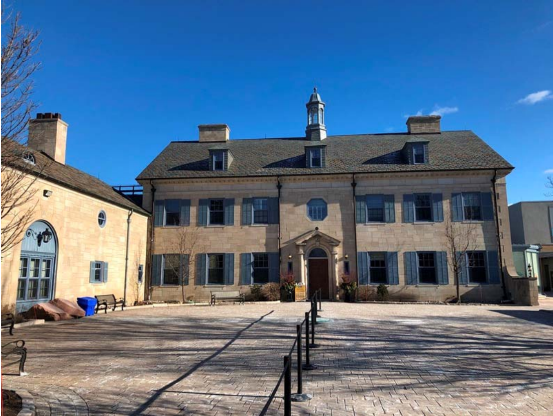
3. View of the forecourt with the service-garage building, left and the house, right
