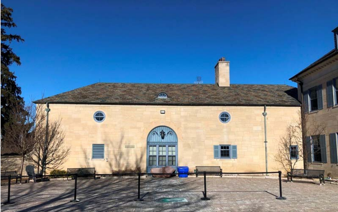
4. View of the service-garage building, south elevation
