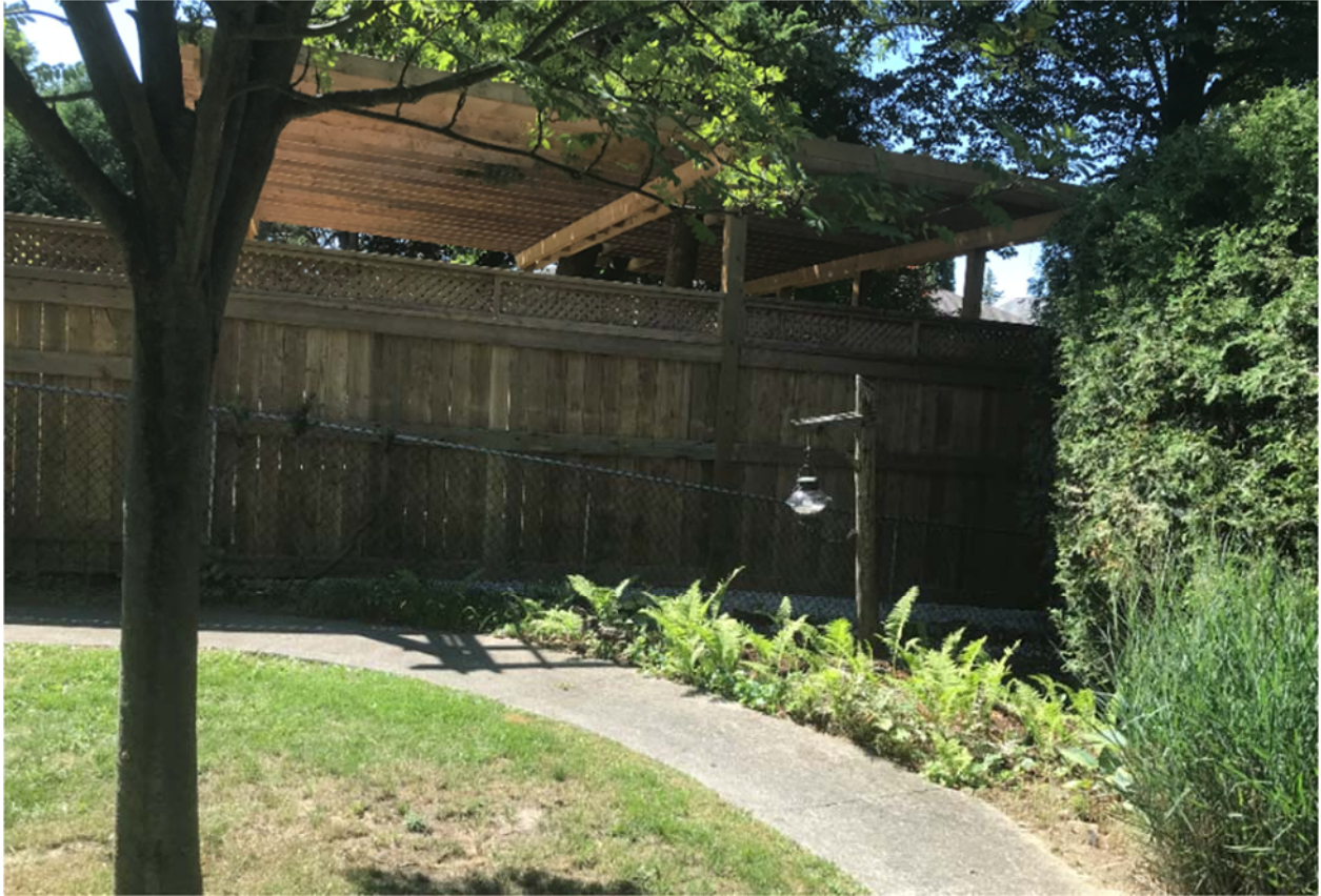
Attachment 3: Picture of Fence/Pergola structure from neighbouring property (36 Rollscourt)
