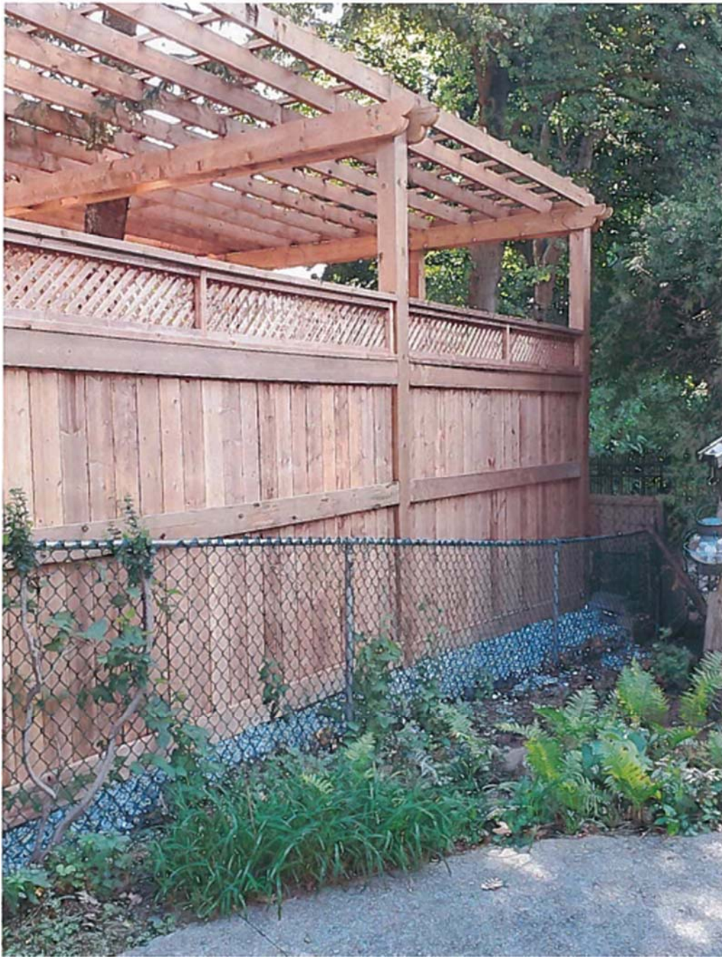
Attachment 4: Picture of Fence/Pergola structure from neighbouring property (36 Rollscourt)
