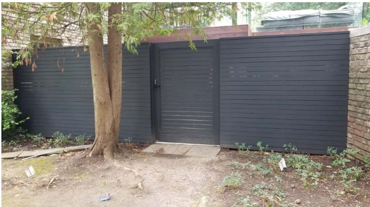
Attachment 2: Photo of wooden fence
