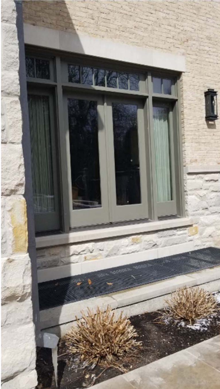
Attachment 4: Rear of house
