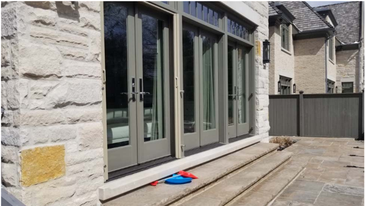
Attachment 3: Rear of house
