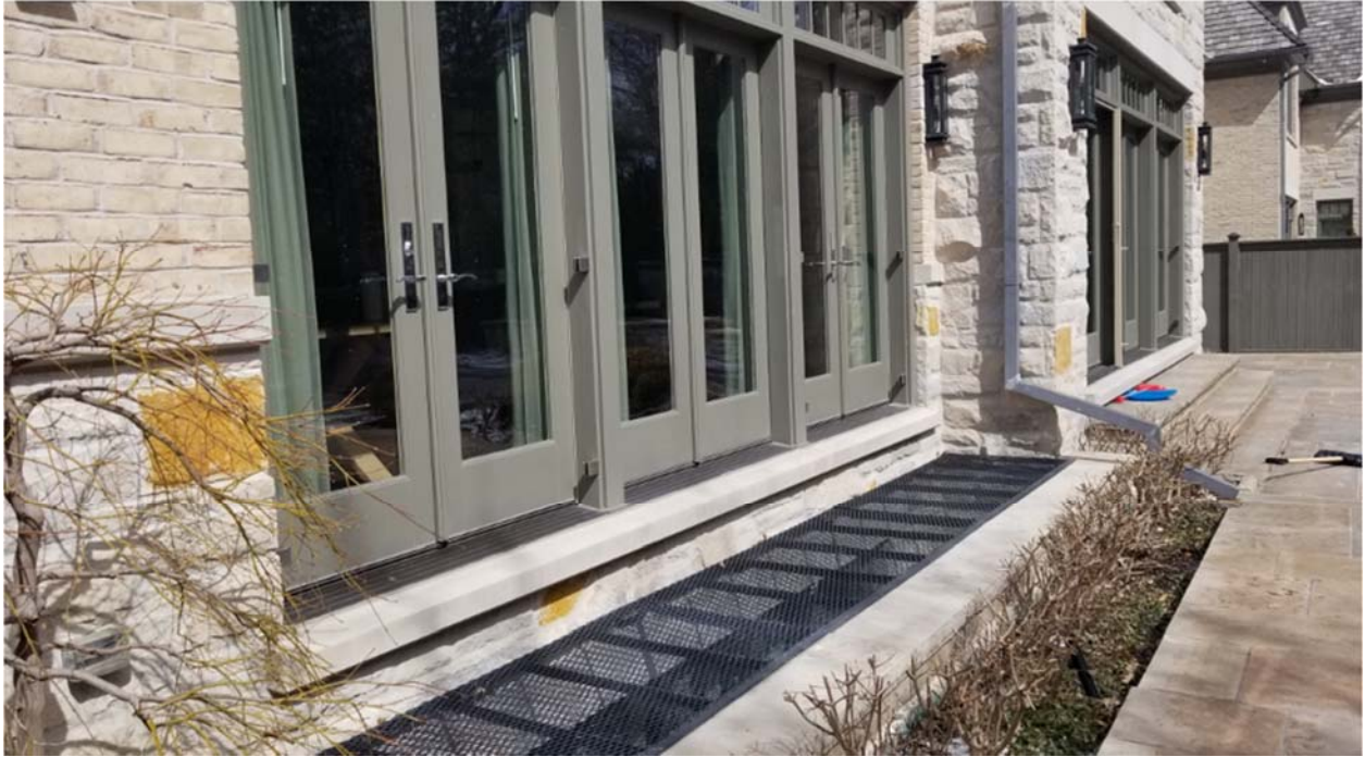
Attachment 2: Rear of house
