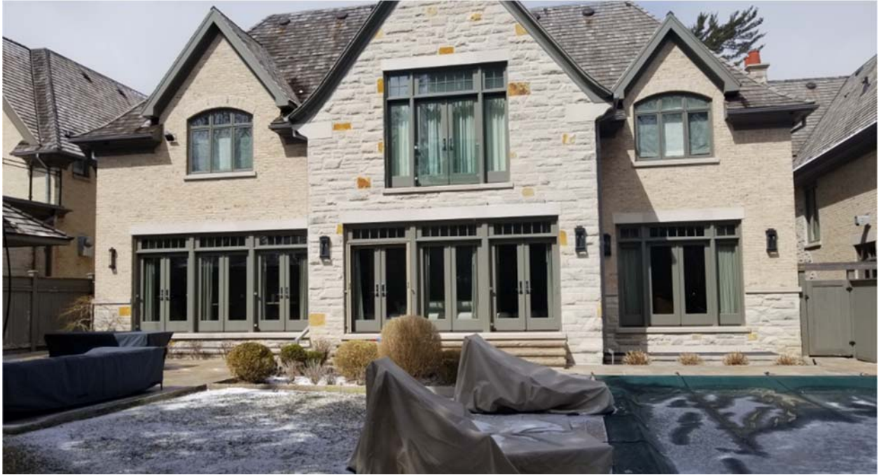
Attachment 5: Rear of house
