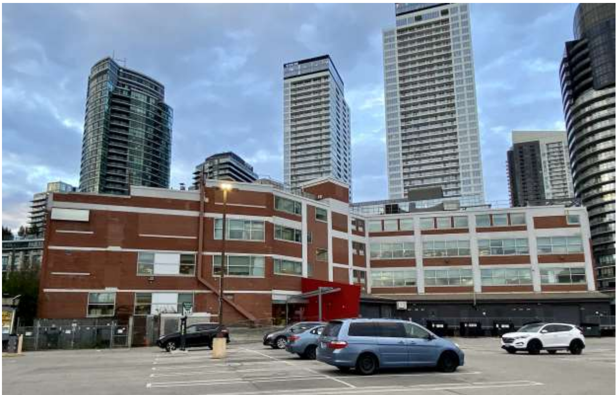
Rear/South Elevation. Non-Street facing
