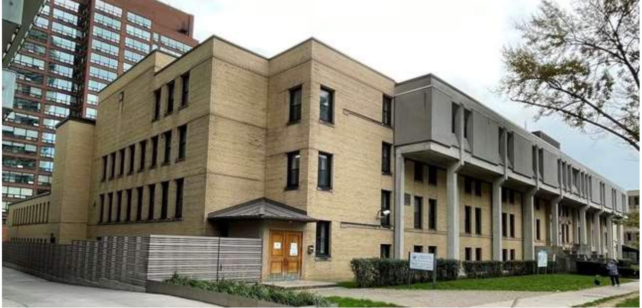
38. St. Basil's Seminary, side (east) and principal (north) facades with later additions including the two-storey extension (far left), 4th floor extension on the north elevation and the new single storey entrance. (HP, 2021)
