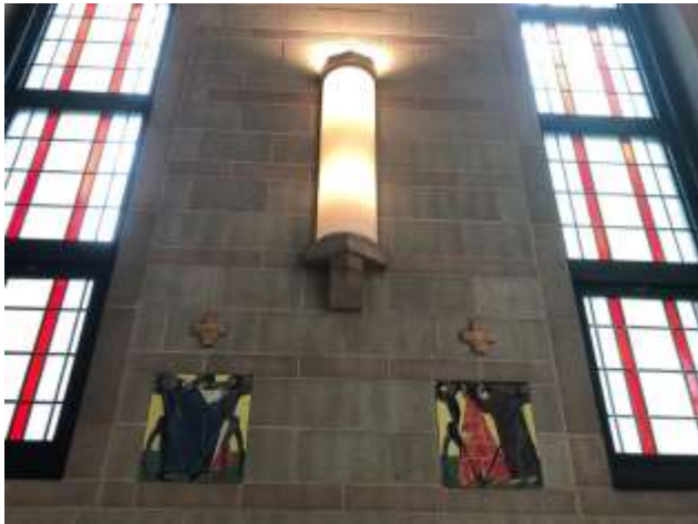
65. Chapel interior, east wall showing the details of the concrete block, two of the Stations of the Cross and the light fitting designed by Cormier (HP, 2020)
