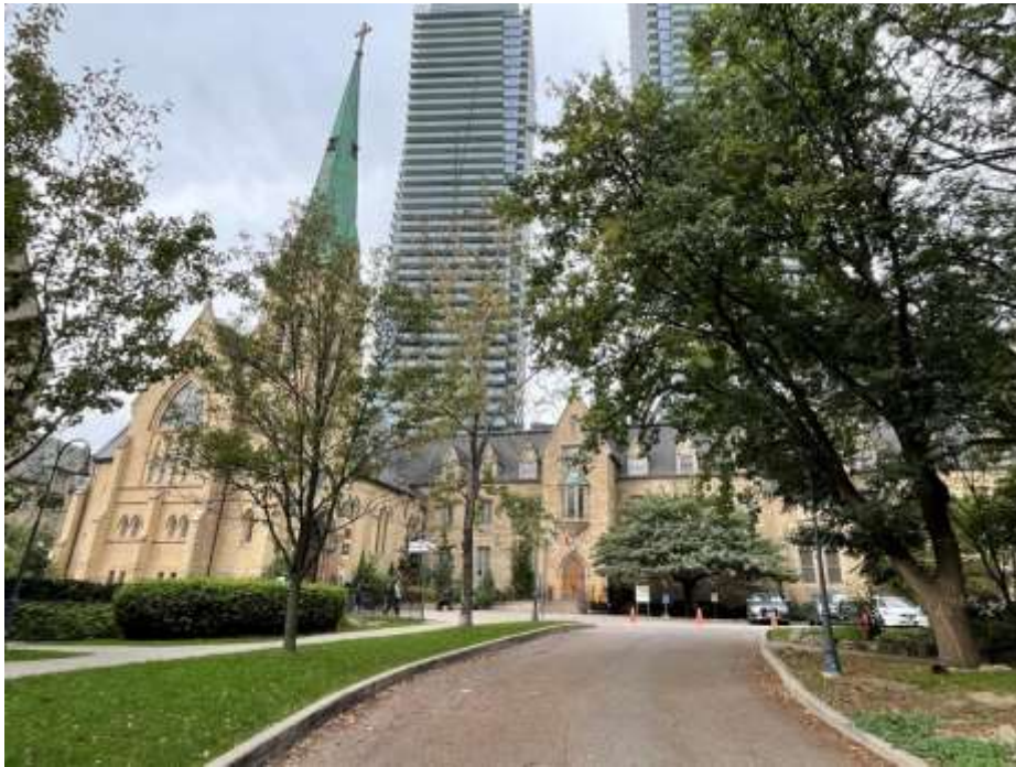
72. View looking north towards the St. Michael's College complex with St. Basil's Church on the left and Odette Hall in the centre. (HP, 2021)
