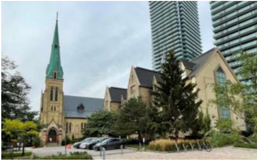
7. View looking west of St. Basil's Church with Odette Hall on the right. The east end wall (far right) after the removal of later extensions (Heritage Planning [HP], 2021)
