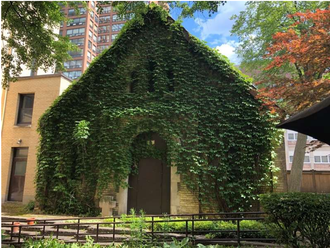
53. Newman Chapel, principal, north elevation facing the west courtyard (HP, 2020)
