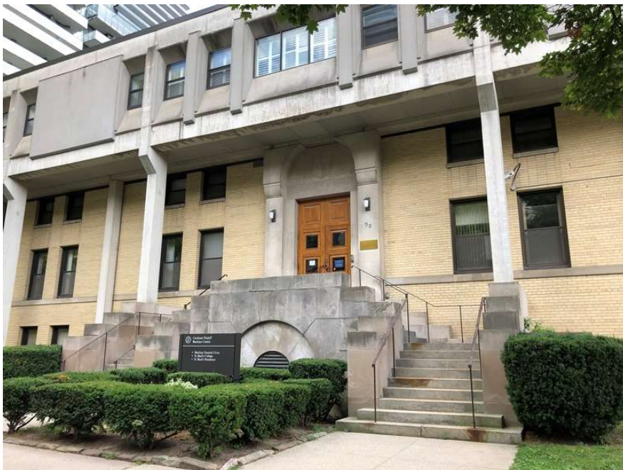
43. St. Basil's Seminary, north elevation, entrance with later addition at the fourth floor level (HP, 2021)
