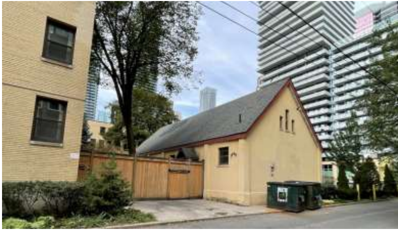
48. View of the south elevations of the west wing of St. Basil's Seminary and Newman Hall Chapel facing St. Basil Lane (HP, 2021)
