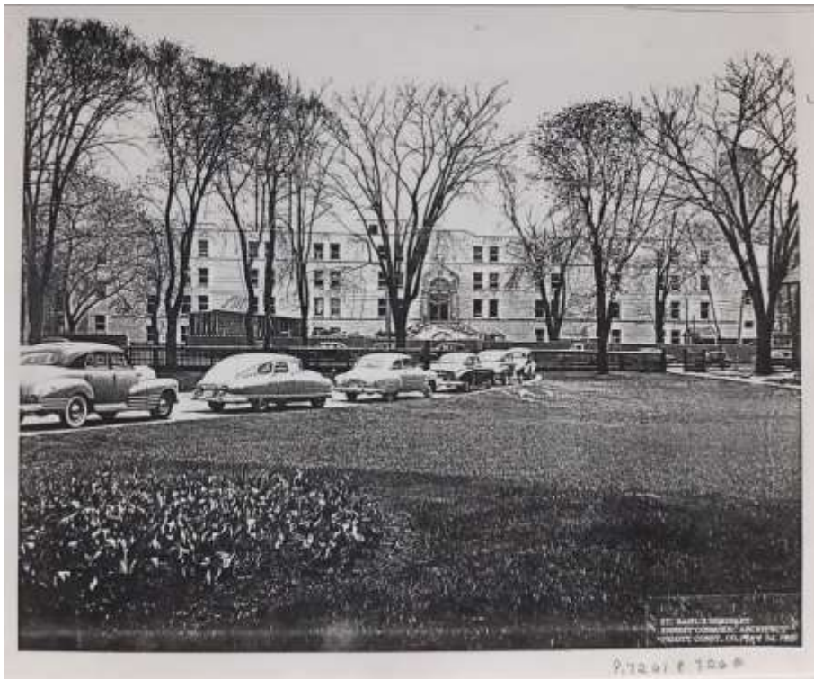
73. View looking south from St. Basil's Church towards St. Basil's Seminary (Ernest Cormier fonds, Pigott Construction Progress Photos, Canadian Centre for Architecture)
