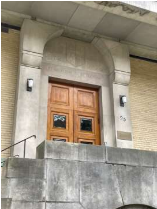
45. Principal Entry on the north elevation (HP, 2020)
