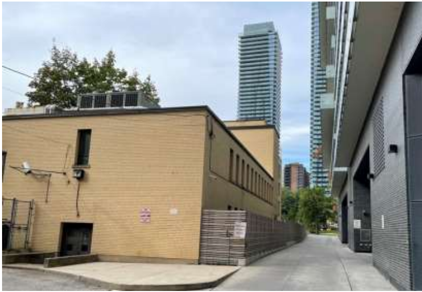
50. View of the south and east elevations of the 1959 east wing of the seminary with a recent condominium tower to the right (HP, 2021)
