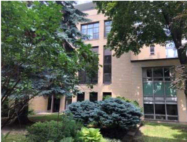
55. View of the east wing, west elevation with the original double-storey library volume shown on the left and the 1959 two-storey addition on the right facing the east courtyard (HP, 2021)
