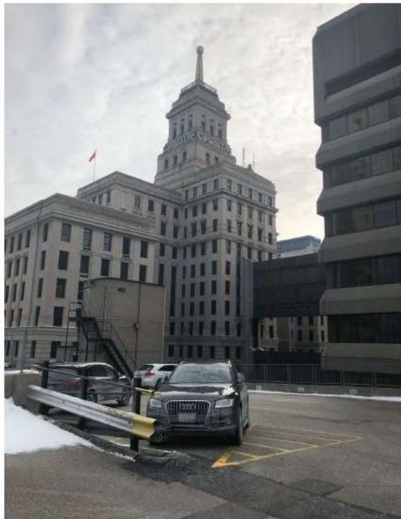
TYPICAL ELEVATION - DISTANT VIEW - EXISTING
