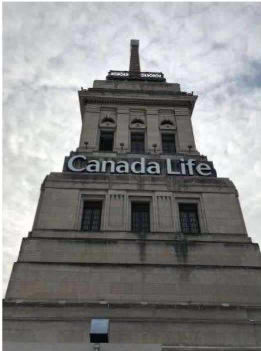
TYPICAL ELEVATION - CLOSE-UP VIEW - EXISTING
