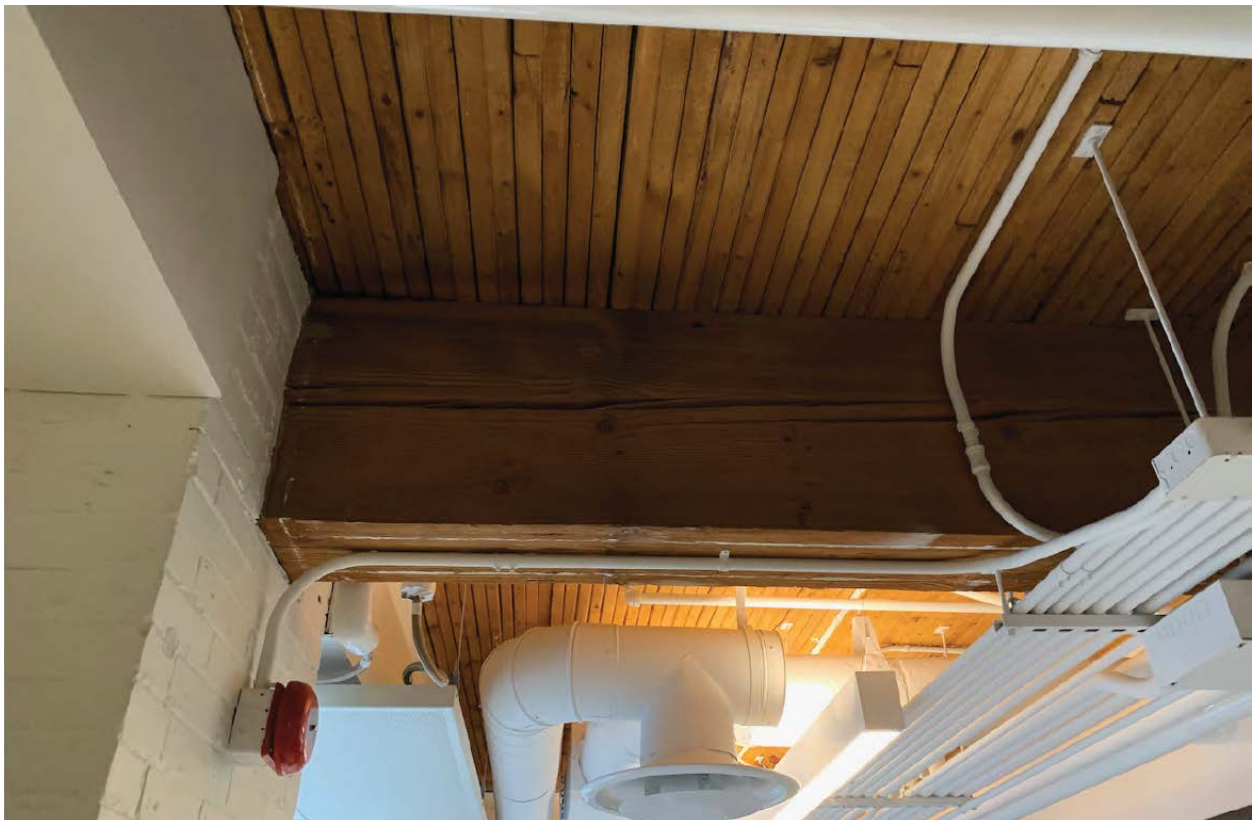
Detailed view of the interior heavy timber post and beam structure of the front (east) portion of 906 Yonge Street (ERA Architects Inc., 2021)
