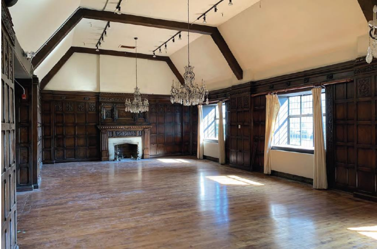
Interior view of 906 Yonge Street's third floor "Oak Room" featuring ornately carved oak wall panelling, an ornately carved wood stone and tile fireplace on the north wall, and a cathedral ceiling featuring wood-clad beams (ERA Architects Inc., 2021)
