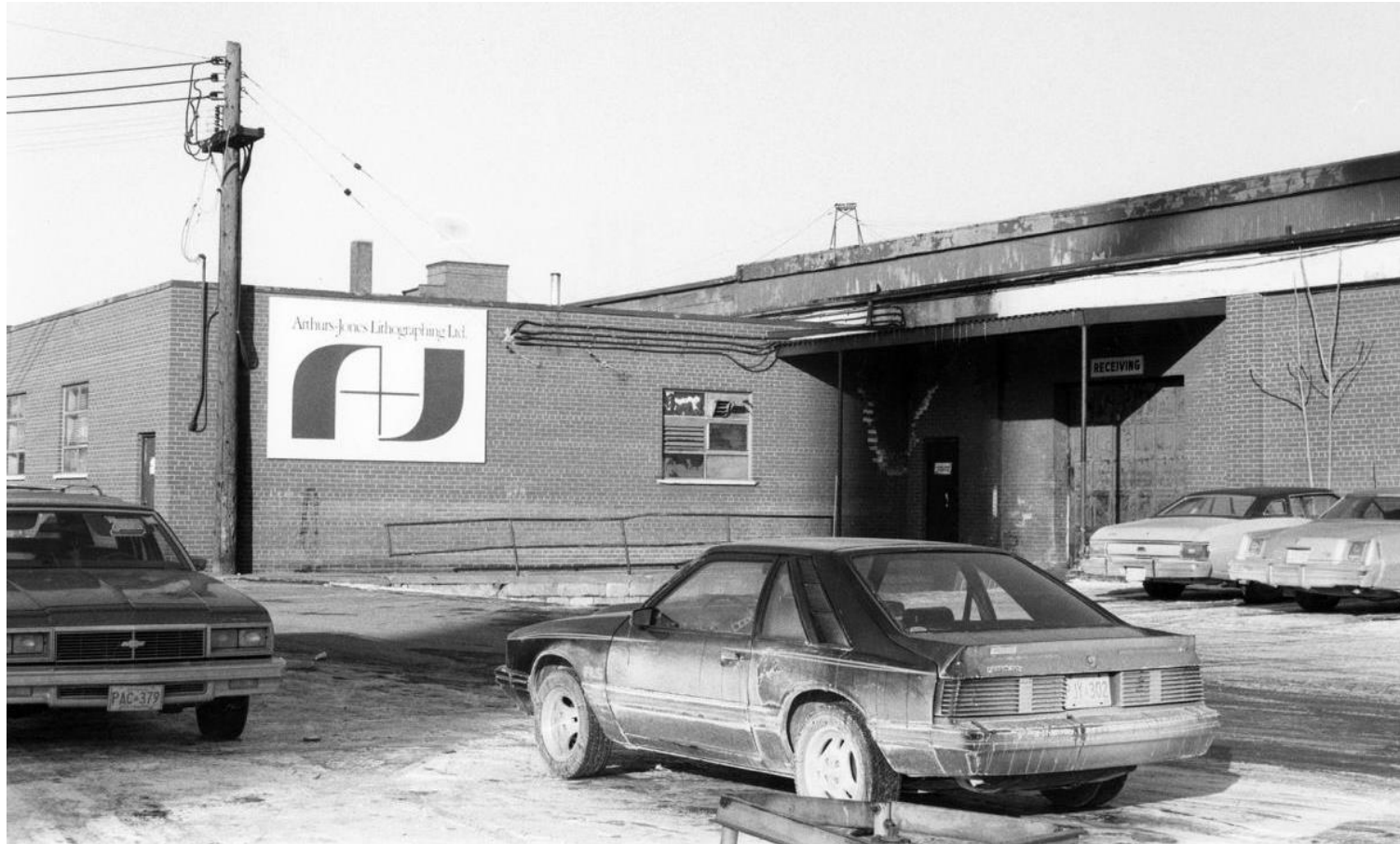
221 Sterling Road; northeastward view of the complex's southwest corner, 1980: "Arthurs-Jones Lithographing Ltd., Sterling Road, south of Merchant Lane, Toronto, Ont."
