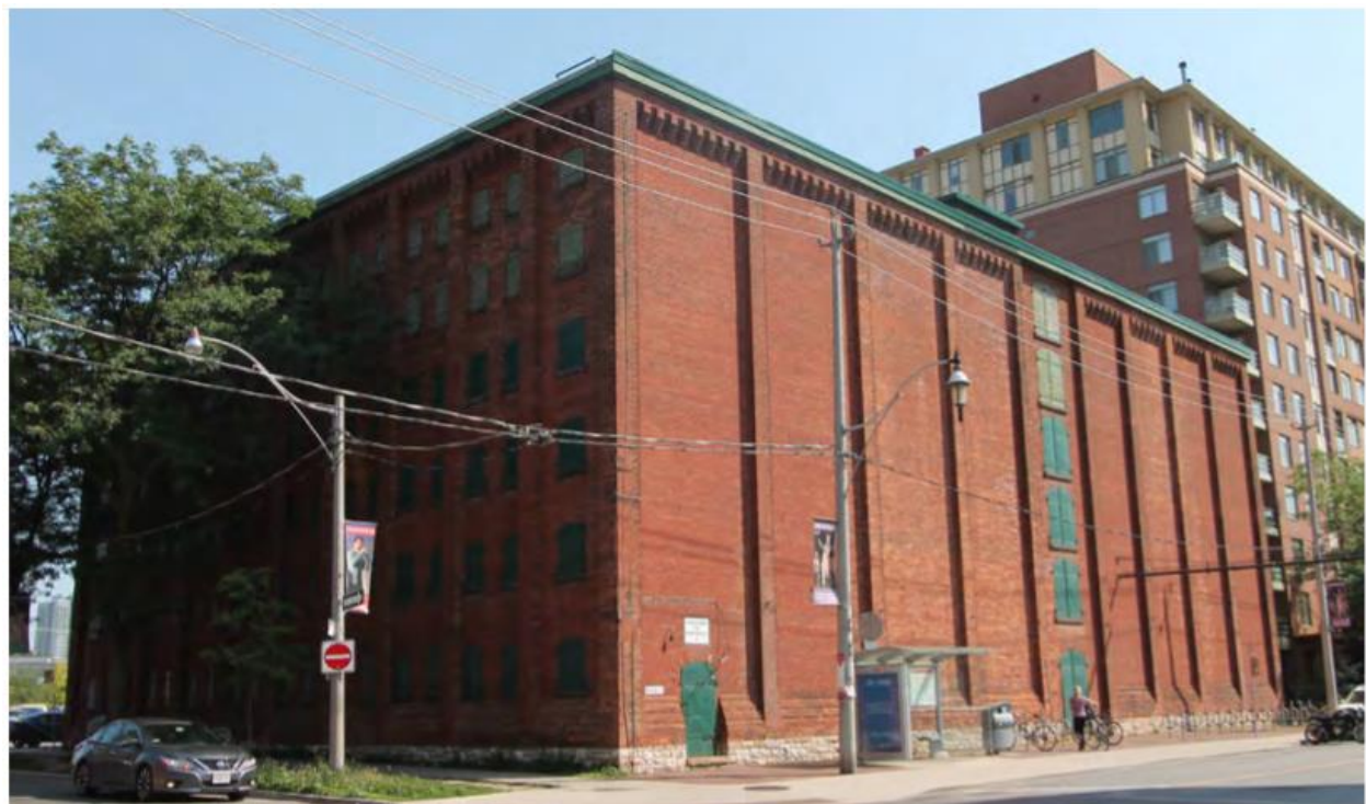
60 Mill Street, west and south elevation of Rack House D. (ERA Architects Inc.)
