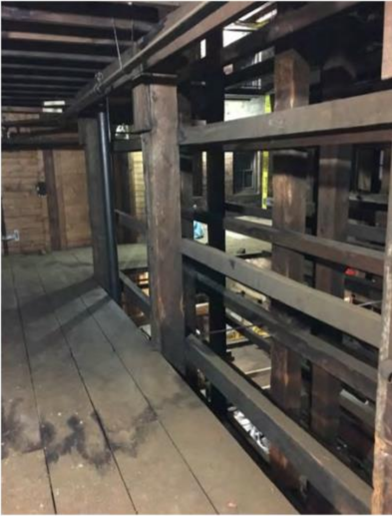
60 Mill Street, interior timber racking structure. (ERA Architects Inc.)
