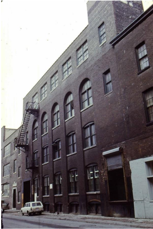
Figure 18. Archival Photographs of 14 Duncan Street in 1973, showing the south elevation on Pearl Street with the 1906 wing and its fourth-floor addition before the alterations to the building (Toronto Historical Board)
