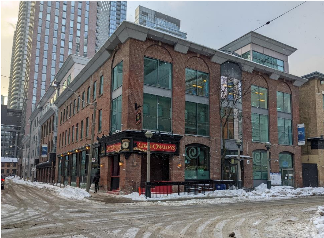
Figure 22. View of the southeast corner of 14 Duncan Street (Heritage Planning, 2022)
