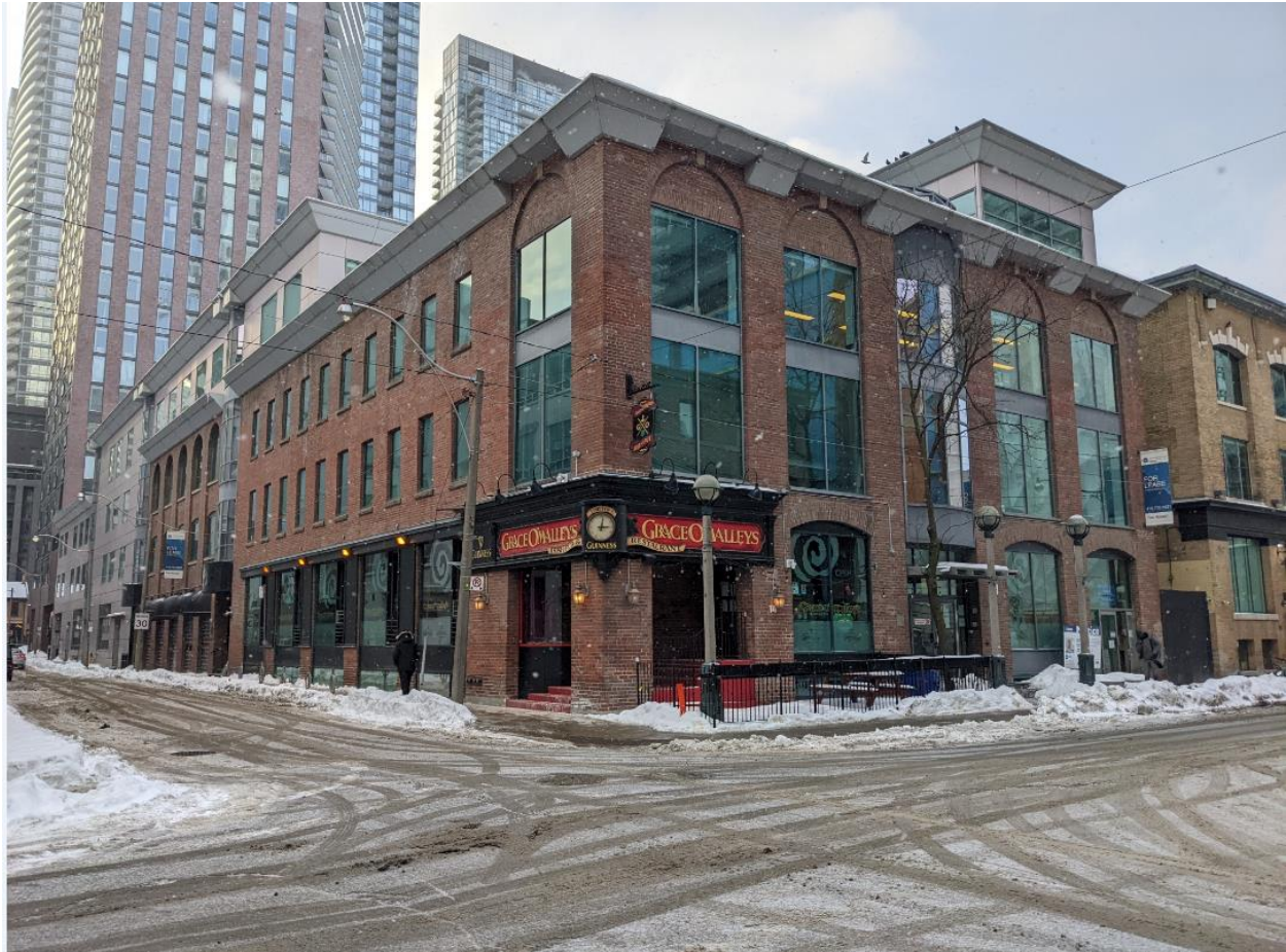
Northwest corner of Duncan and Pearl streets showing the Telfer Paper Box Building (Heritage Planning, 2022)
