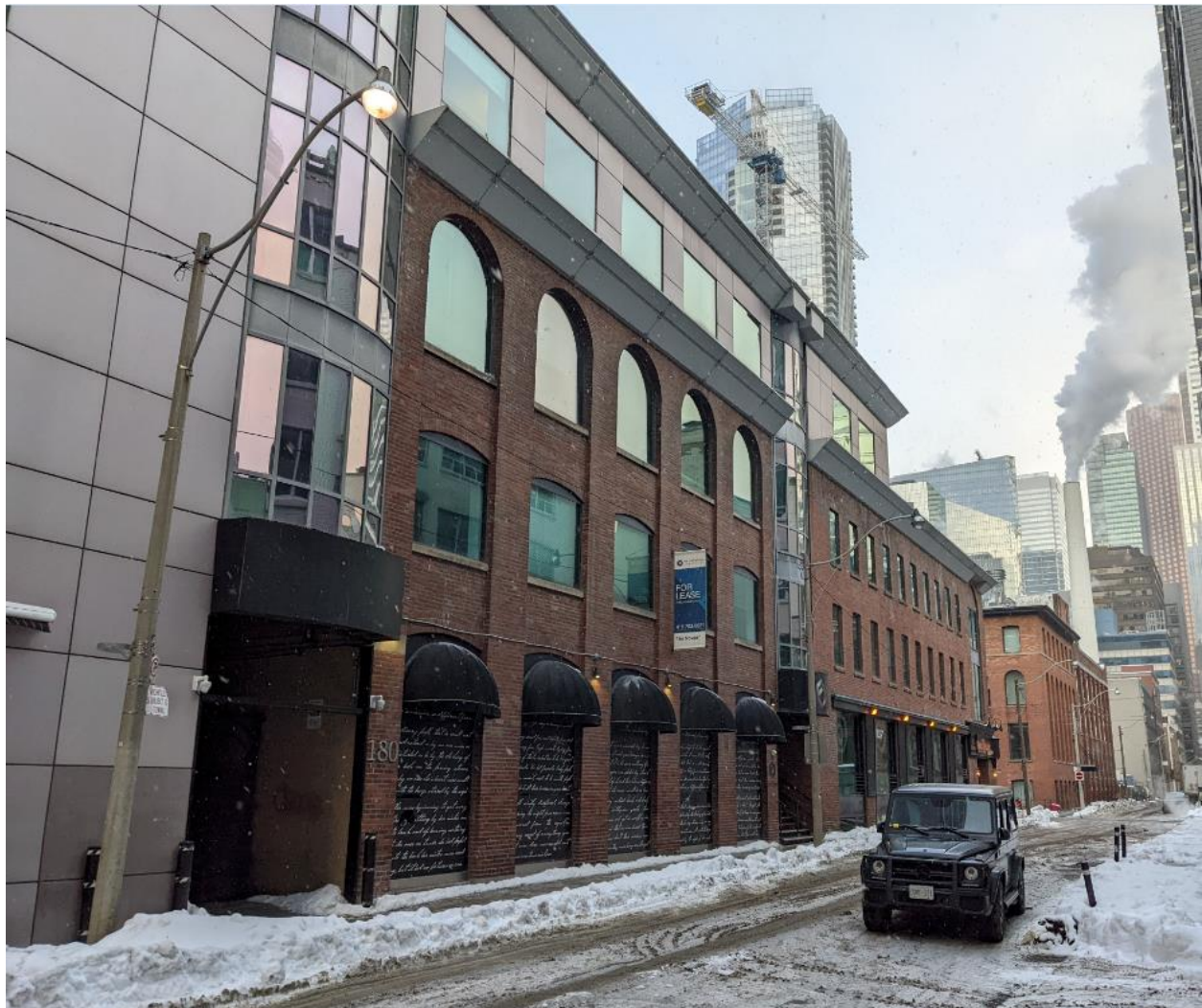
Figure 27. Detail of the side (south) elevation, illustrating the 1902 building (right) and the 1906 addition (left) with the fourth-storey addition that was reclad in the late-20 th century (Heritage Planning, 2022)
