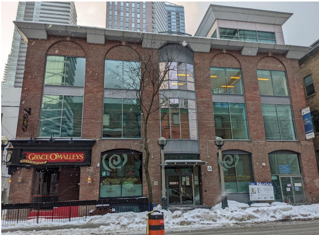
Figure 23. View of the principal (east) elevation of 14 Duncan Street (Heritage Planning, 2022)
