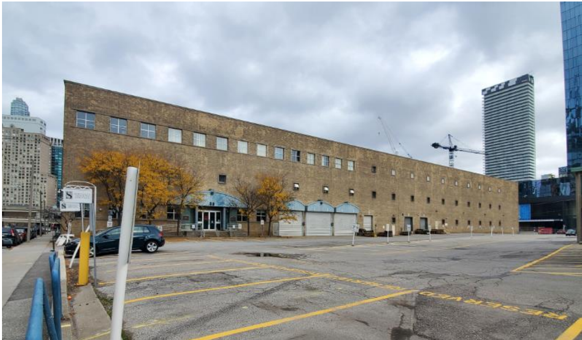
8. Detail of the south elevation of the warehouse fronting Queen's Quay East (Heritage Planning, 2020)
