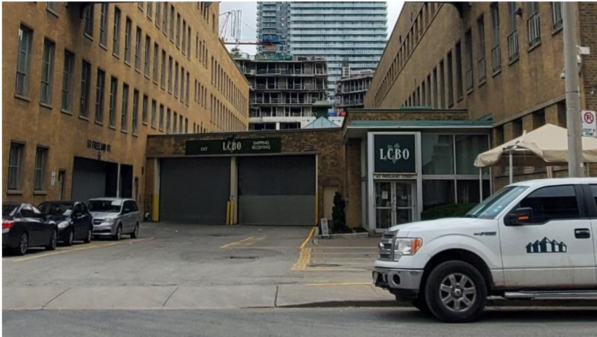
7. Detail of the side (west) entrance to the warehouse and the rolling garages in the one-storey connecting building (Heritage Planning, 2020)
