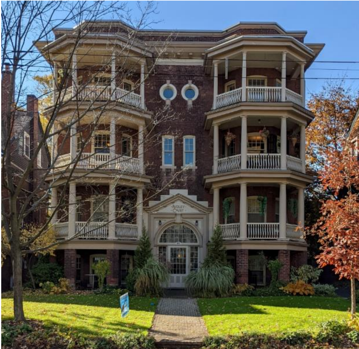
East (principal) elevation of 68 Kendal Avenue (Heritage Planning, 2021)
