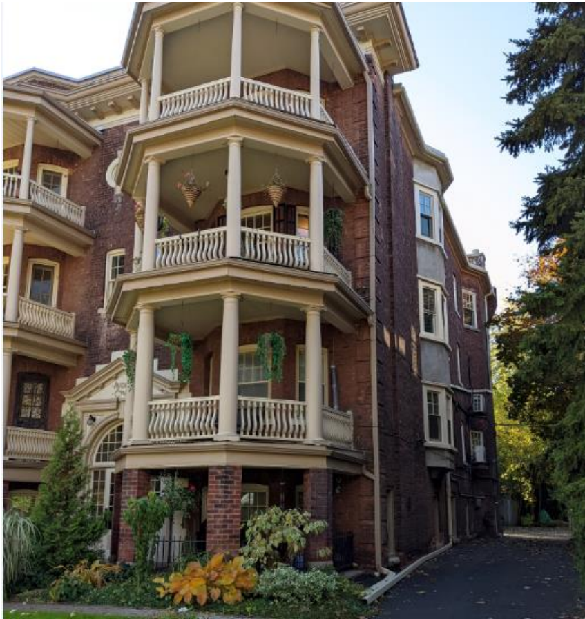
23. Current photograph looking west, showing the north and east elevations of the building at 68 Kendal Avenue (Heritage Planning, 2021).
