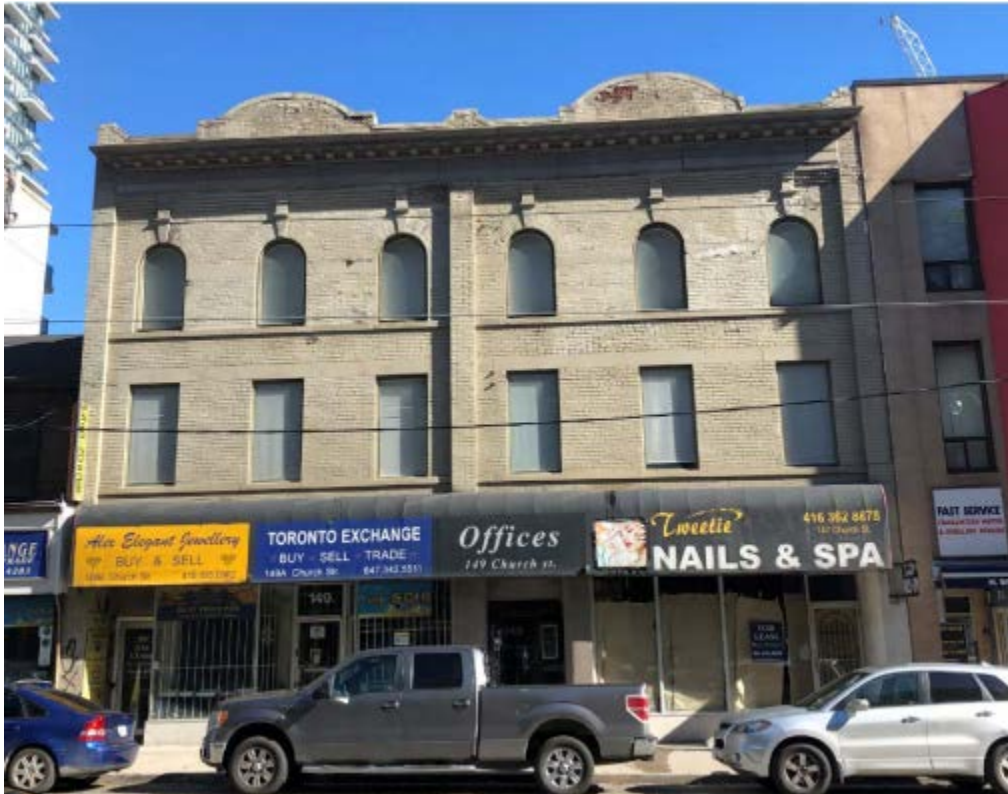
Current photograph looking east, showing the principal (west) elevation of the building at 147 Church Street. (Heritage Planning, 2021)
