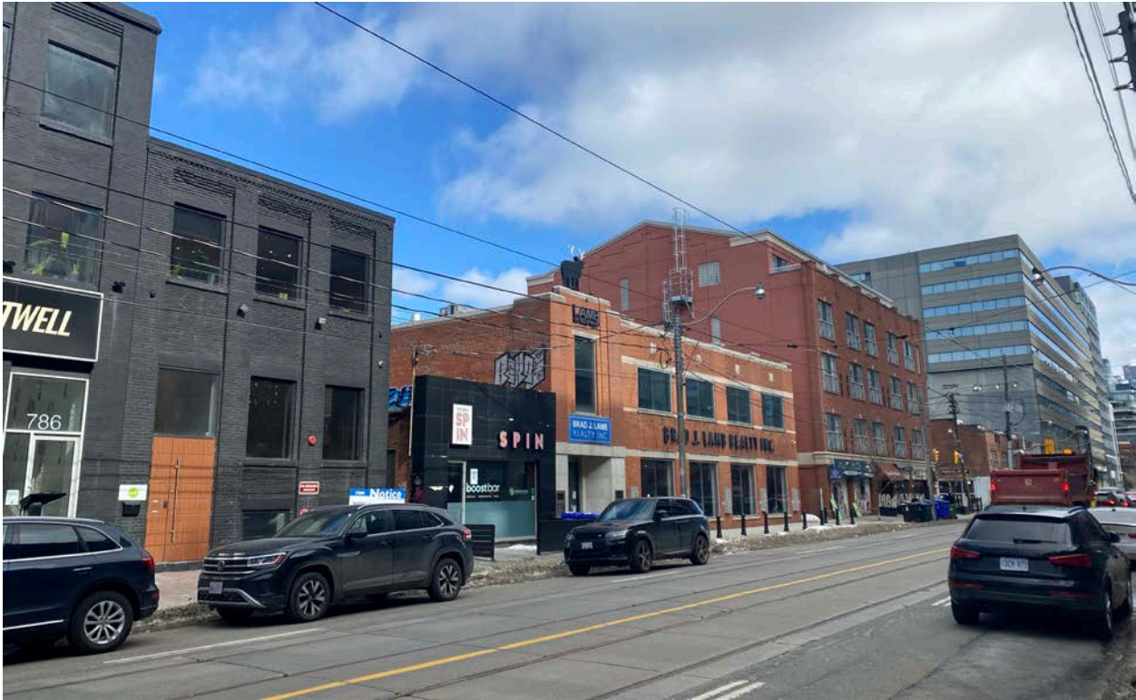
Figure 22: Northeastward view of 778 King Street West (Heritage Planning, 2022).
