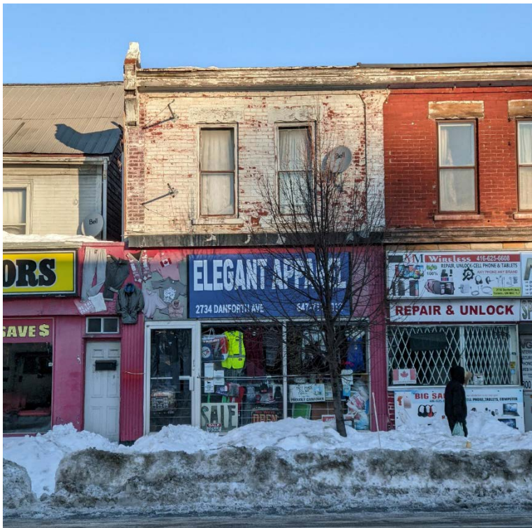
22. Principal (south) elevation of 2734 Danforth Avenue. (Heritage Planning, 2022)
