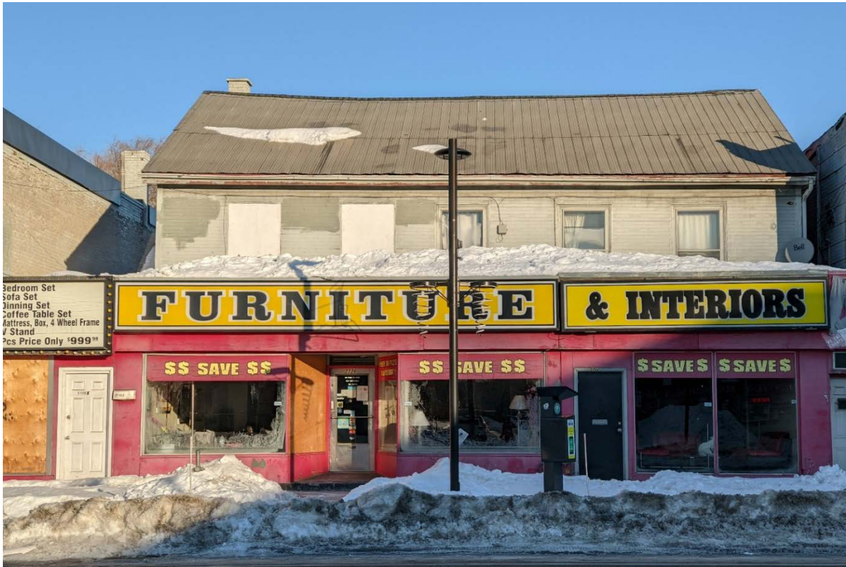
10. Principal (south) elevation of 2726 Danforth Avenue with its early 20th century projecting storefront addition at street level. (Heritage Planning, 2022)
