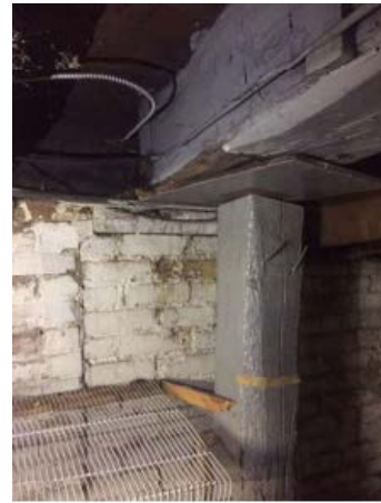
14, 15 and 16. Photos showing the massive timber support beams in the unfinished basement with their hand-hewn markings. (ERA, 2019)
