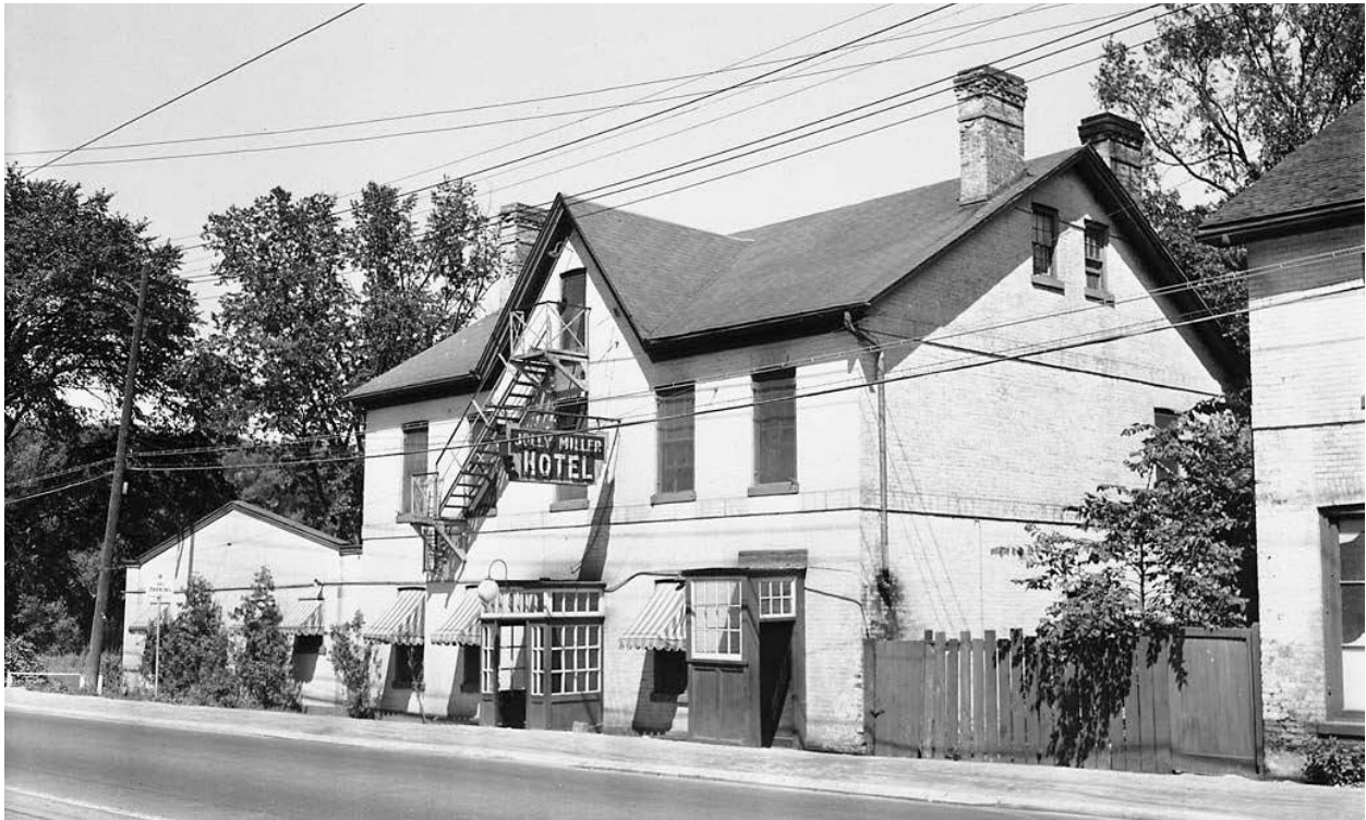
8. The Miller Tavern built c. 1857. The 2-storey building is organized into five bays like the property at 2726 Danforth Avenue, the only difference being a small centred gable above the main entrance at The Miller Tavern (formerly The Jolly Miller Hotel). (South Armour Heights Residents Association)
