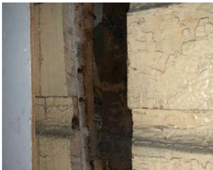
17 and 18. Photos showing the exterior sheathing of the original building including lath and plaster protected by tongue-and-groove wooden siding. At right, the north elevation of the tail is currently over-clad with vinyl siding. (ERA, 2019)
