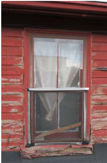
12 and 13. Photos showing the wooden frame windows on the north elevation with their two-over-two panes and brick chimney. (ERA, 2019)
