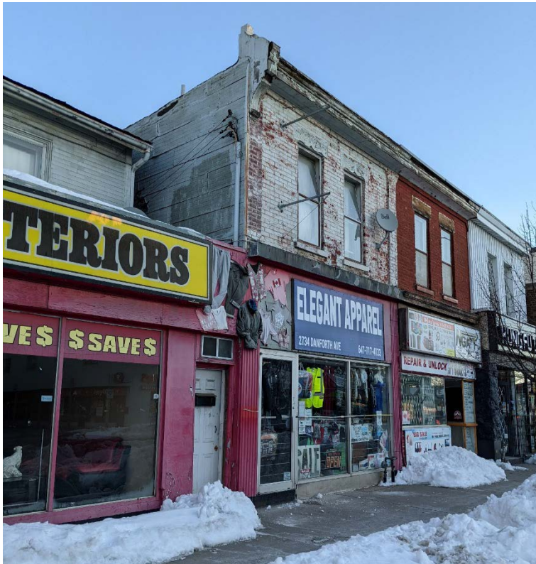
21. Current photo of 2734 Danforth Avenue showing the wooden cornice and decorative corner bracket. Also visible are the two adjacent properties at 2736 and 2740, which were built together with the subject property in c.1886 (Heritage Planning, 2022)
