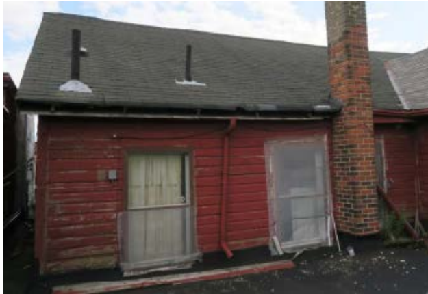
12 and 13. Photos showing the wooden frame windows on the north elevation with their two-over-two panes and brick chimney. (ERA, 2019)
